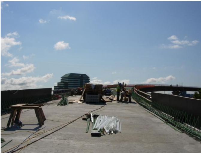
FIGURE 5. Concrete deck for 'Flyover' (Bridge No. 169) on Project No. 92-619.
