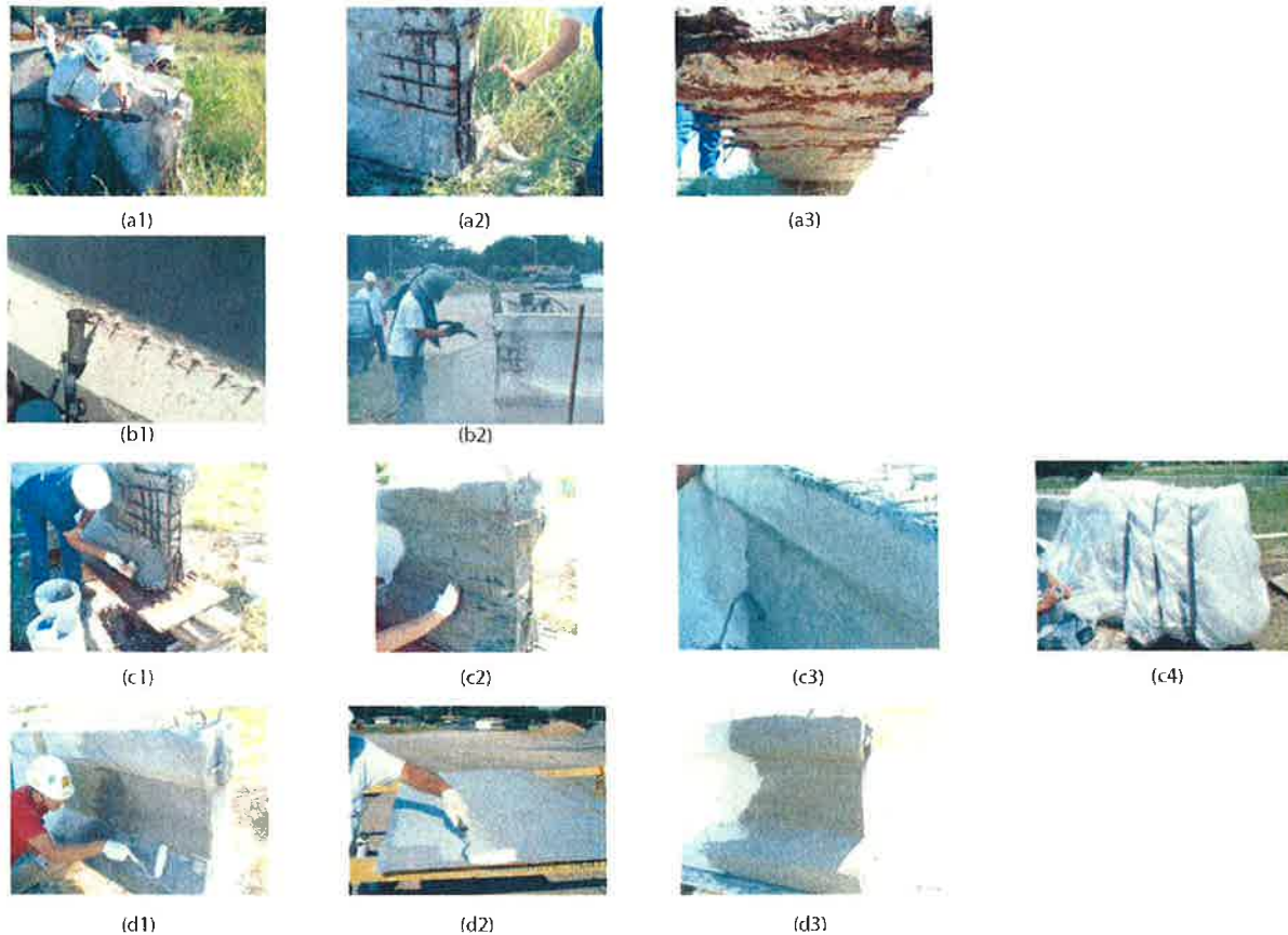
Figure 7: Retrofitting process documented by Mr. Christopher Davis: (a1) using a pneumatic drill to remove unsound concrete; (a2) using a standard hammer to remove unsound concrete so that more damage was not done; (a3) original view of damage to the bottom of the girder; (b1) sandblasting the surface; (b2) using a pressure injection epoxy to repair existing cracks; (c1) applying the initial coat of the wet mortar; (c2) applying the second coat of the intermediate mortar; (c3) the final mortar being the thickest and the repaired end finally shaped; (c4) the burlap sack that was used during curing; (d1) rolling on the epoxy to the girder prior to install the FRP wrap; (d2) impregnating the three-layer FRP wrap prior to installing it, and (d3) rolling the FRP wrap onto the girder to avoid air voids in the finished product.
