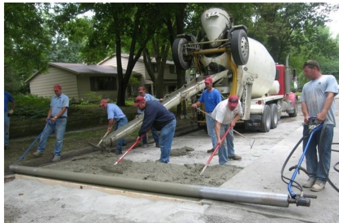
Figure 6–24. Roller screed for leveling of poured concrete
