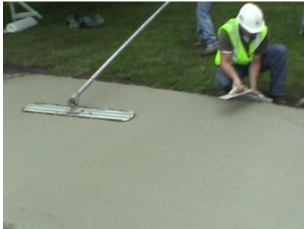
Figure 6–16. Finishing of pavement, South 4th Street
