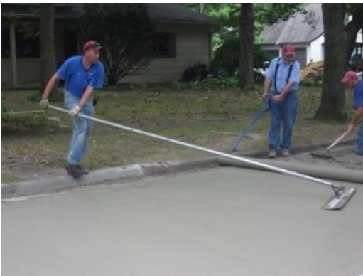
Figure 6-29. Finishing of pavement, North Riverside Drive
