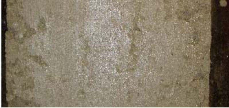
Figure 4–29. Plan view of MCM1-10 pavement from the mini-paver
