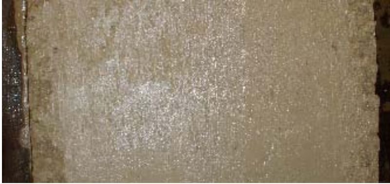
Figure 4–32. Plan view of MCM1-05 pavement from the mini-paver
