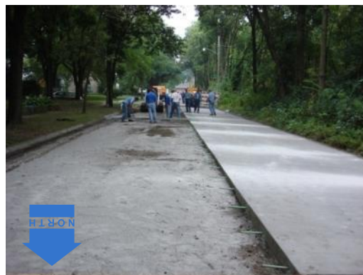
Figure 6–23. Slab made from conventional concrete mixture (right) and SCC base (left)
