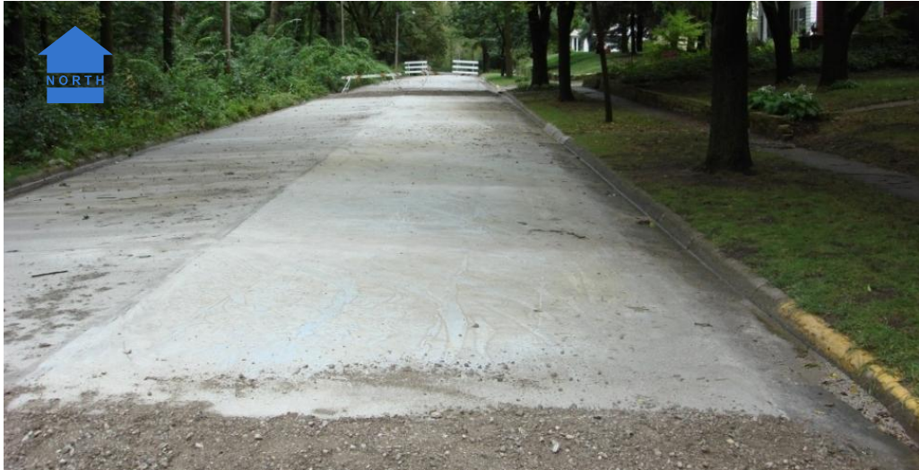
Figure 6-41. SFSCC slab after 3 days of curing, North Riverside Drive
