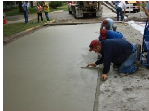
Figure 6-29. Finishing of pavement, North Riverside Drive
