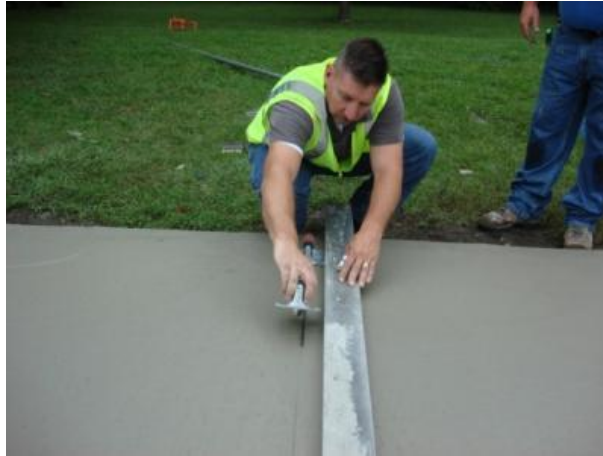
Figure 6–17. Cutting of joint, South 4th Street
