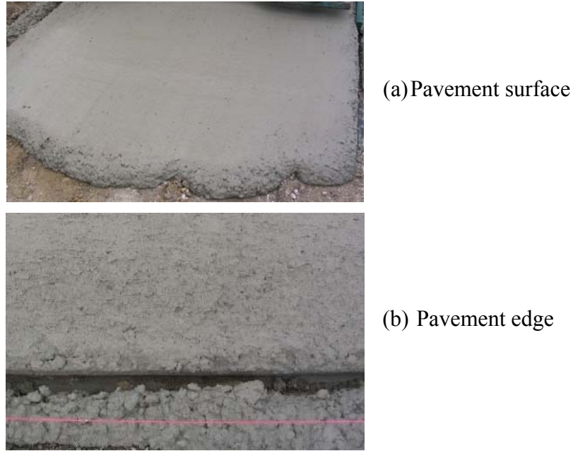
Figure 6–3. SFSCC pavement of the first field trial
