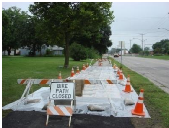
Figure 6–19. Curing of concrete, South 4th Street
