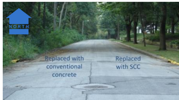
Figure 6–22. Asphalt pavement that was replaced
