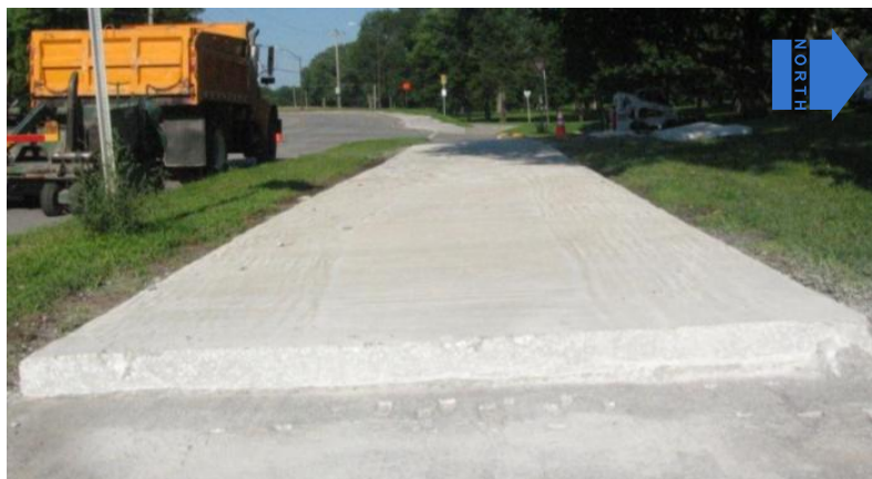
Figure 6–34. SFSCC bike path after 7 days of curing, South 4th Street
