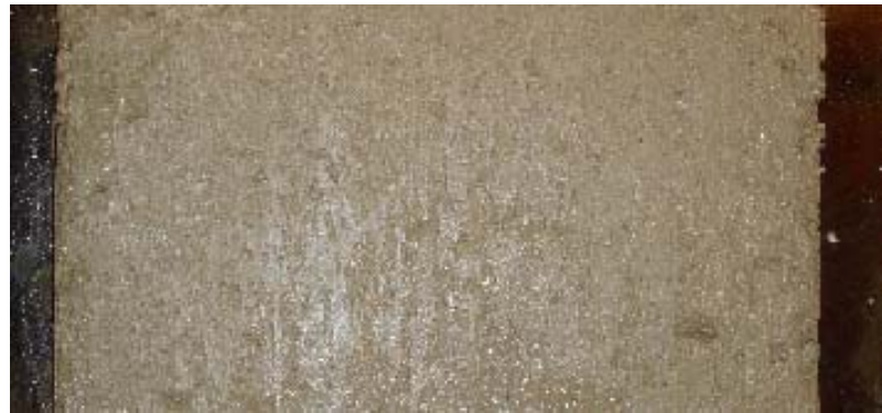
Figure 4–31. Plan view of MCM3-10 pavement from the mini-paver
