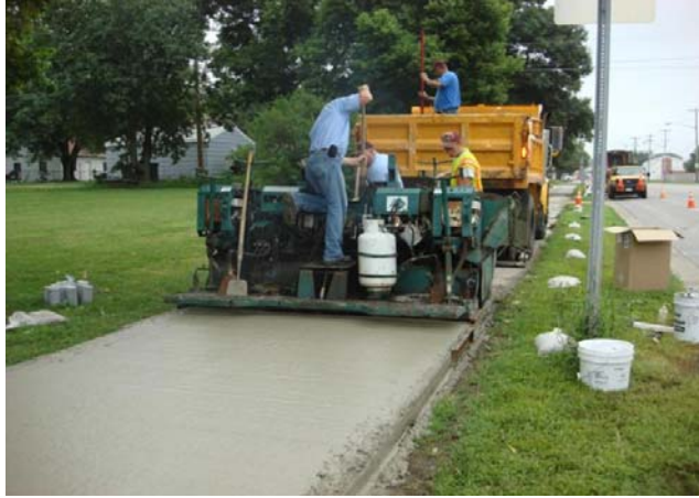
Figure 6–15. S4TH-M2 slab before finishing
