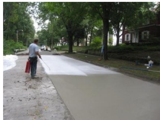
Figure 6-31. Application of curing compound, North Riverside Drive
