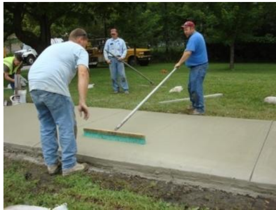
Figure 6–18. Brooming for surface texture, South 4th Street
