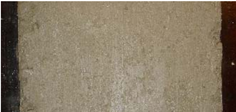
Figure 4–30. Plan view of MCM2-10 pavement from the mini-paver
