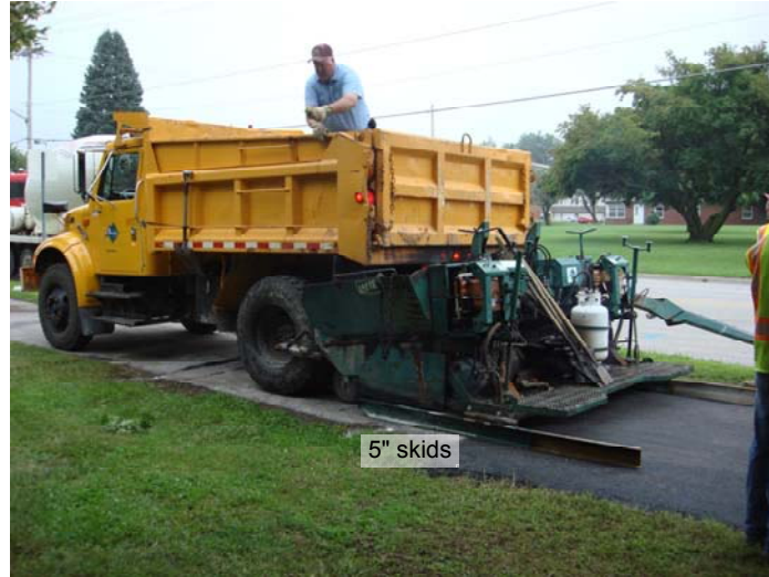
Figure 6–9. Modified asphalt paver for slip-form paving
