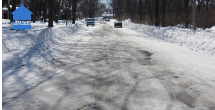
Tracks on snow show vehicle path/loading (taken on February 2010)
