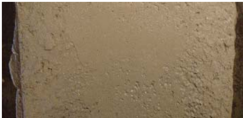
Figure 4–28. Plan view of MCM pavement from the mini-paver
