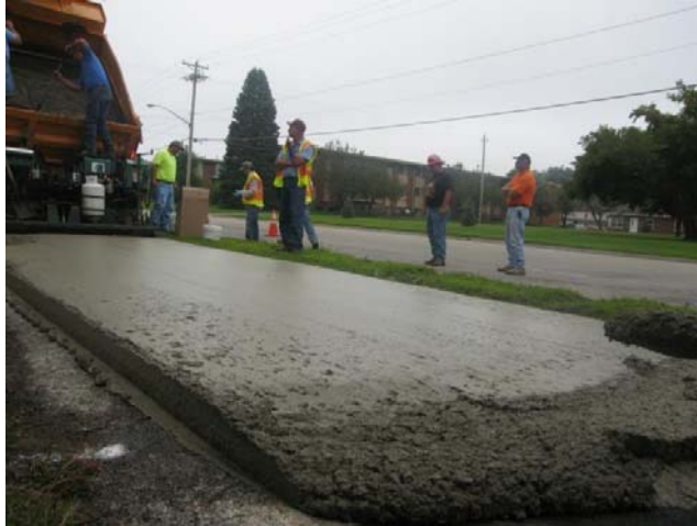
Figure 6–13. S4TH-M1 slab before finishing
