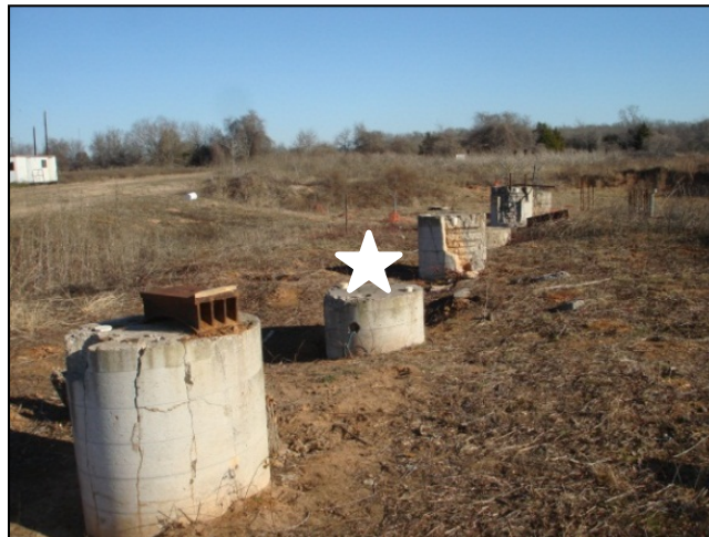
Figure 12-21. Five Straight Shaft Foundations at the NGES.
