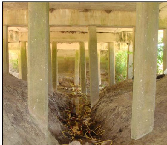
Figure 12-33. Field Setup for Bridge 17-094-0315-02-019.
