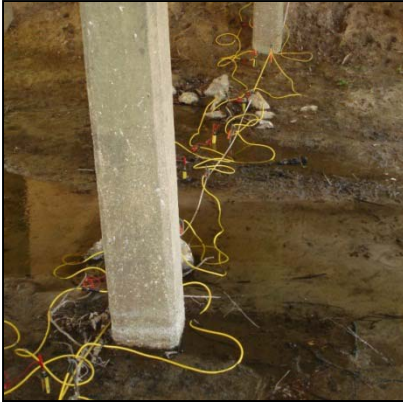
Figure 12-34. Two Piles Tested through Water.
