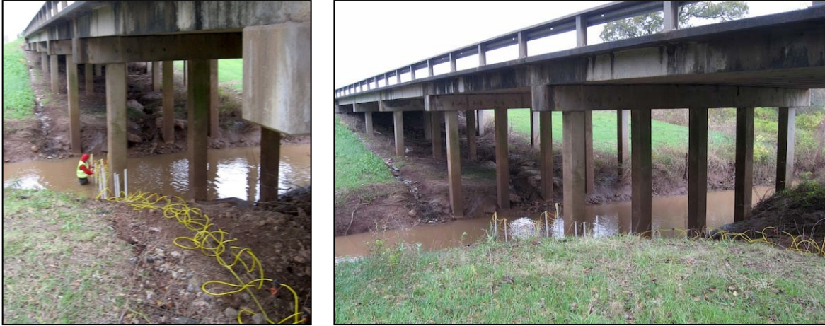
Figure 11-6. Bridge 14 ERI Fieldwork.
