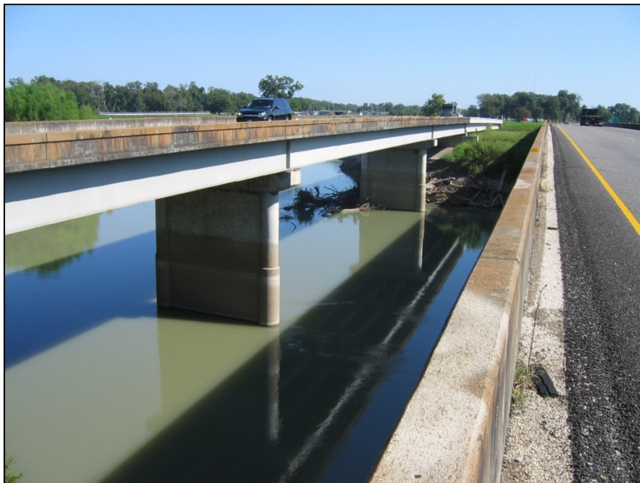
Figure 9-9. US 59 over the Guadalupe River.
