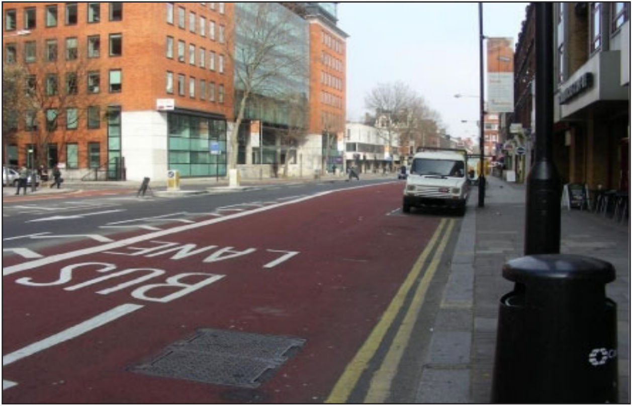
Figure 3. Additional-width Bus Lane to Allow for Parking (London)
