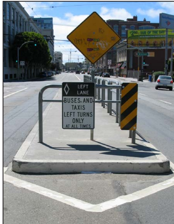
Figure 26. Left-Curbside Lane with Island (San Francisco)
