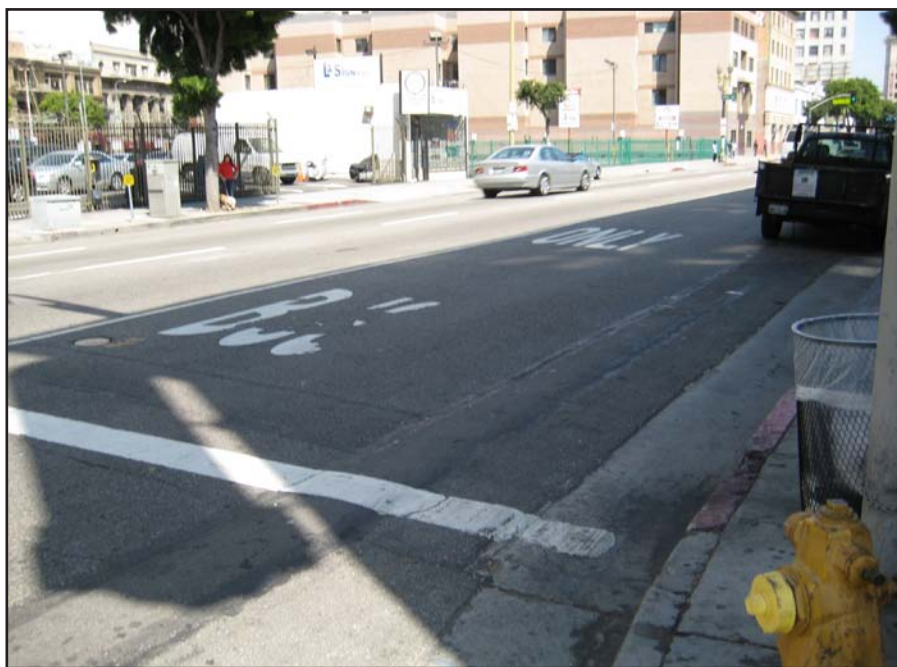
Figure 10. “Bus Only” Text Painted on the Pavement of a Bus Lane (Los Angeles)
