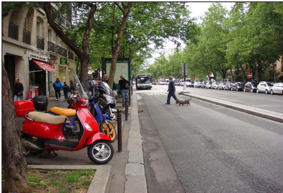
Figure 17. Bus Lane with a Raised Curb Separating It from the Regular Traffic Lane (Paris)
