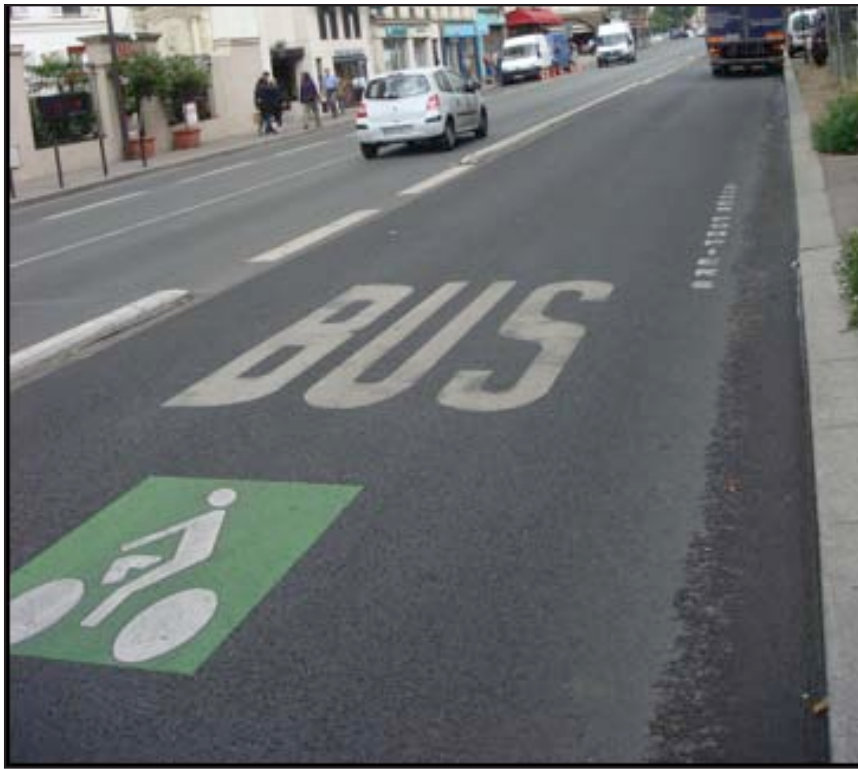
Figure 19. Pavement Markings Indicating a Bus Lane that Permits Cyclists (Paris)
