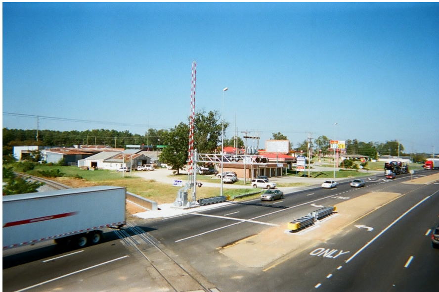
Figure 3-3. Northbound lanes after installation
