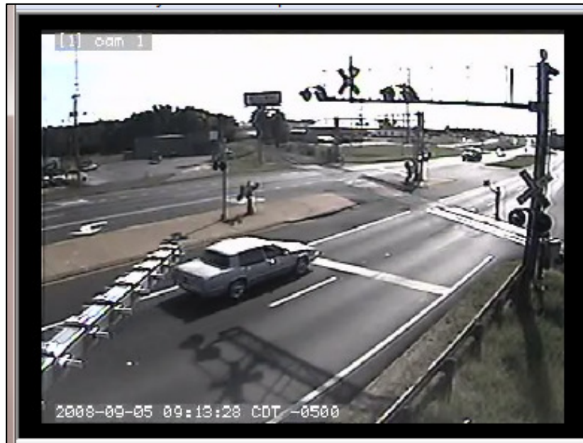
Figure 3-1. The crossing before gate installation
