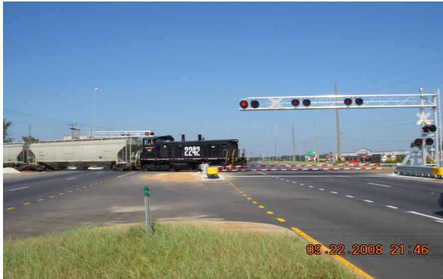
Figure 3-4. Southbound lanes after installation
