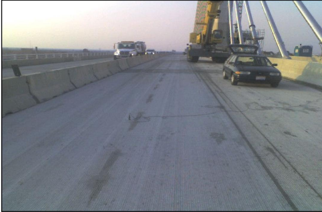
Figure 15.2 Typical accelerometer set up for the VGCS Bridge OMA test (Chauhan, 2008)
