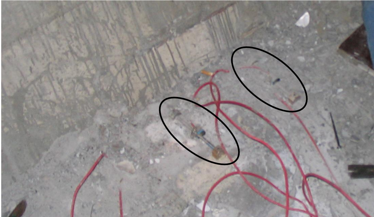
Figure 6.3. Vibrating Wire Strain Gages in Segment 28SB25, Partially Embedded (Bosworth 2007, Fig. 2.8)
