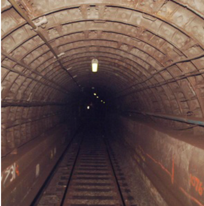
Figure 10. A PATH Tunnel Under the Hudson River
