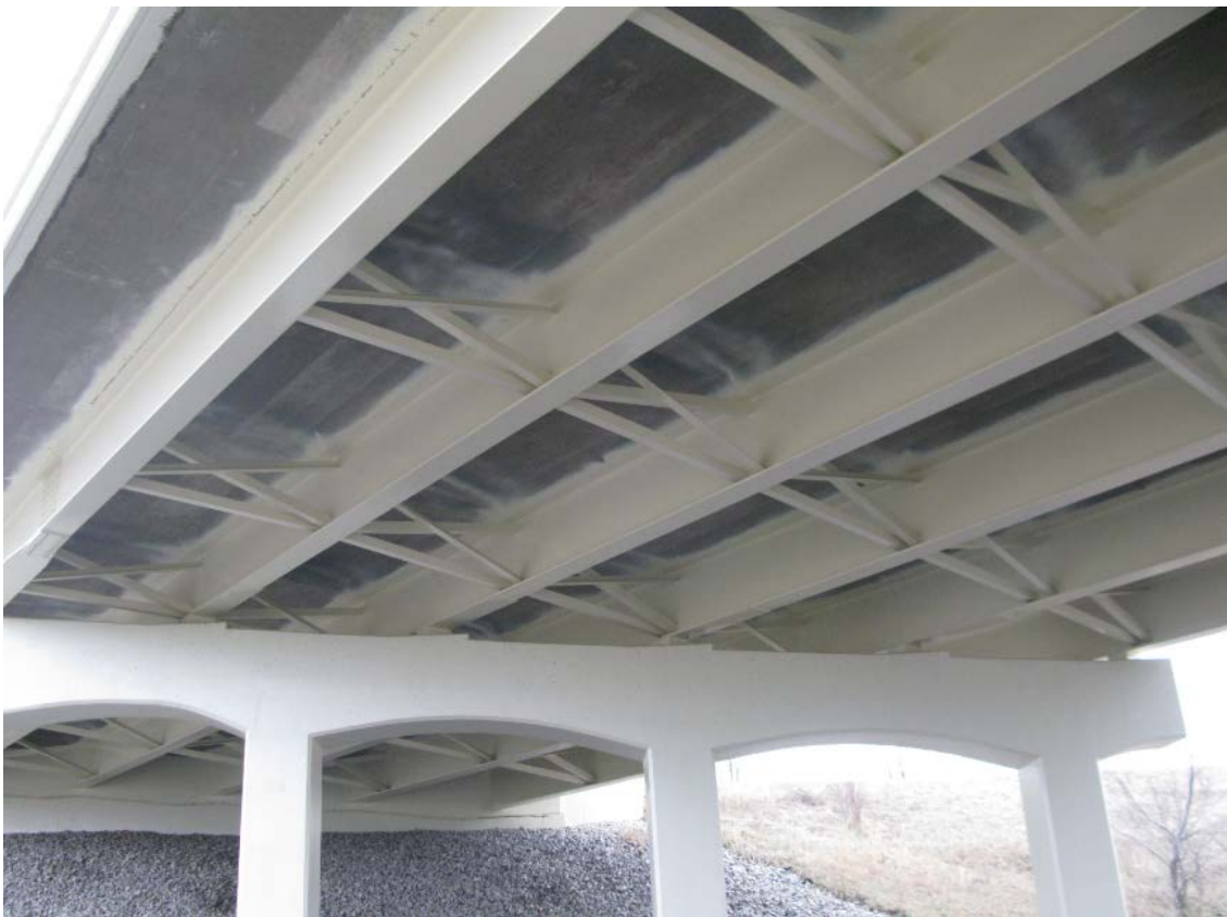
Figure 6 Stringer Supported Bridge
