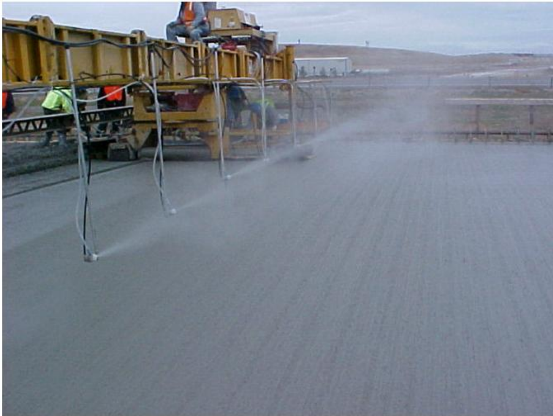
Figure 4 Fogging of Fresh Concrete (Patnaik, et al., 2010)
