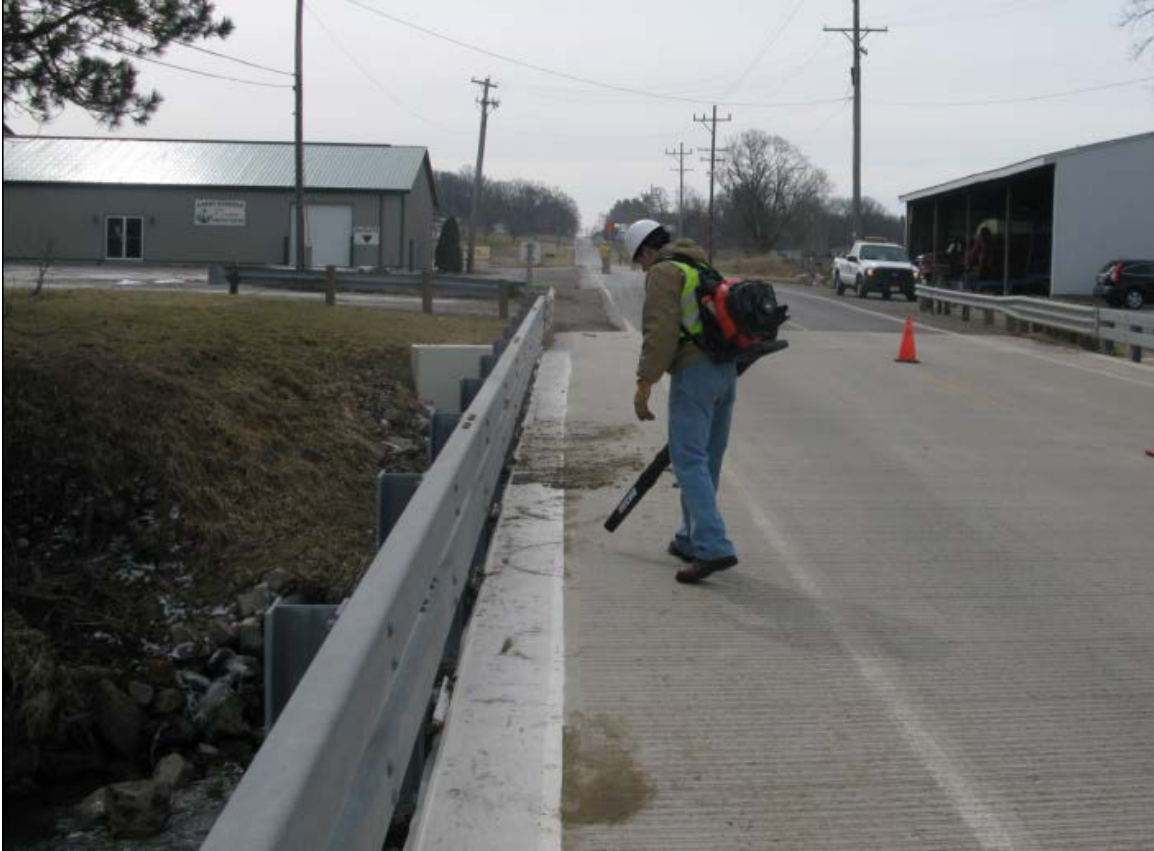
Figure 9 Clearing Bridge Deck of Debris
