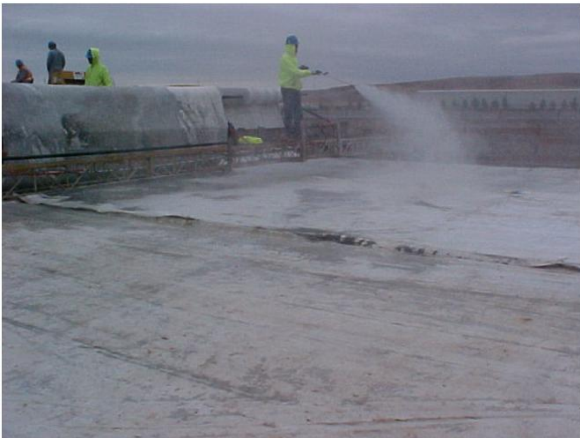
Figure 3 Curing Blankets on Fresh Concrete (Patnaik, et al., 2010)
