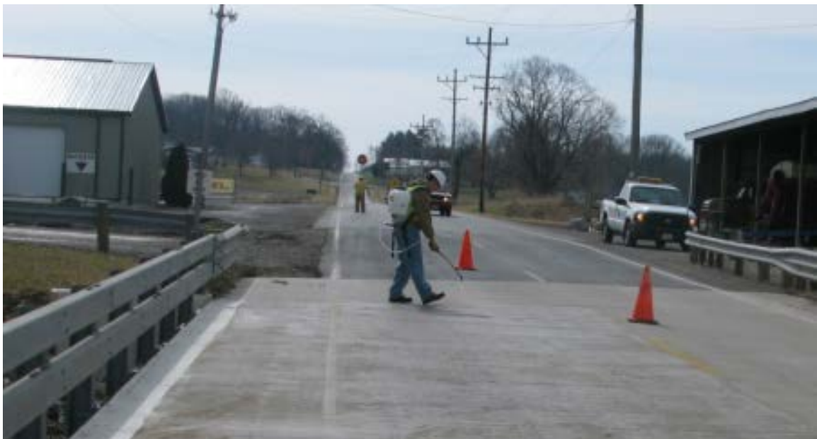
Figure 10 Spraying Water on Bridge Deck
