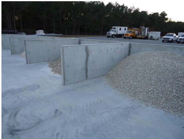
Figure 3-3. Storage bins for aggregates.
