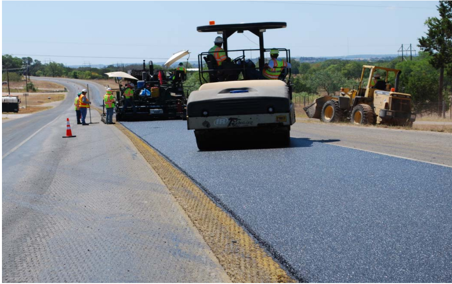
Figure 5-17. Placement of the CMHB-F on US 87.
