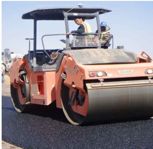
Figure 5-14. Compaction of the SMA.
