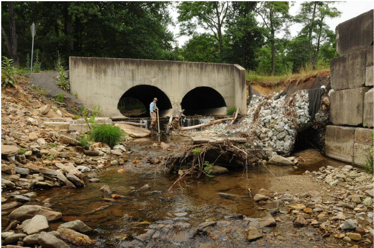
Photo 4.1. LTBD measured at the culvert outlet of Site 45.
