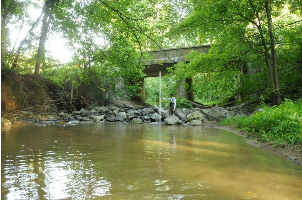
Photo 4.2. LTBD measured downstream of bridge at Site 50.
