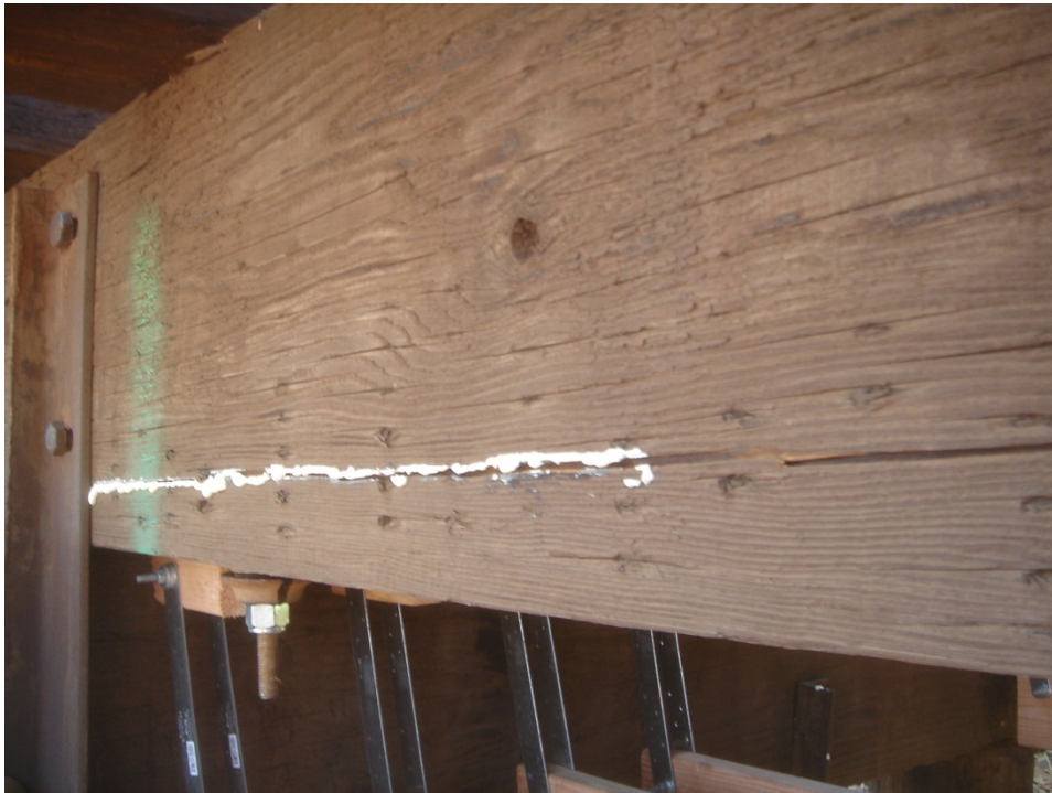
Figure C.38 Spray foam used to fill cracks
