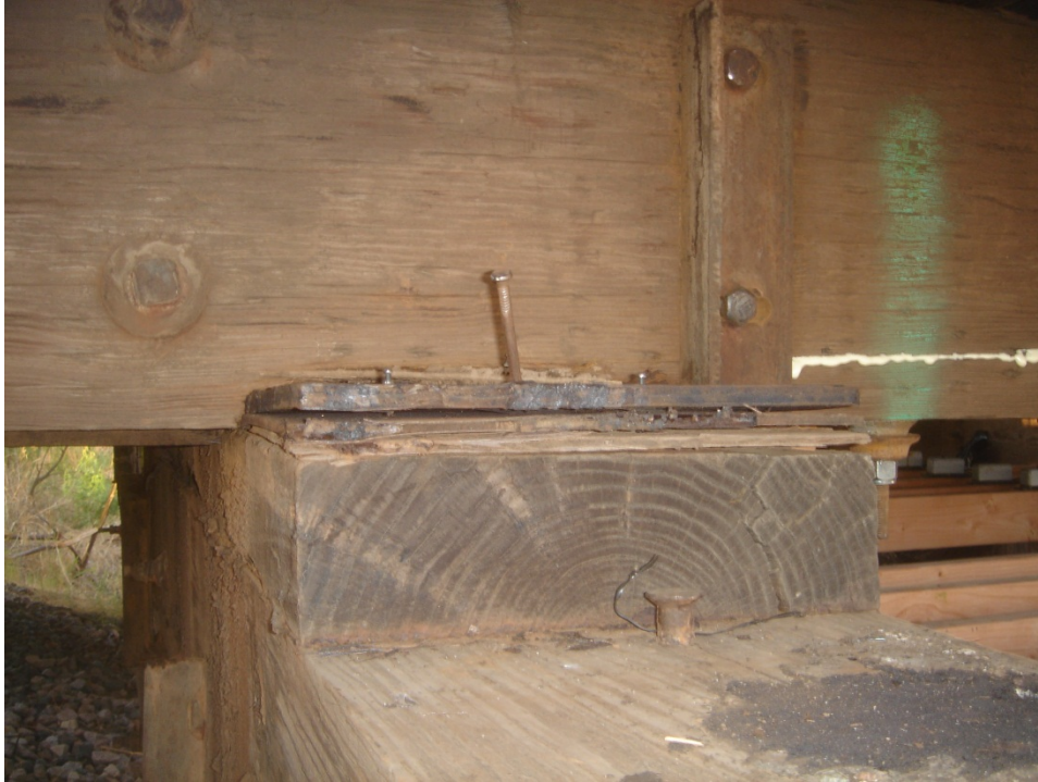
Figure C.35 Stringer 8 - Shim added below end of Span 1, Span 2
