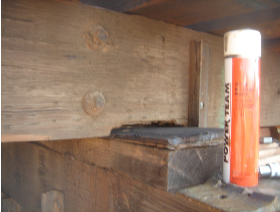
Figure C.33 Stringer 8 - Shim added below end of Span 1, Span 2
