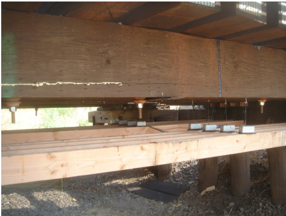
Figure C.28 Alternate view of Instrumentation Setup – Bridge No. 2
