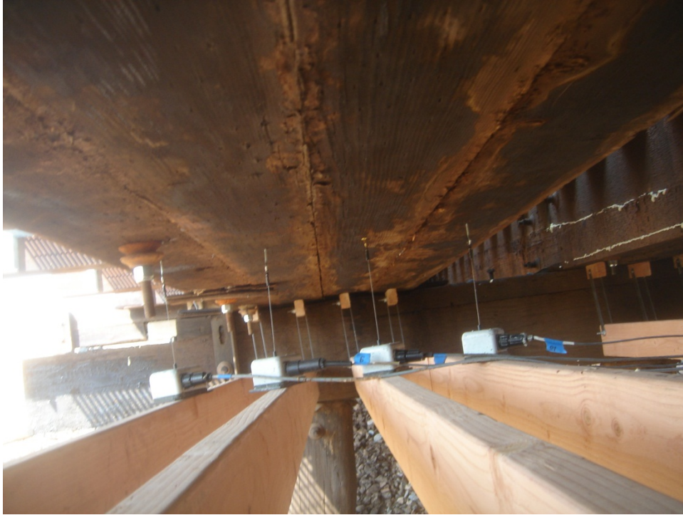
Figure C.29 Alternate view of Instrumentation Setup – Bridge No. 2
