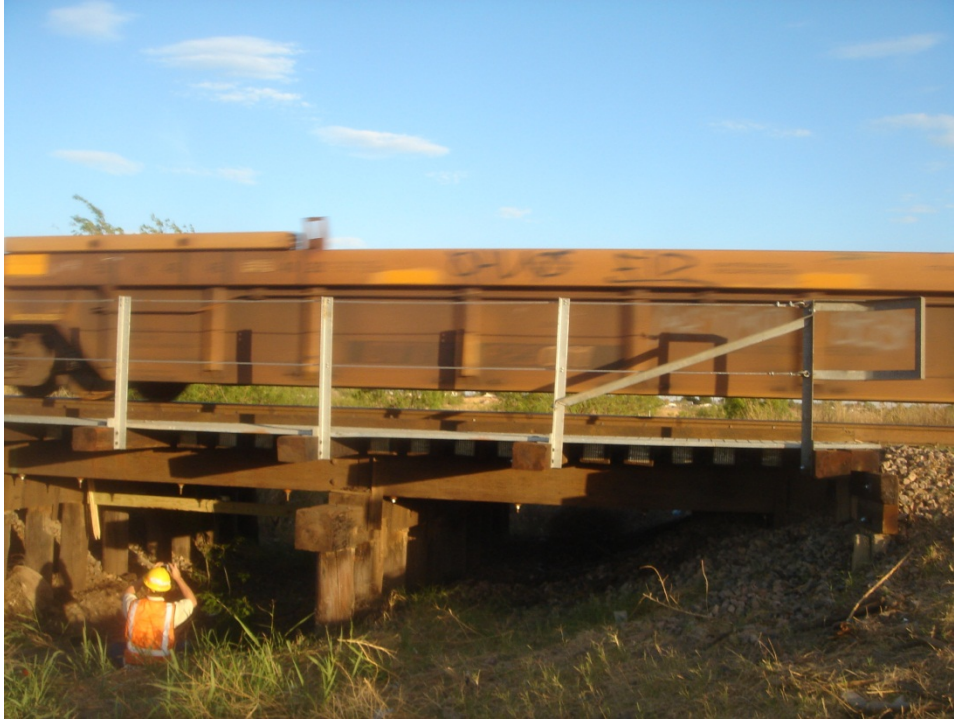
Figure C.53 Empty car crossing bridge.
