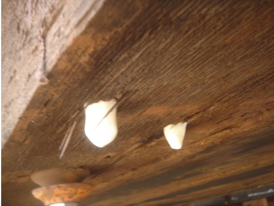
Figure C.41 Epoxy flowing through hole in bottom of beam.
