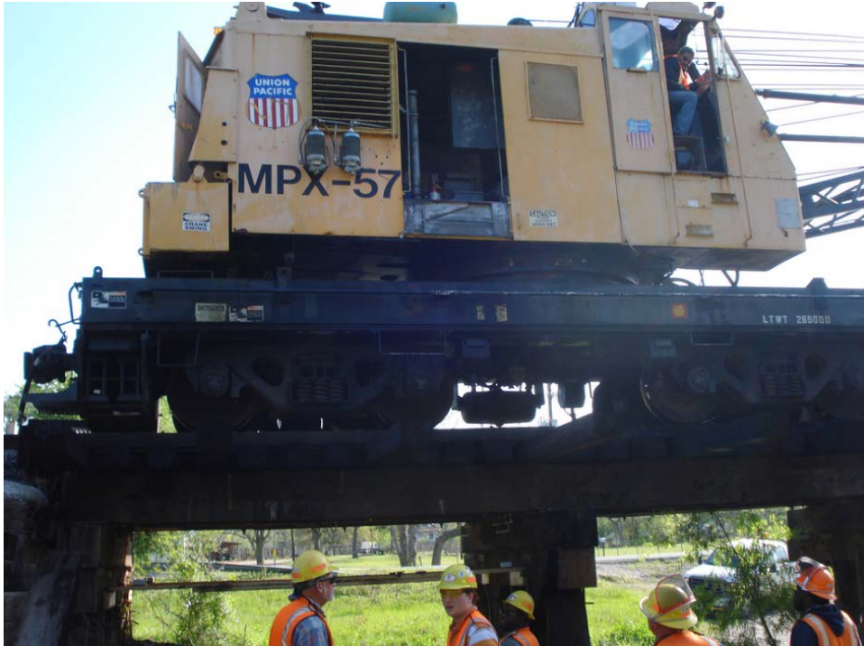
Figure B.17 Crane for loading bridge – Glidden Sub 69.11
