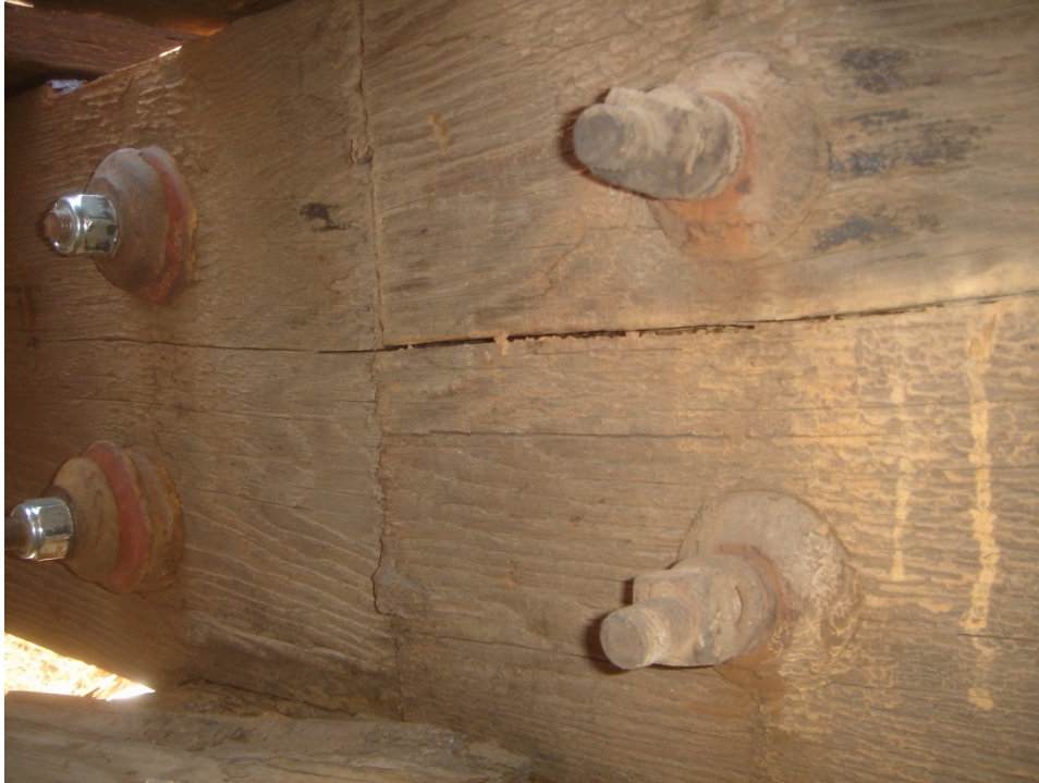
Figure C.19 Stringer 5 – Two members butted together over pier.
