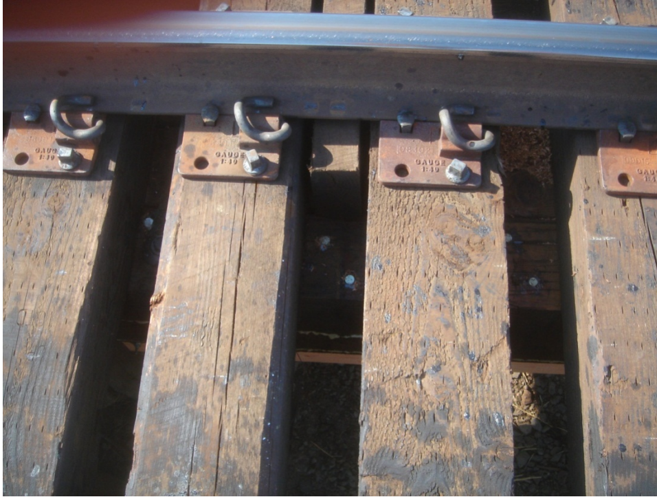
Figure C.43 Top view of spikes inserted in beams.
