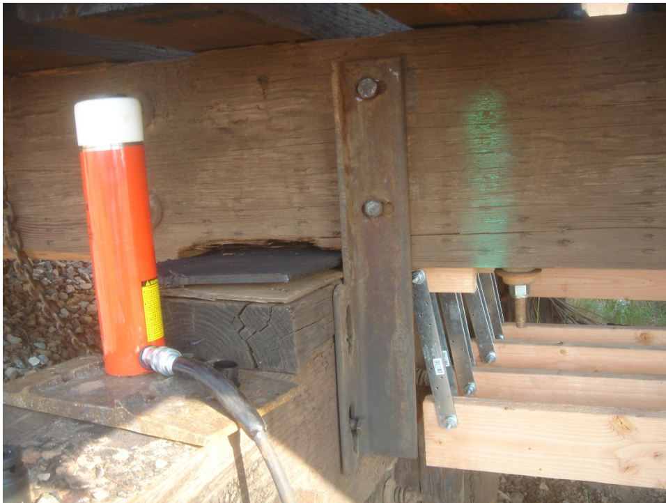
Figure C.34 Stringer 8 - Shim added below end of Span 1, Span 2
