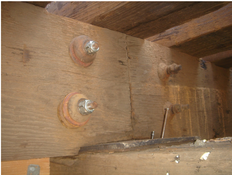
Figure C.20 Stringer 5, Spans 1 and 2 – Two members butted together over pier.
