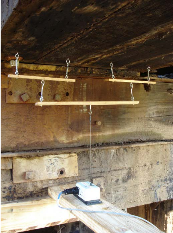
Figure B.2 Displacement measurement Set up for Glidden Sub 69.11
