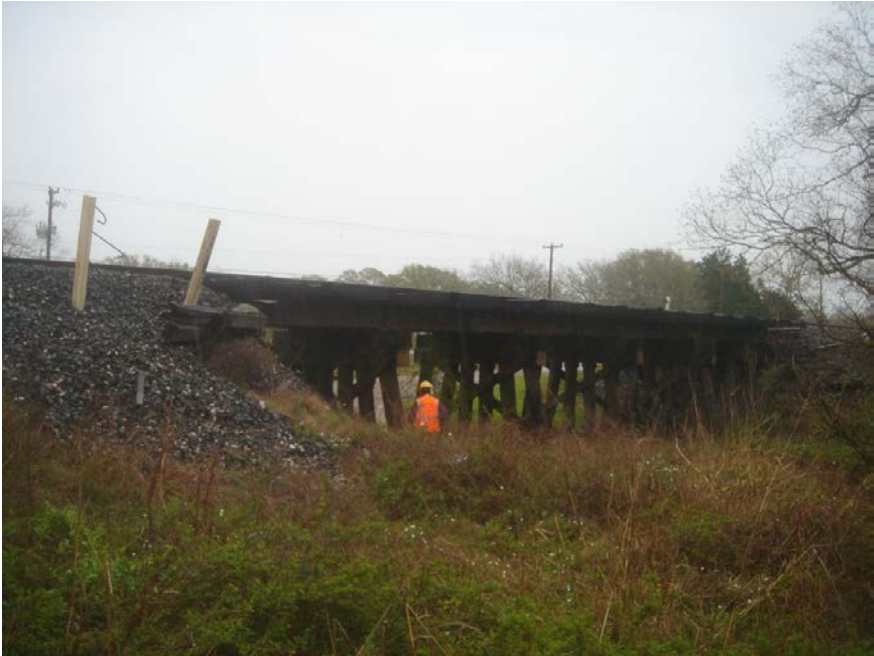
Figure B.1 Bridge No. 1 – Glidden Sub 69.11
