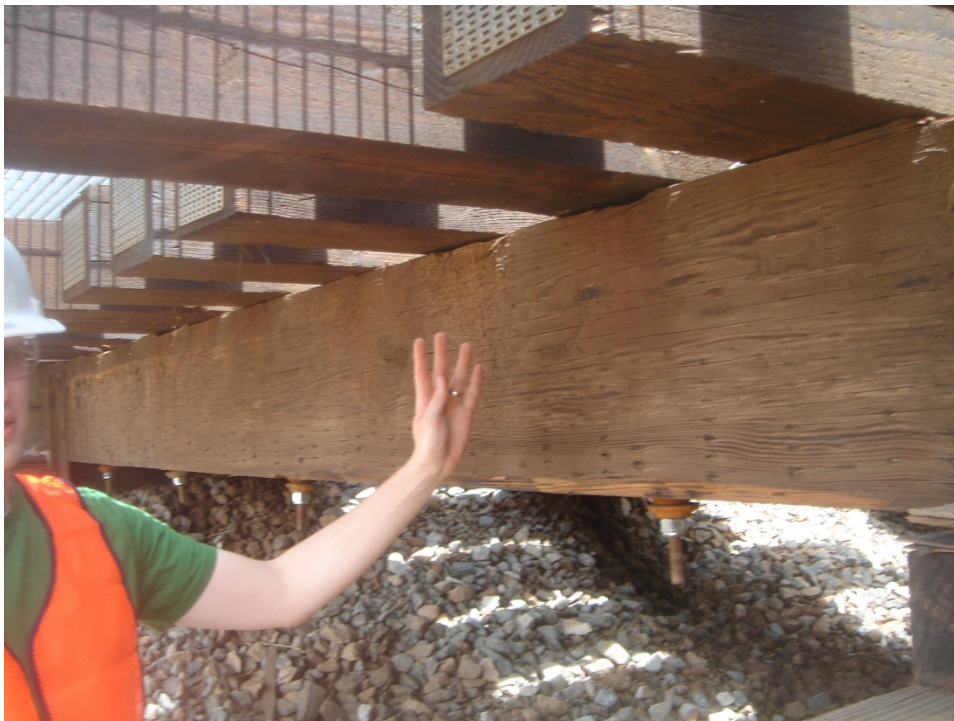
Figure C.24 Stringer 8, Span 1 – Minimal damage, despite 4A coding in inspection report.
