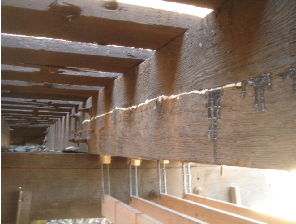
Figure C.39 Spray foam used to fill cracks
