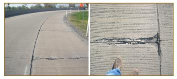
Photograph of field observation showing damage in pavement joints.
