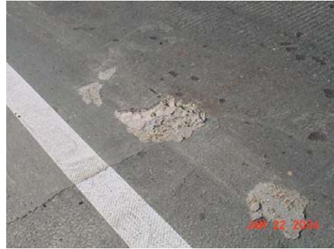
Figure 3.3.36. Spalling.
