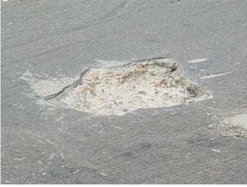
Figure 3.3.16. Severe spall.
