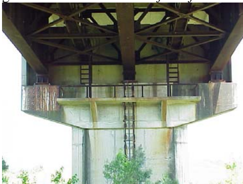
Figure 3.3.5. Corrosion of reinforcement
