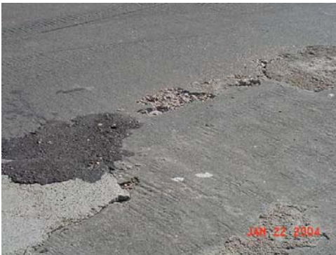
Figure 3.3.34. Spalling.
