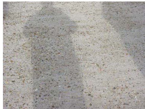
Figure 3.3.54 Light scale and wear.
