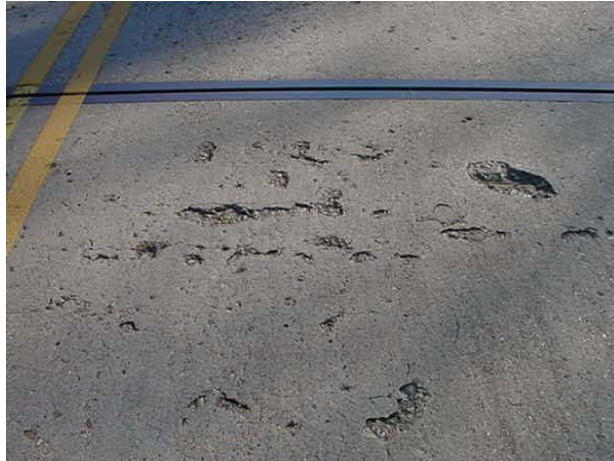
Figure 3.1.3 Light scale observed in MDOT District V.
