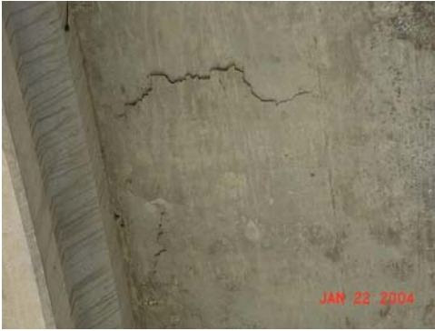
Figure 3.3.39. Delamination.
