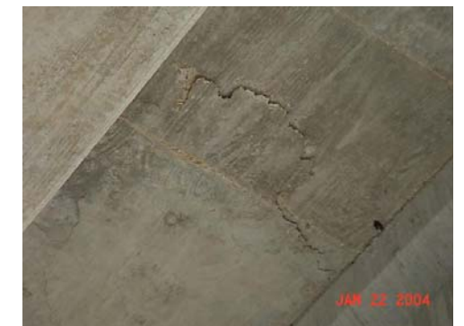
Figure 3.3.44. Delamination.
