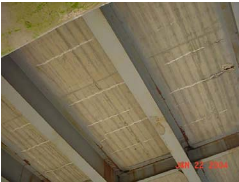
Figure 3.3.41. Efflorescence.
