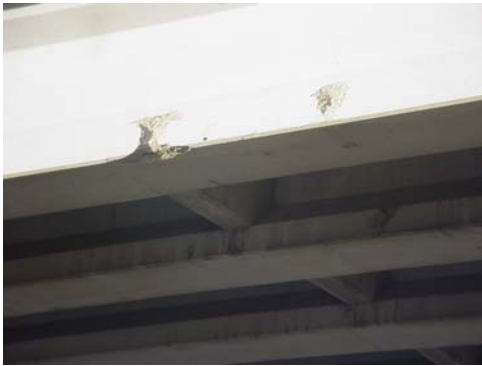
Figure 3.3.51. Collision damage.
