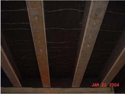
Figure 3.3.33. Efflorescence.
