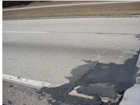
Figure 3.3.50. Severe spalling.
