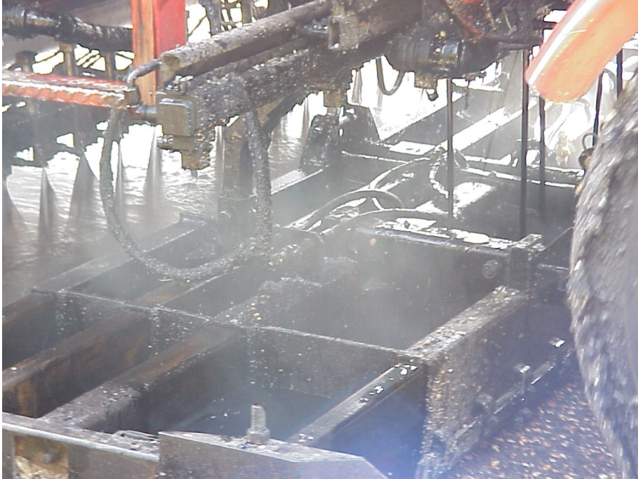
Figure 13 – Spreader Box Full of Sealant
