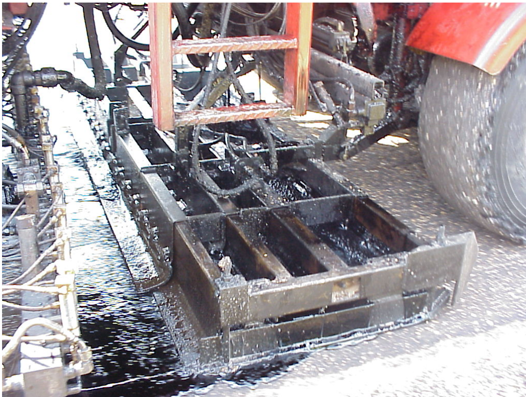
Figure 12 – Application of DRM Sealant
