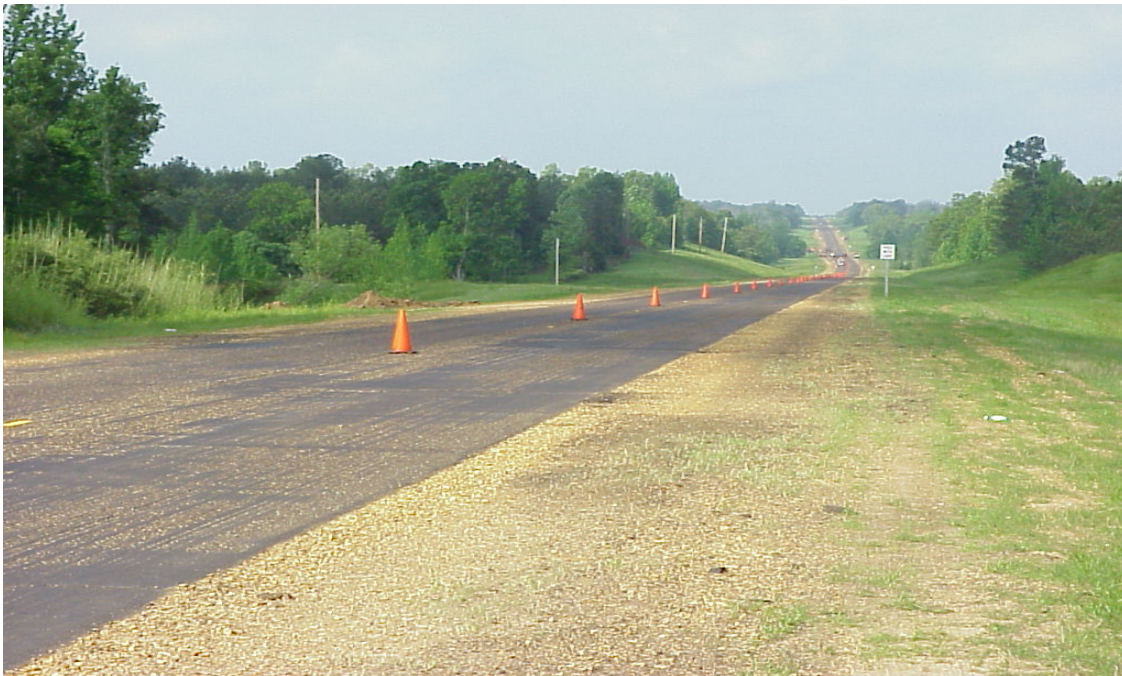
Figure 8 – Test Section After Milling
