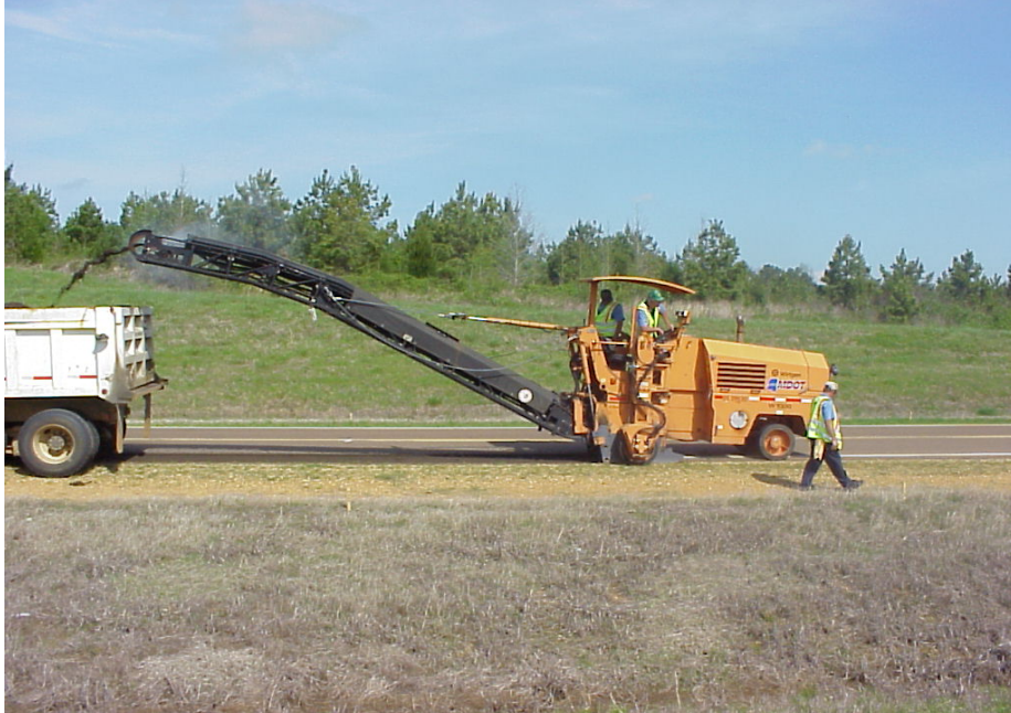
Figure 7 – Continued Milling
