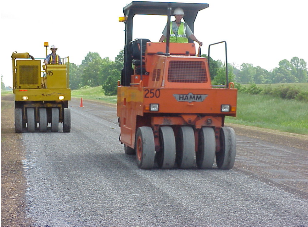
Figure 18 – Rolling the DRM
