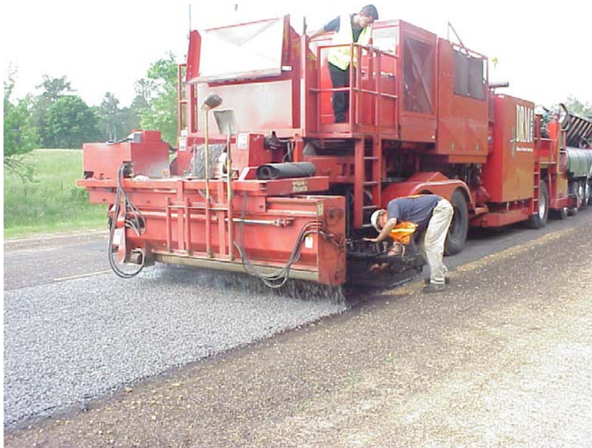
Figure 16 – Aggregate Being Spread
