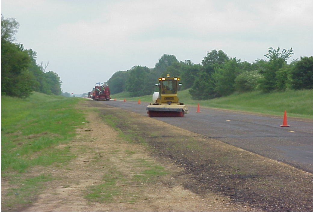
Figure 9 – Cleaning the Milled Surface
