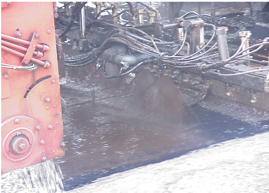
Figure 14 – Application of DRM Emulsion
