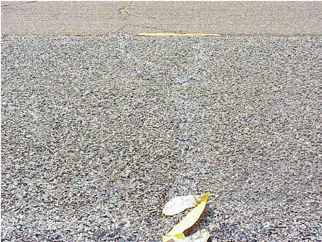
Figure 21 – After DRM and Rolling
