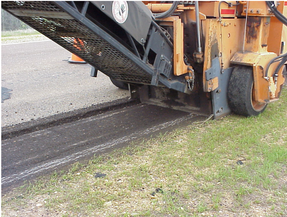
Figure 6 – Milling
