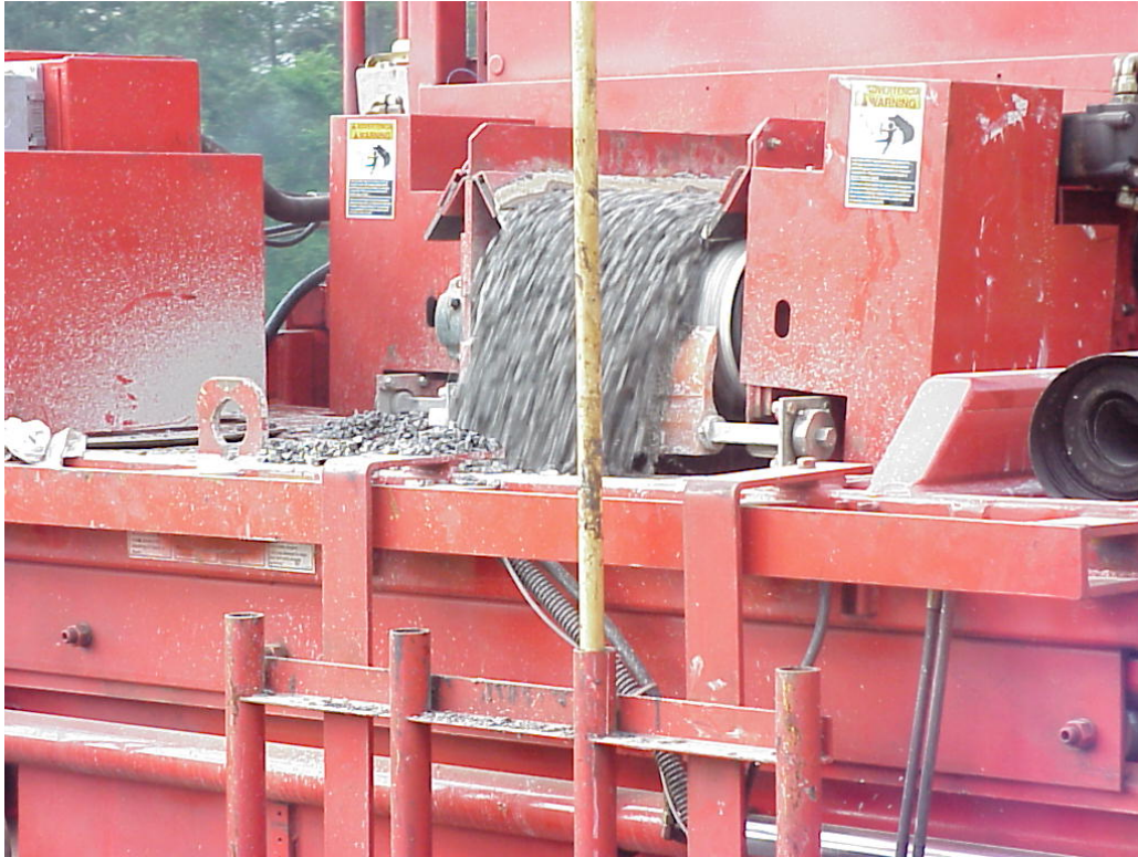
Figure 15 – Aggregate Fed into Spreader
