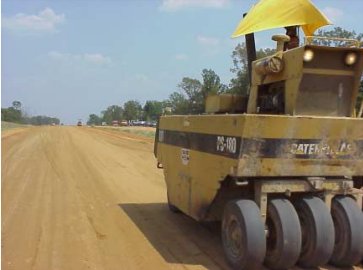
Figure 43. Compaction with a Rubber Tire Roller
