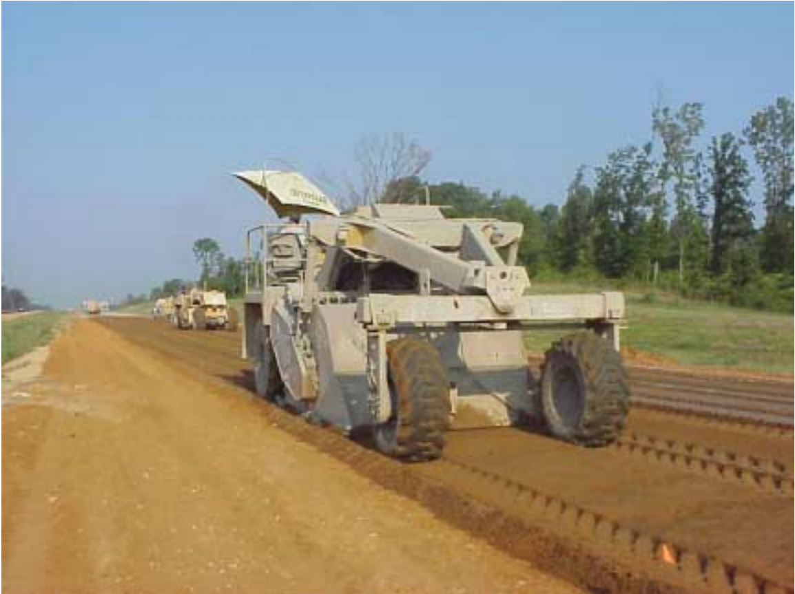
Figure 39. Pulvamer Used for Blending LFA, Soil, and Water
