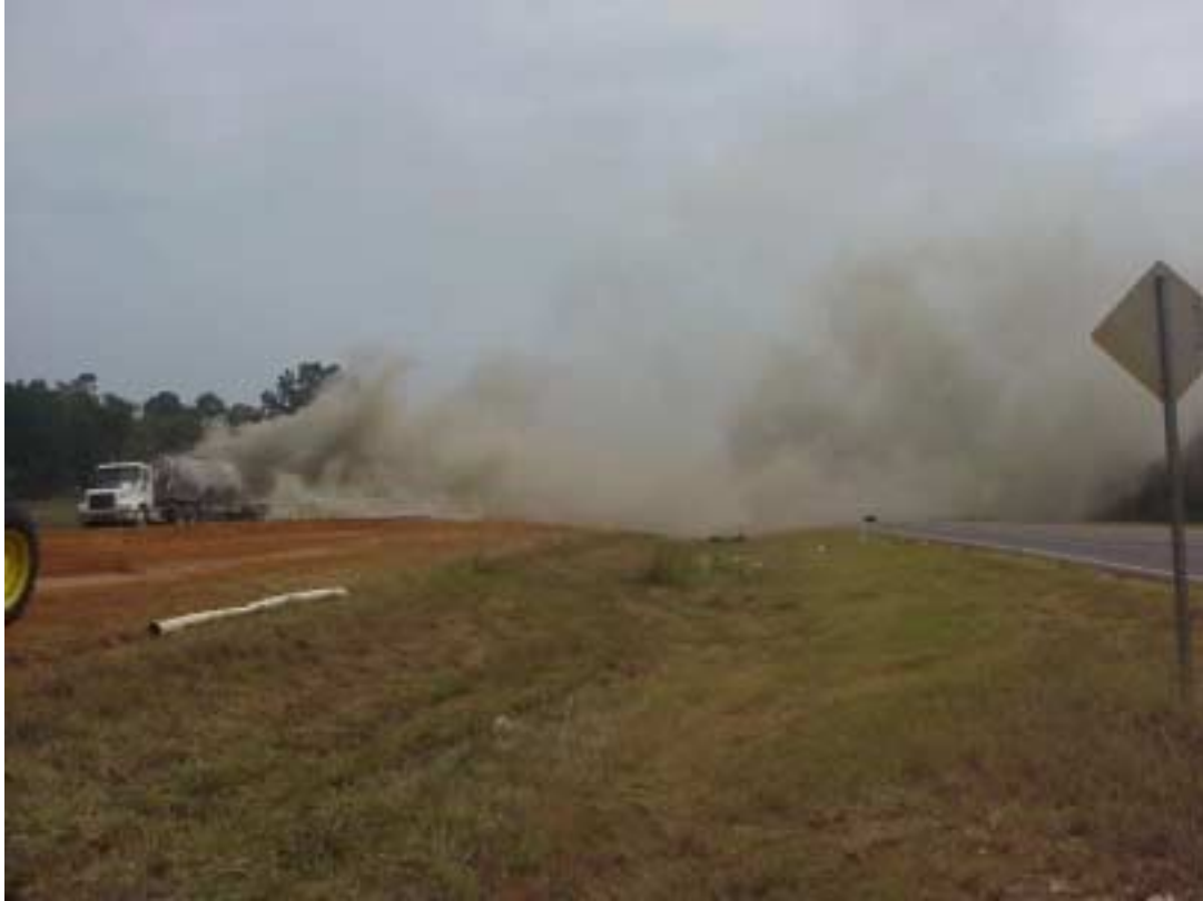
Figure 35. Dust Problem Associated with Current Method of Spreading Lime and Fly Ash
