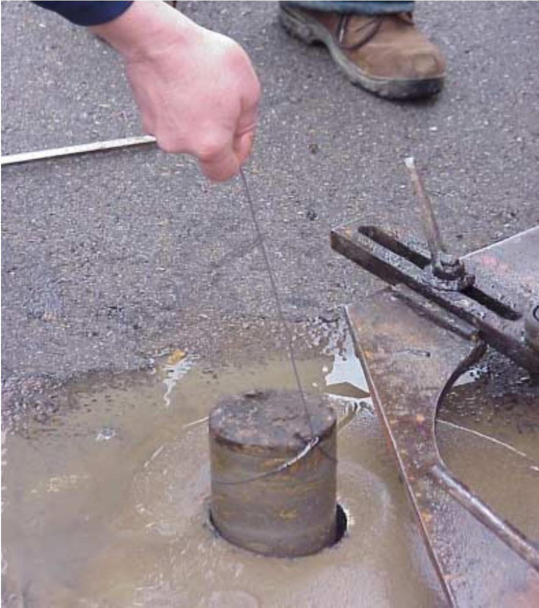
Figure 3. Method Used to Extract LFA Cores from Pavement
