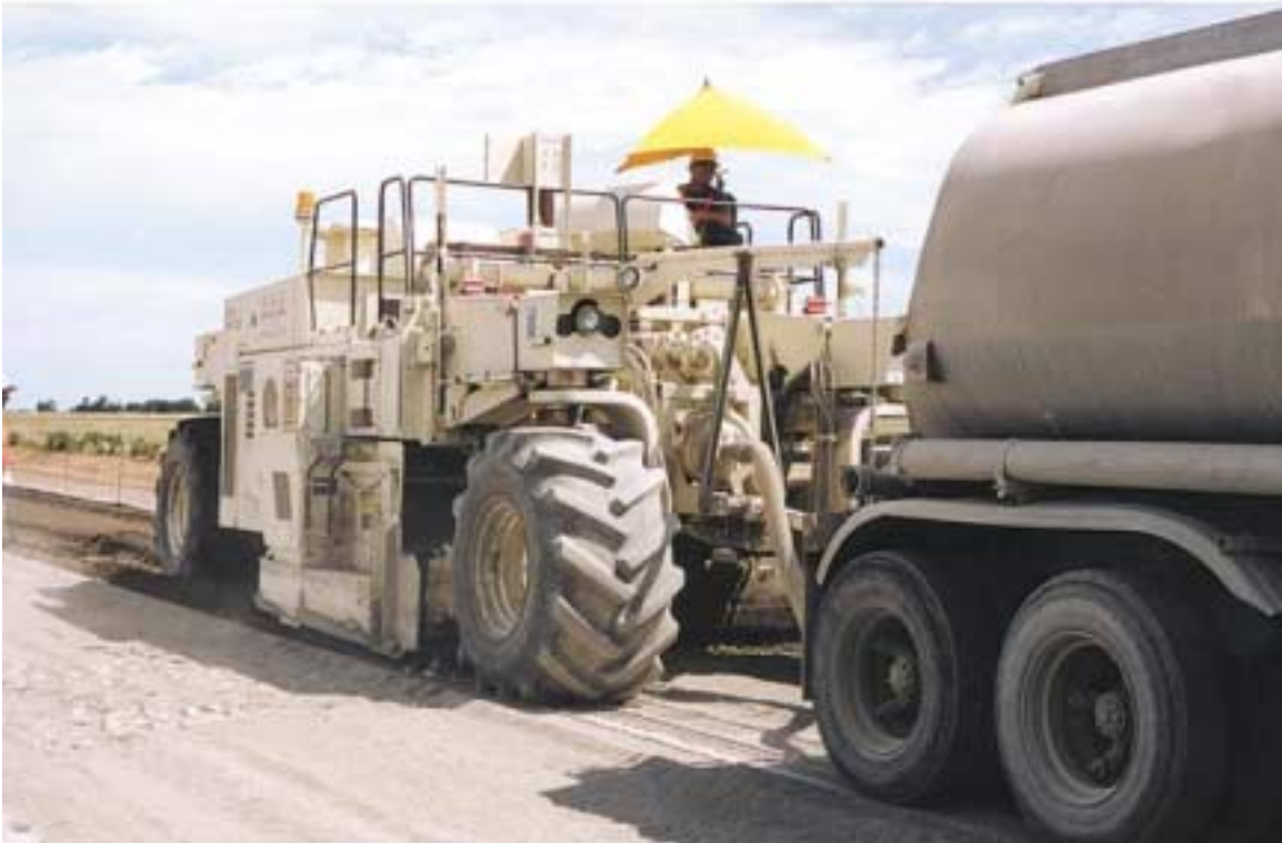
Figure 38. Proposed Method of Nursing to Incorporate Water Into LFA and Soil Blend (Photo courtesy of Halsted)
