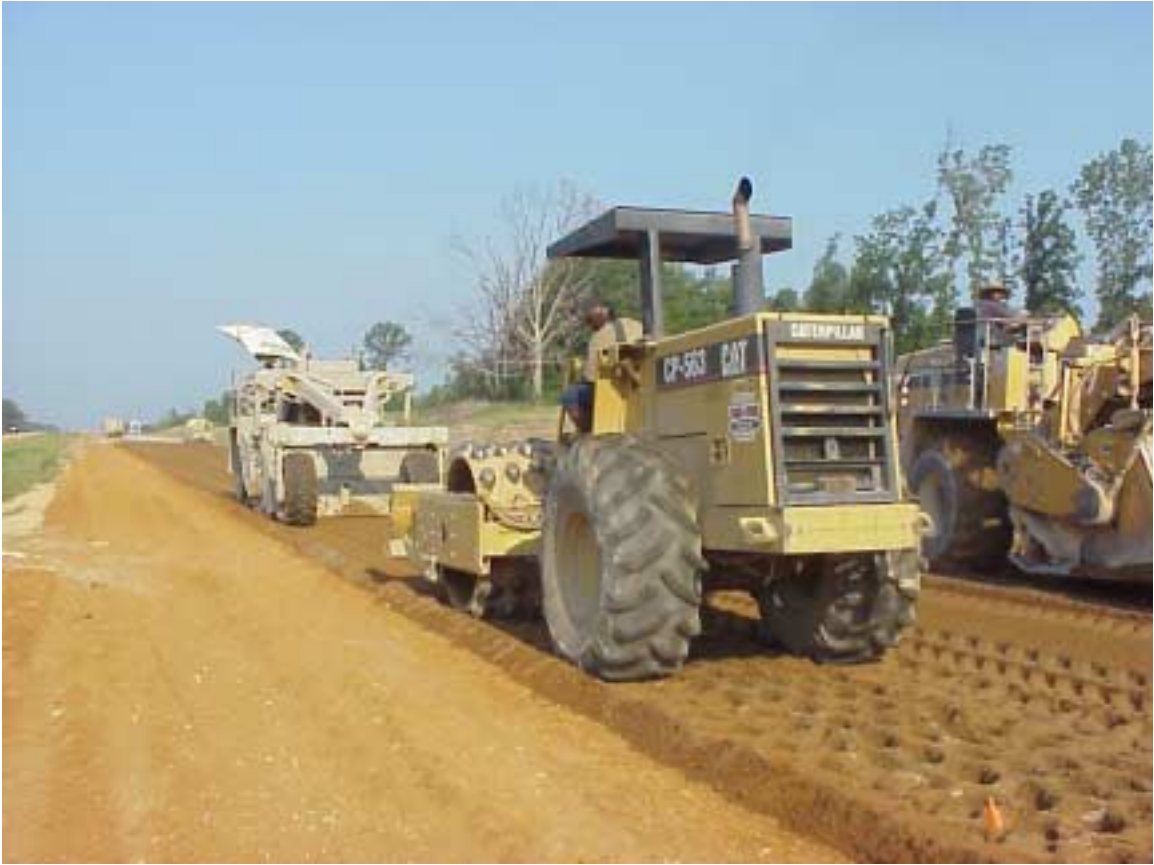
Figure 42. Compaction with a Sheepfoot Roller
