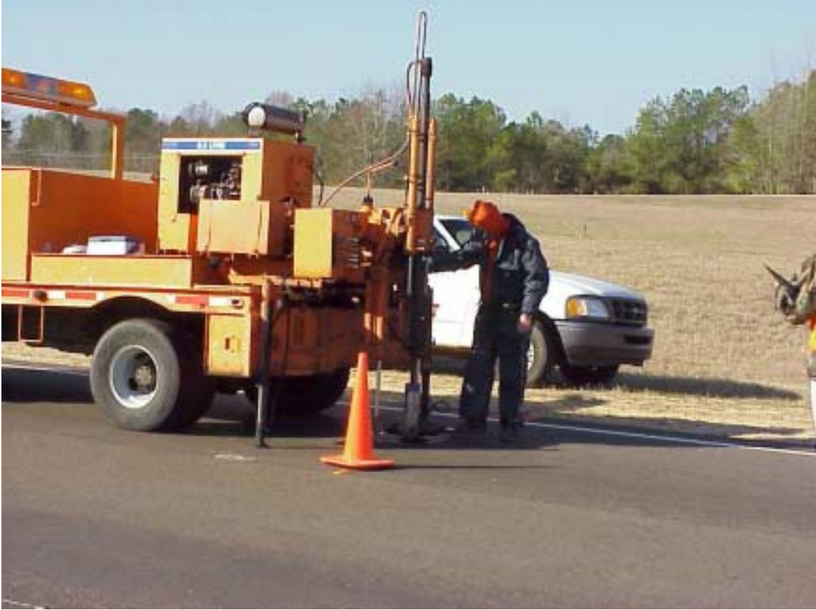
Figure 2. Drill Rig Used for Obtaining LFA Cores
