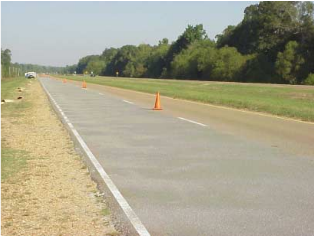
Figure 14 – Completed E-Krete application
