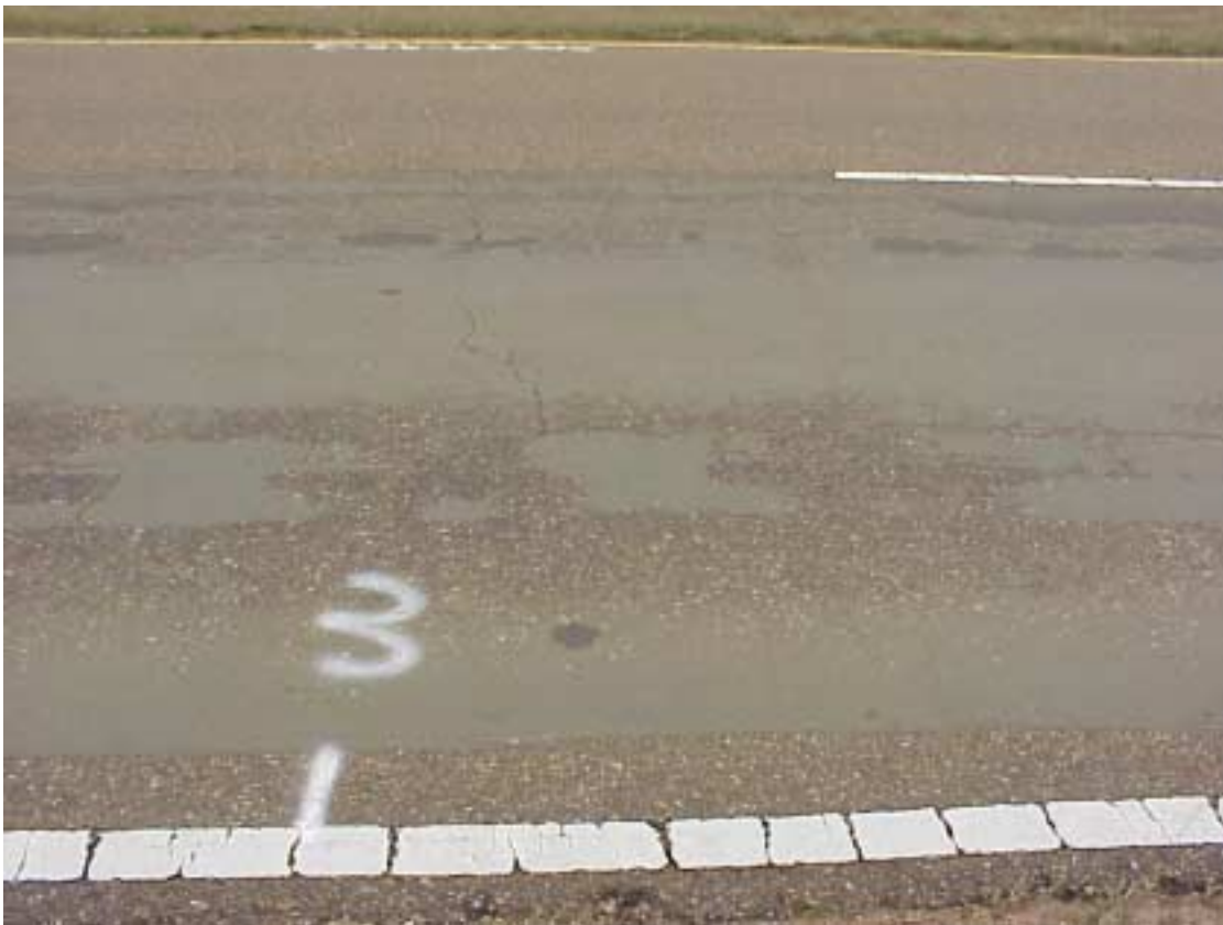
Figure 21 – Wearing of E-Krete after one year
