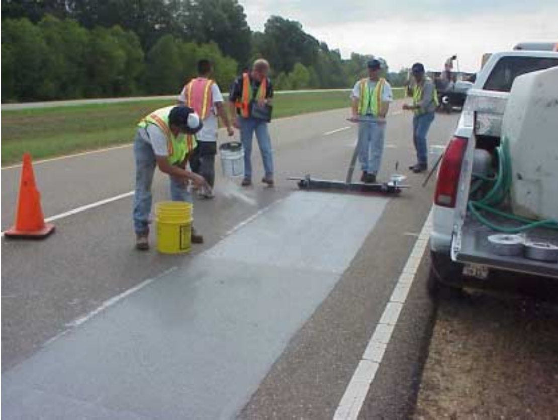
Figure 10 – Broadcasting of Georgia granite on fresh E-Krete for skid resistance
