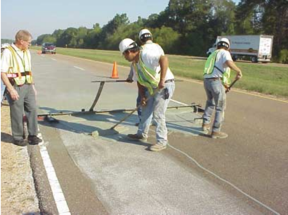
Figure 13 – Using squeegees to distribute E-Krete ahead of the 10'-6" screed
