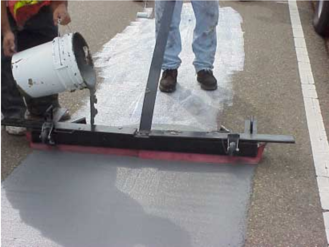
Figure 8 – 4 foot wide screed application for initial application of E-Krete
