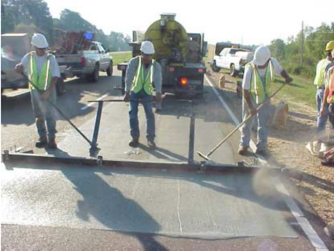
Figure 12 – 10'-6" Screed utilized for the final surface application
