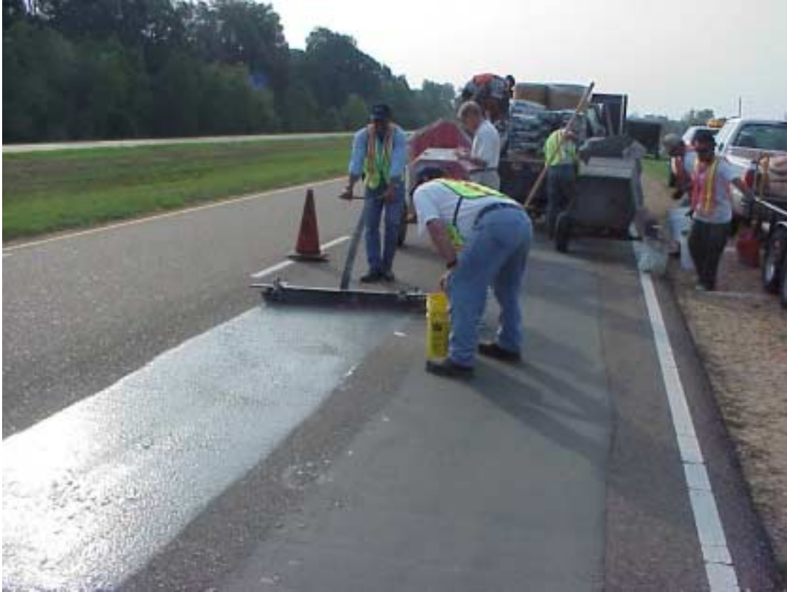
Figure 11 – Second day of construction utilizing two mortar mixers
