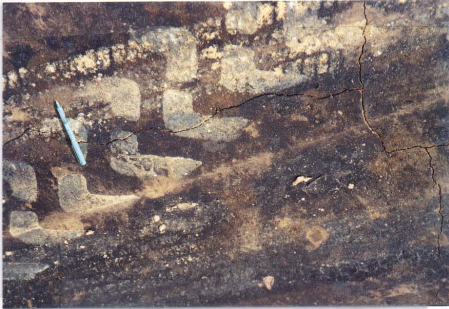
Figure 4.24 High severity cracks in section 6, lime – fly ash, 241 + 50, fourteenth day.
