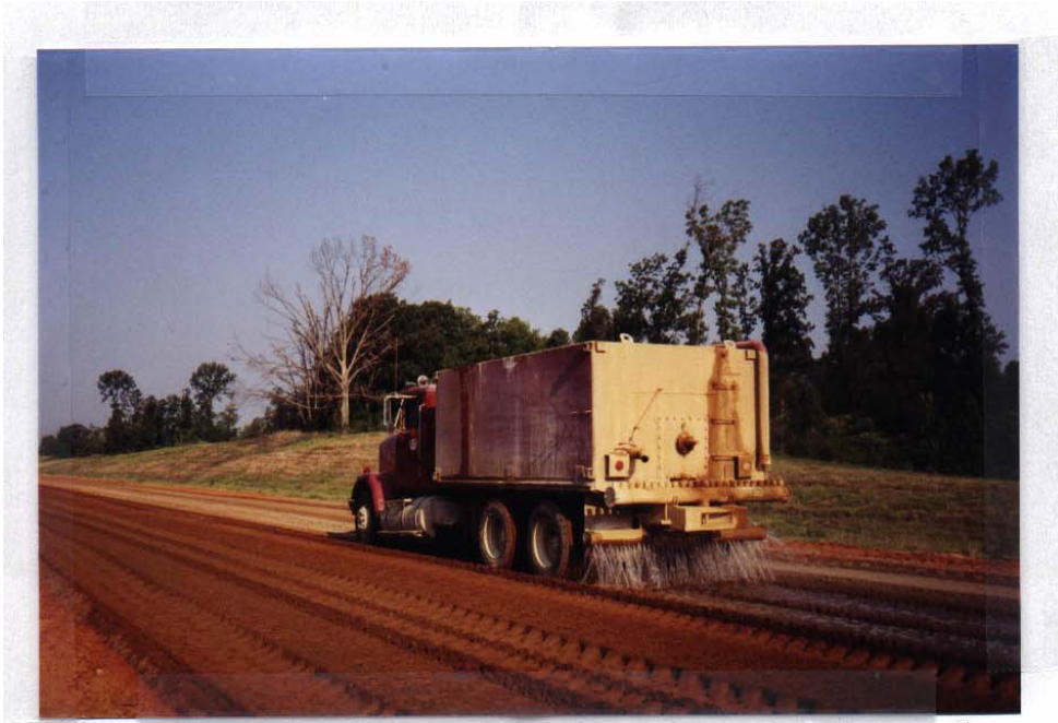
Figure 4.2 Water being added to the dry-mixed soil and additive(s).
