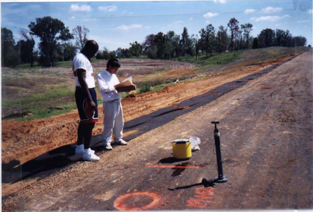
Figure 4.28 View of geogauge (left) and Clegg impact hammer (right).
