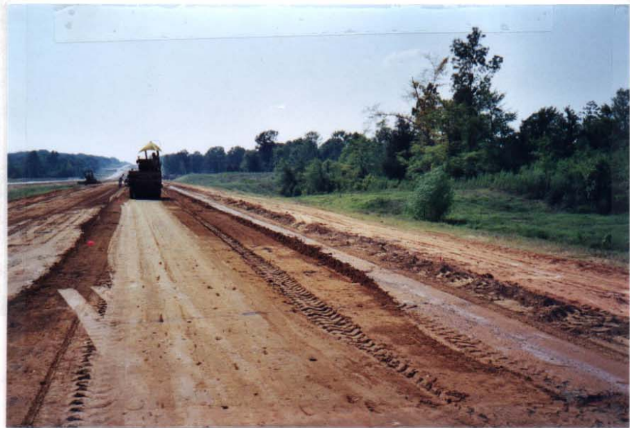
Figure 4.5 Finish-compaction by rubber-tired roller.
