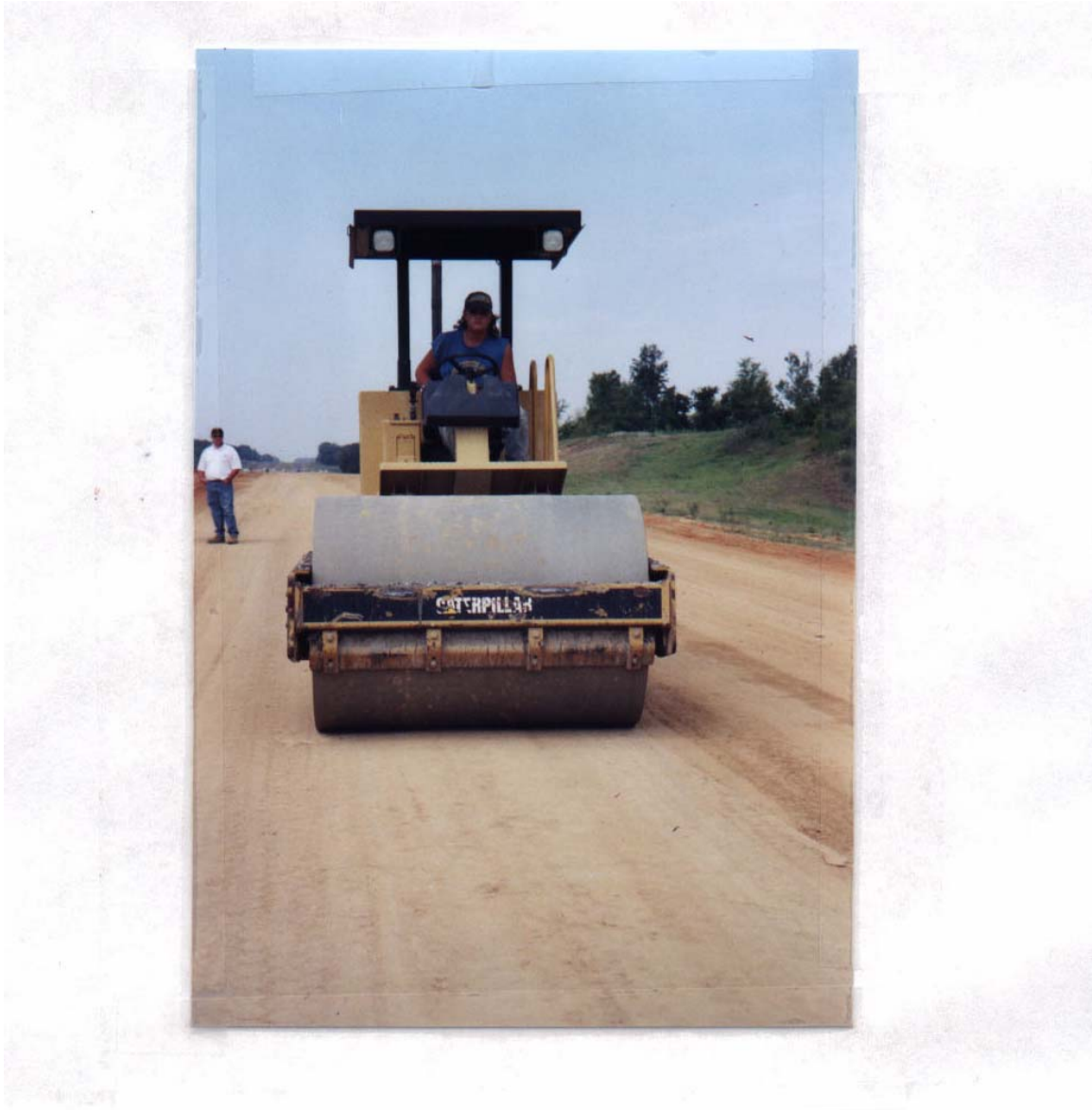
Figure 4.9 Vibration roller in operation precracking the layer after 24 hours.
