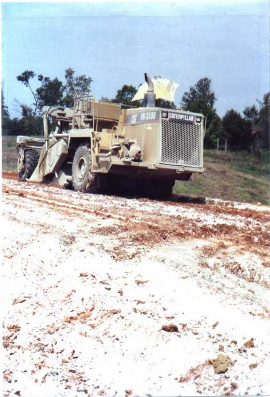
Figure 4.1 Dry mixing soil and lime employing a rotary mixer.
