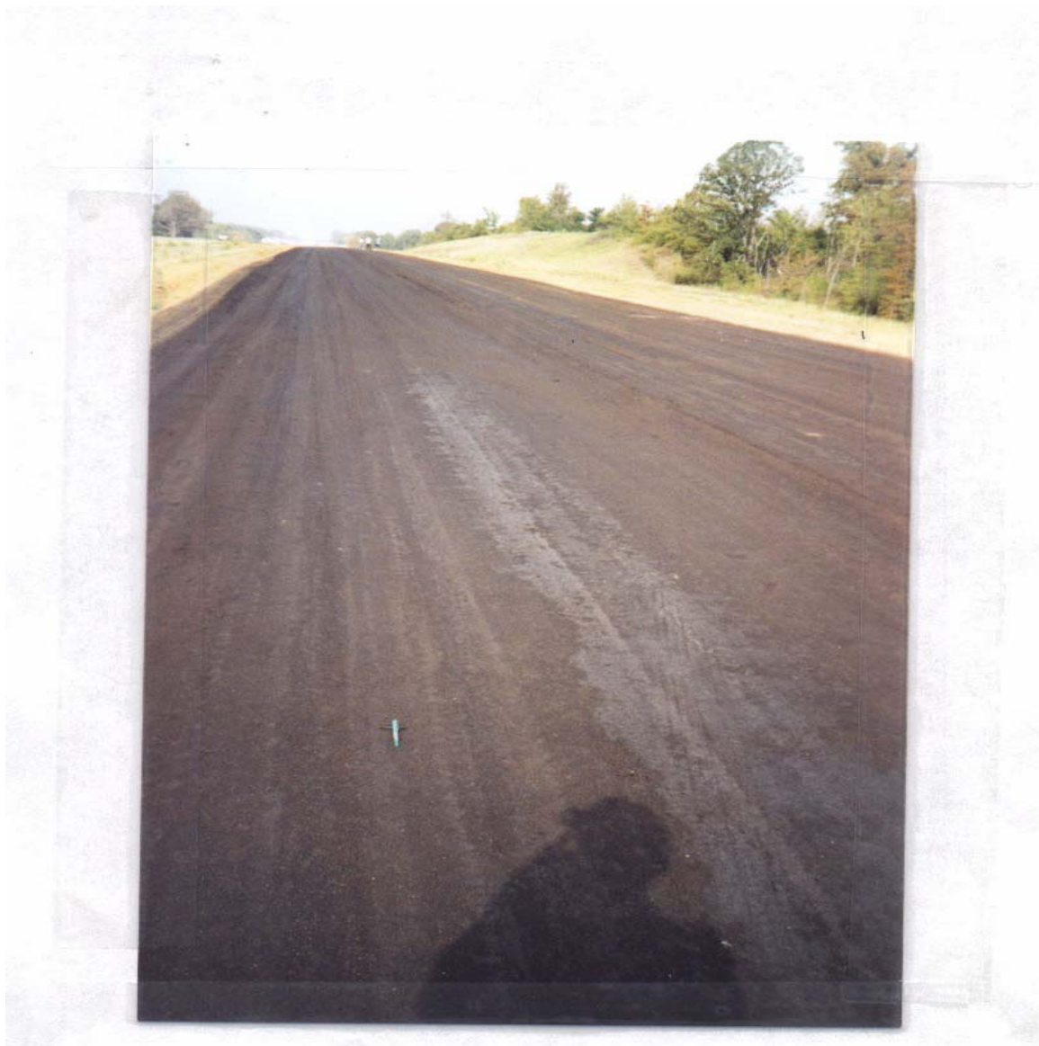
Figure 4.21 Crack-free surface of section 2 (precracked), fourteenth day.
