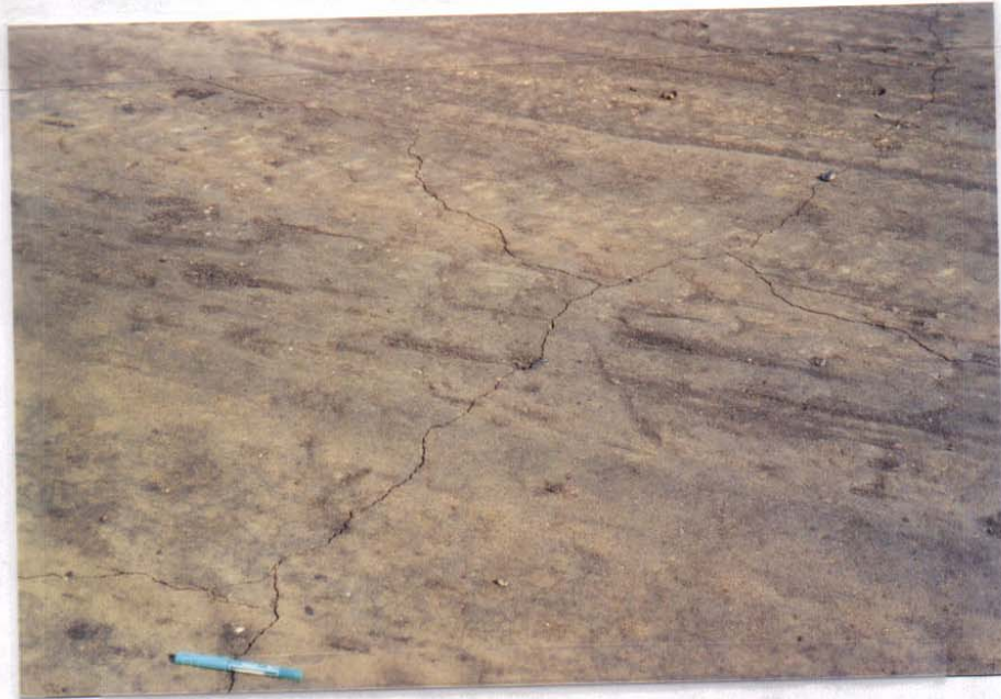
Figure 4.22 Random cracks in section 3A, control cement, fourteenth day.
