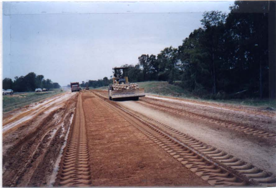
Figure 4.4 Initial compaction by sheep-foot roller.
