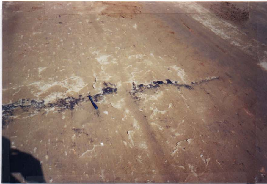
Figure 4.13 Close-up view of a precut joint.
