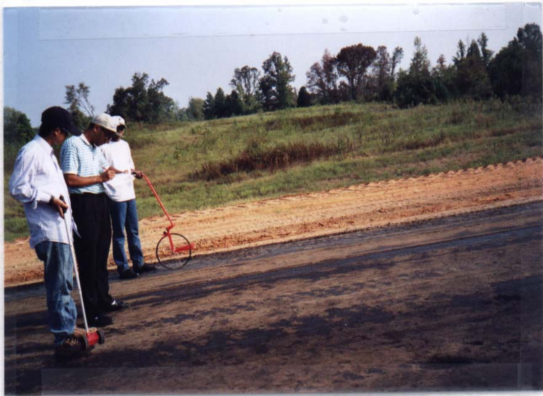
Figure 4.17 Survey crew measuring and mapping cracks.
