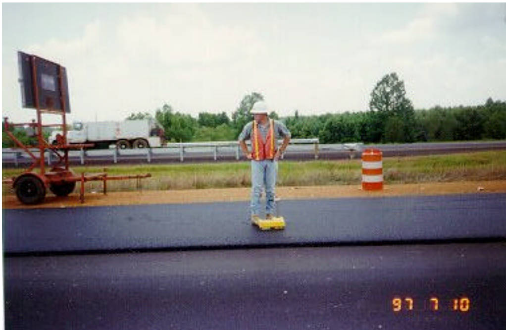
Figure 2.41 Checking density of surface mix.
