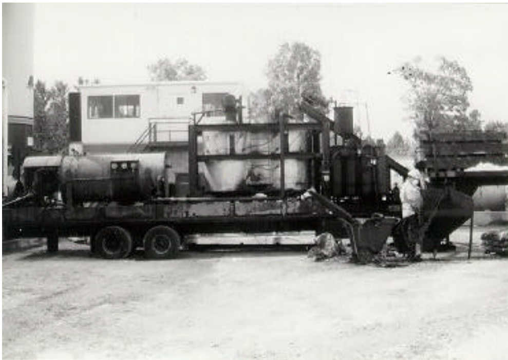
Figure 2.18 Blending unit in place at plant.
