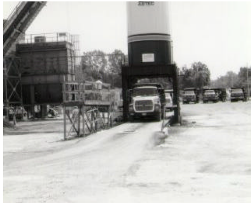
Figure 2.16 Truck loaded from surge silo
