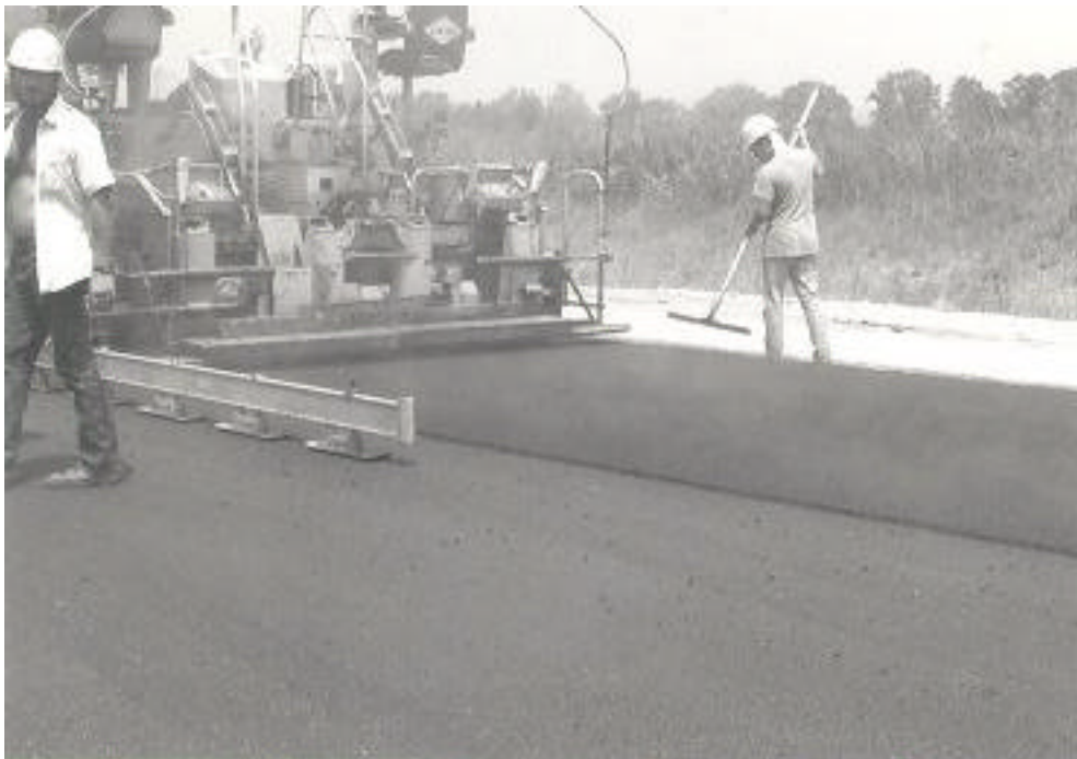
b. Paving of outside lane.
