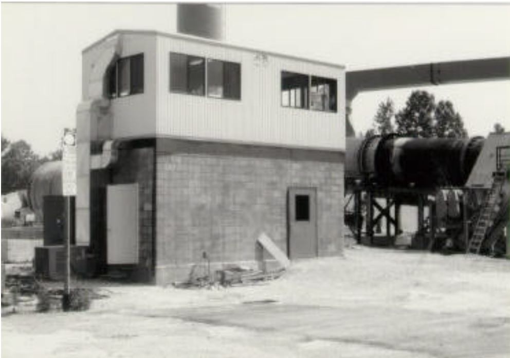
Figure 2.6 Plant control room.
