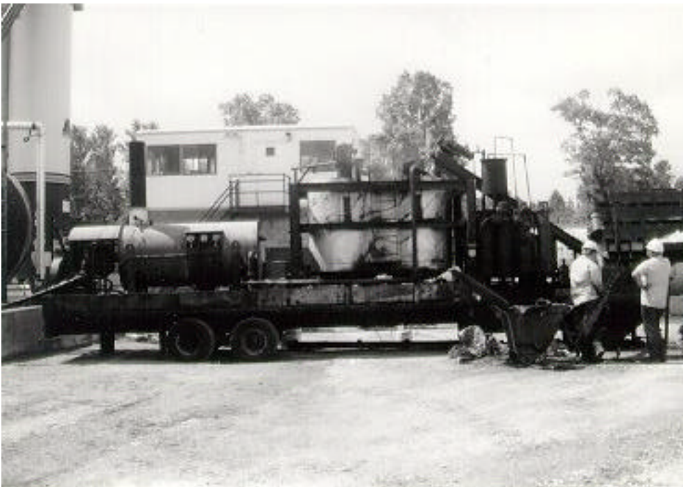
Figure 2.20 Auger transport of crumb rubber to primary tank.
