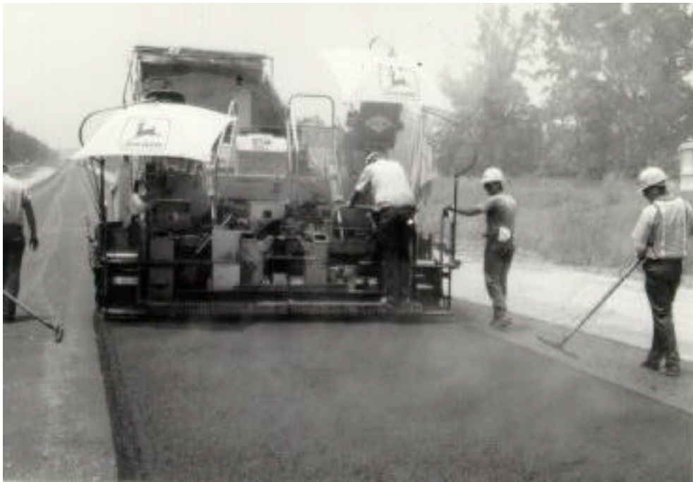
Figure 2.26 Surface course for control section.
