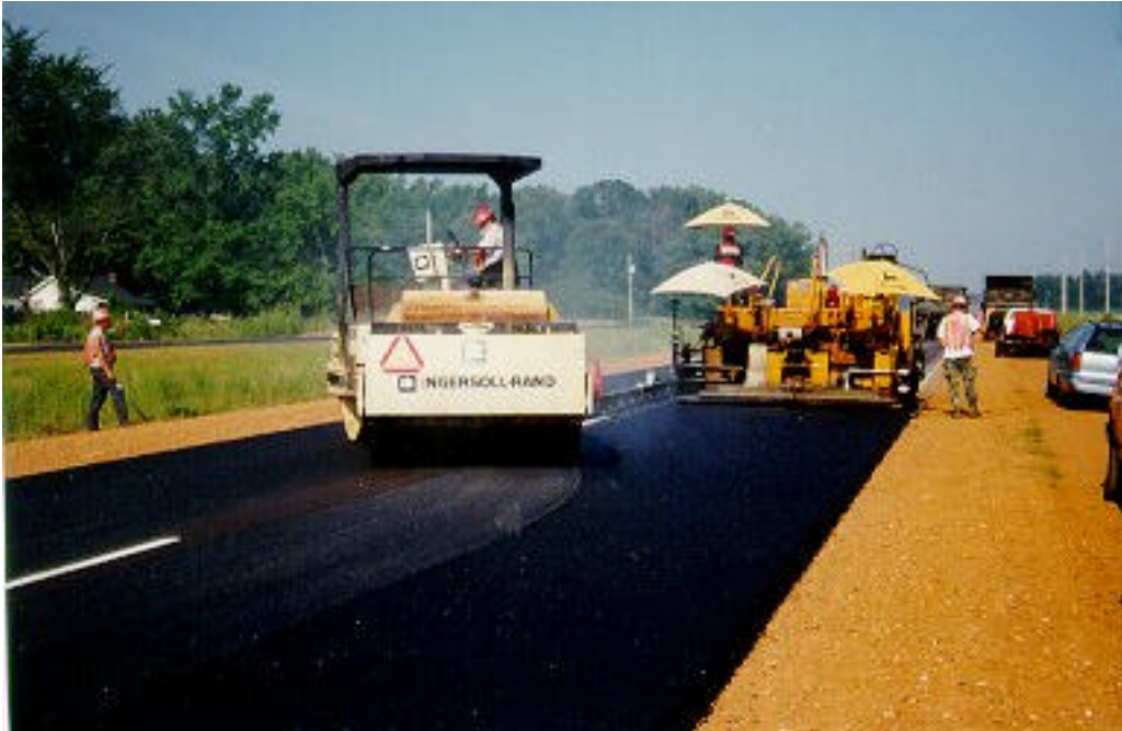
Figure 2.40 Rolling of surface mix with CRM RAP.
