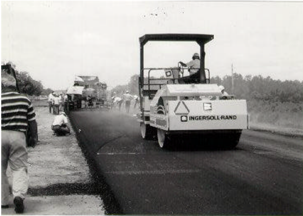
Figure 2.32 Vibratory roller used behind paver.
