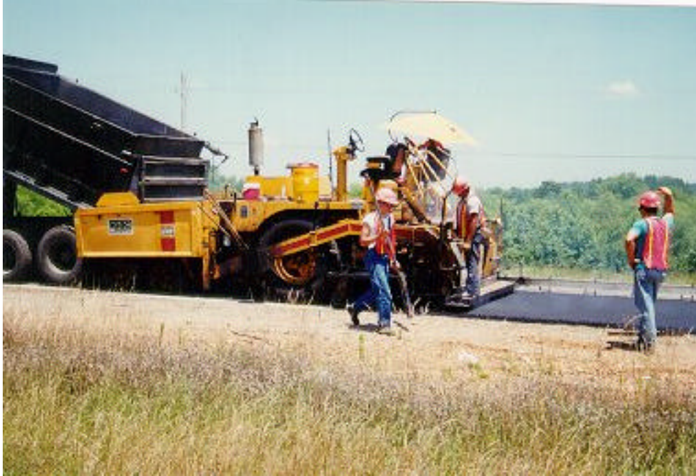
Figure 2.38 Placement of regular HMA in milled areas.
