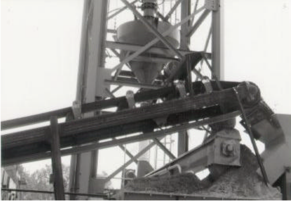
Figure 2.11 Lime added to materials.
