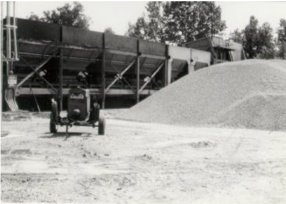
Figure 2.8 Material stockpile and hoppers.
