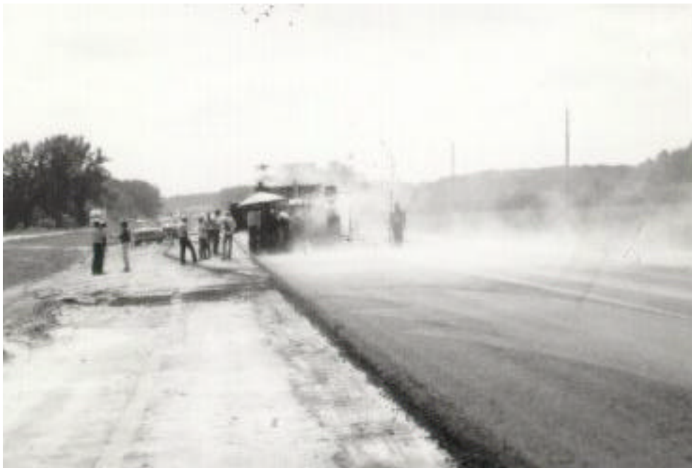
Figure 2.28 Smoke created at and behind paver.
