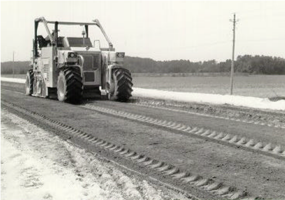
Figure 2.23 Lime fly-ash treated base course.
