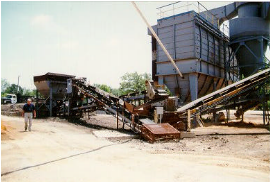
Figure 2.22 Separate hopper and moving belt for CRM RAP.
