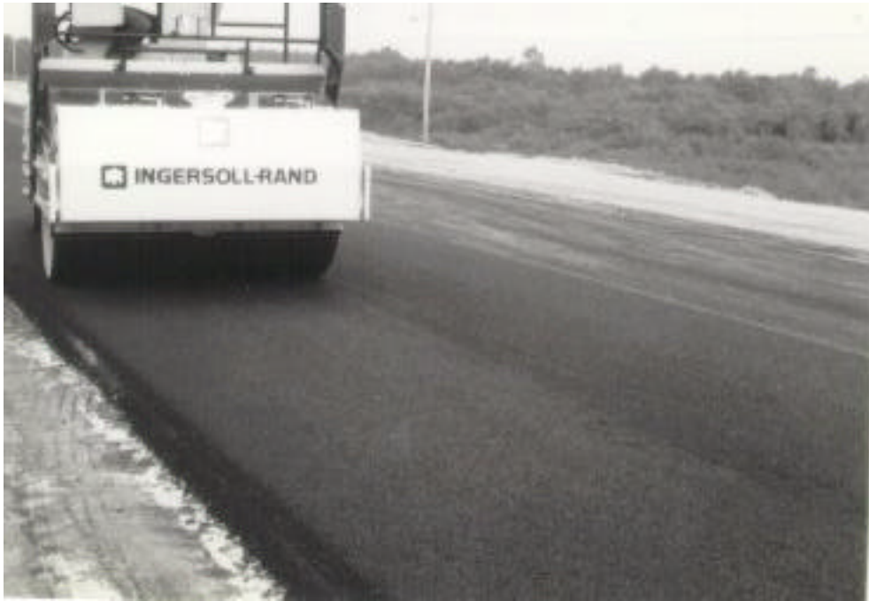
Figure 2.25 Binder course for control section.
