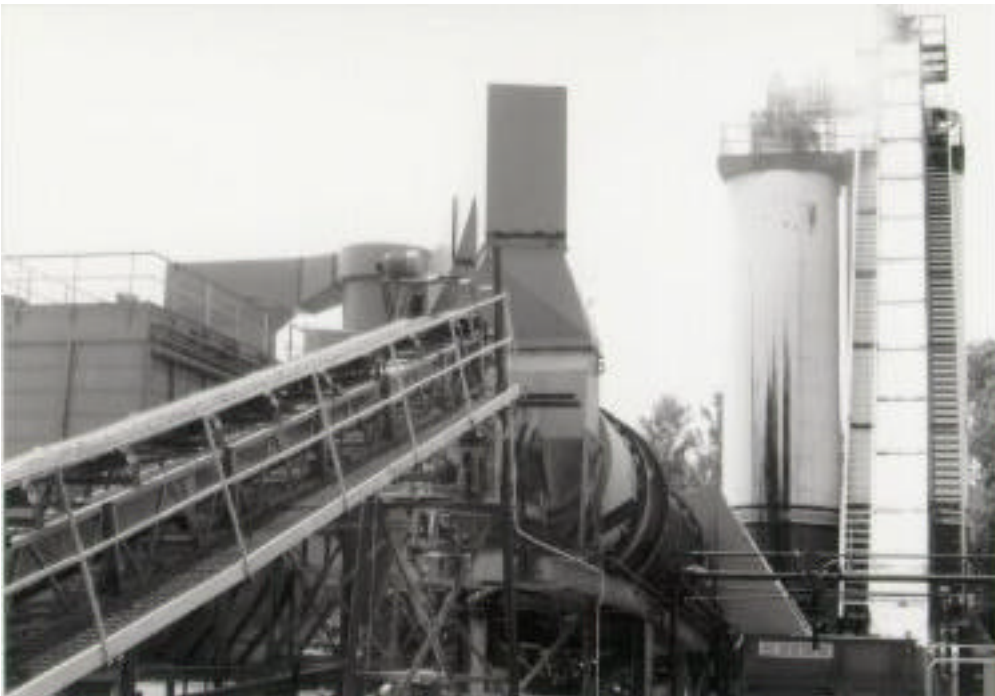
Figure 2.12 Aggregate transport to drum mixer.
