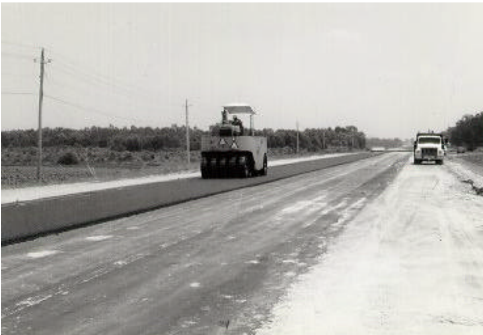
Figure 2.24 Completed base course.
