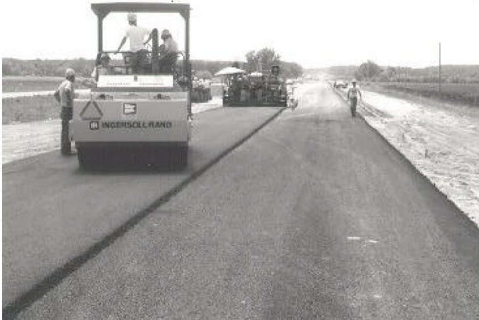
a. Paving of inside lane.
