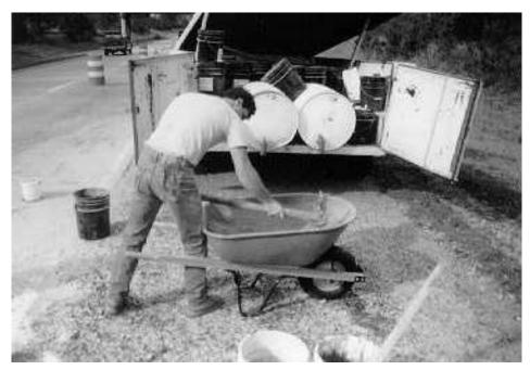
Figure 11. Mixing RESURF II.
