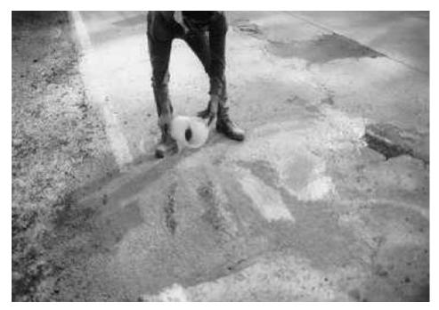
Figure 14. Painting the patch with resin.
