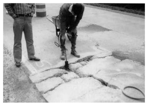
Figure 5. Drying with a burner.
