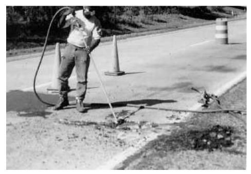
Figure 3. Cleaning out with air.
