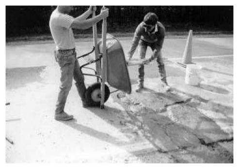
Figure 12. Filling the clean hole.
