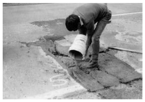
Figure 9. Filling the cracks with RESURF CR.
