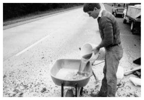
Figure 10. Combining RESURF II mix with the resin.
