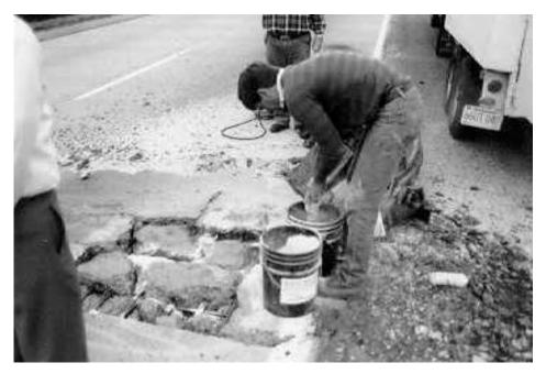
Figure 8. Mixing RESURF CR with resin.
