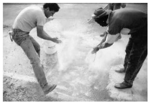
Figure 15. Broadcasting RESURF II aggregate.
