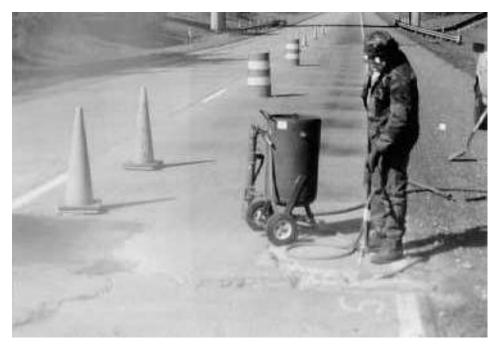
Figure 4. Sandblasting holes.
