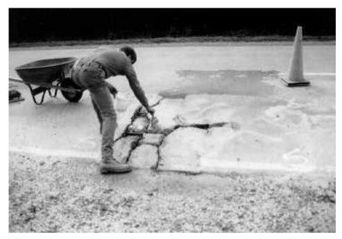
Figure 7. Painting resin on the patch.
