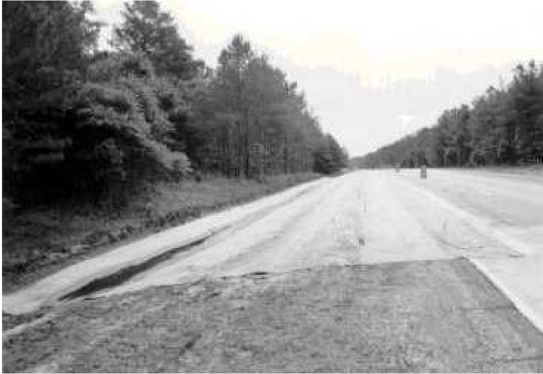
Figure 5. Fabric installed in median ditch.
