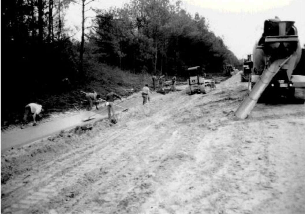
Figure 7. Installing concrete ditch.
