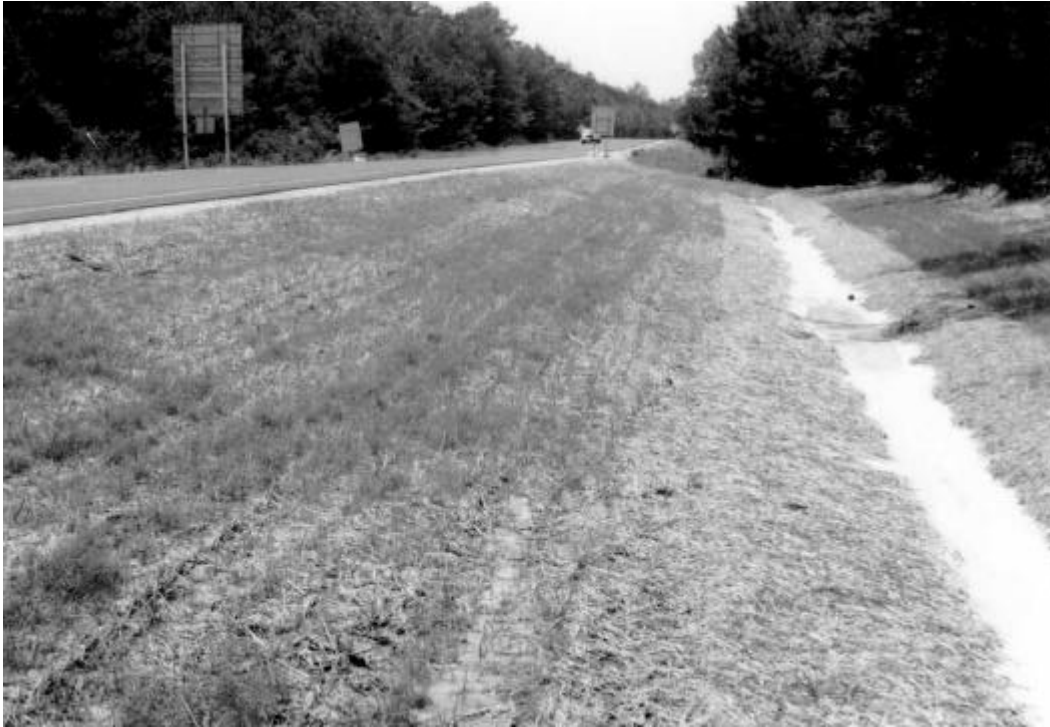
Figure 9. A finished ditch.
