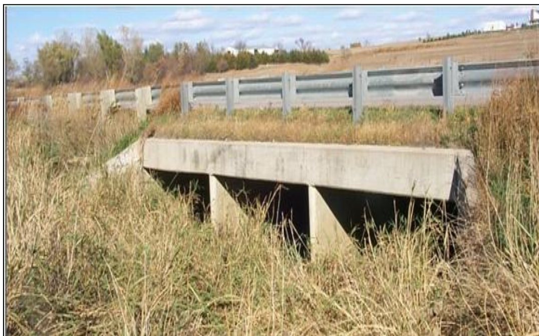
Figure 8. Guardrail installed to shield culvert opening
