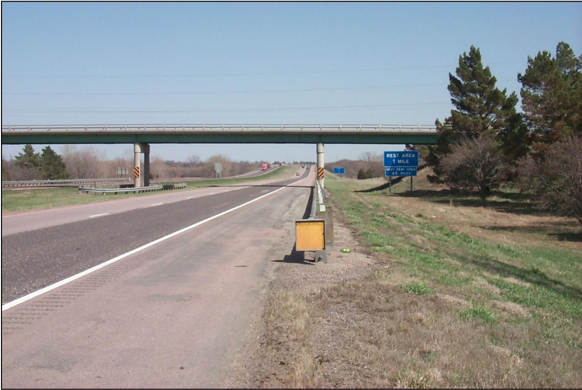
Figure 20. Tangent guardrail installation
