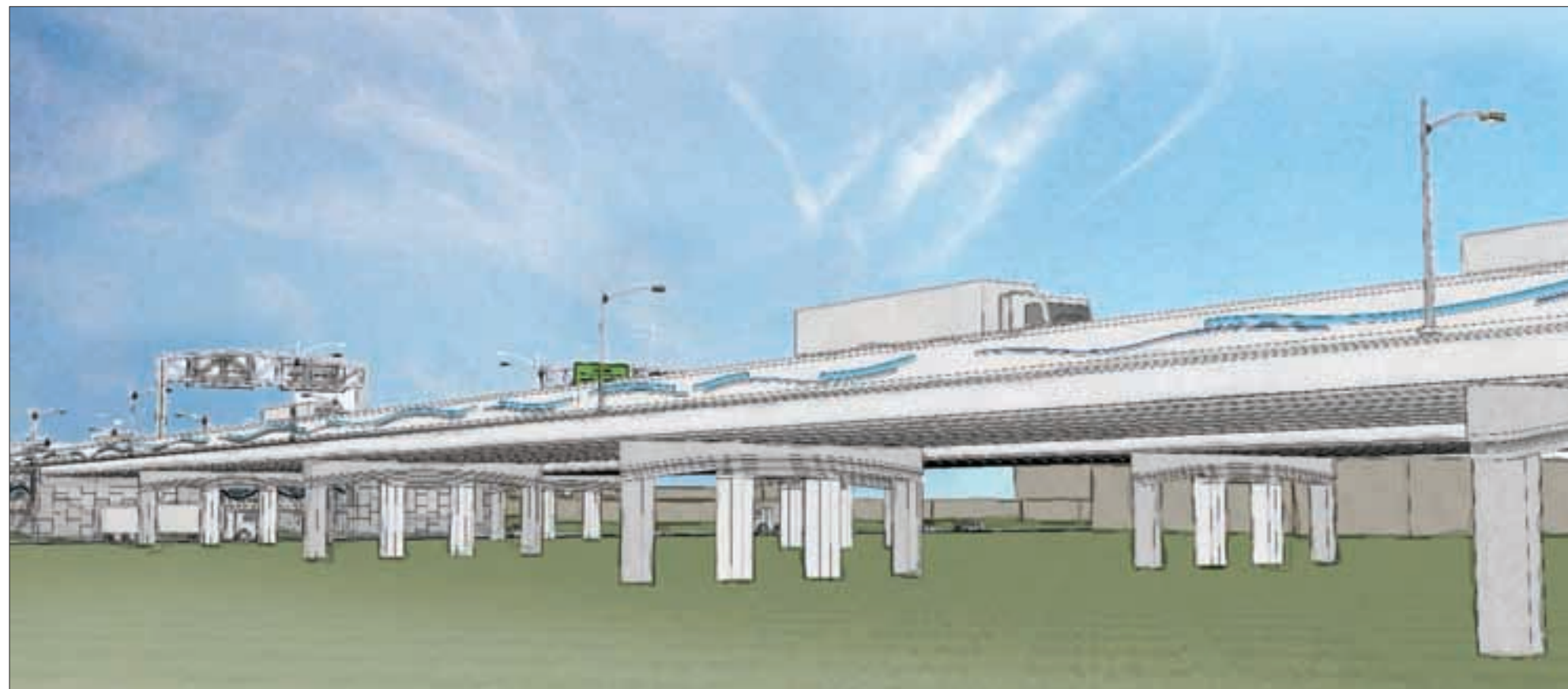
Figure 3.6 – Pier Concept at Mainline Bridge Viaduct
