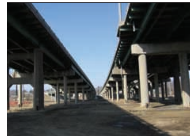
Figure 1.11 - Mainline/Underpass Bridge, Moline
