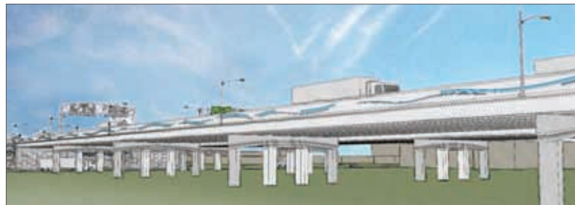
Figure 3.6 – Pier Concept at Mainline Bridge Viaduct
