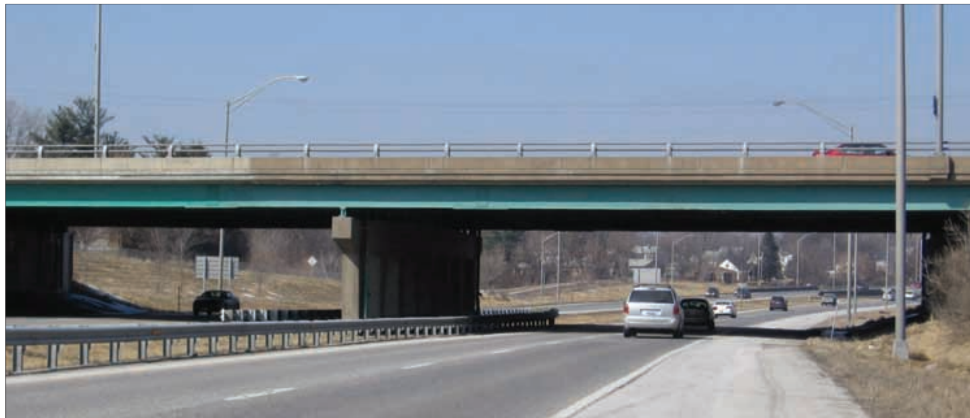
Figure 1.10 - Overpass Bridge at the Avenue of the Cities, Moline
