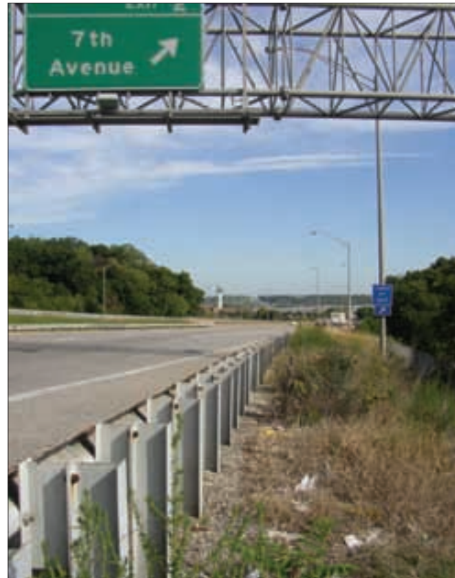
Figure 1.14 - Example of Barriers and Sign Truss
