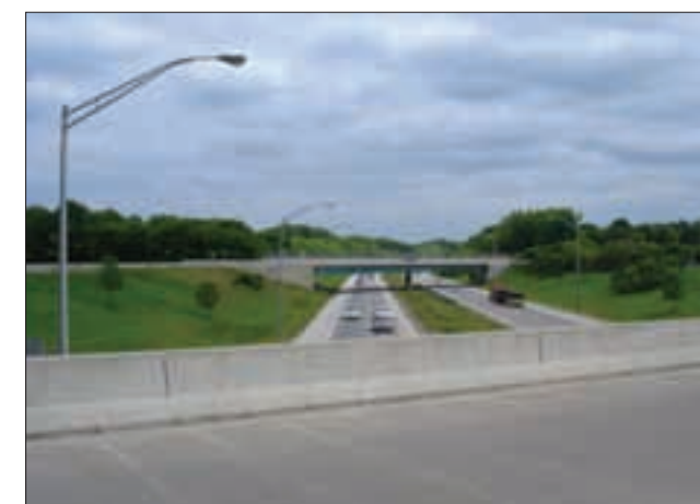
Figure 1.13 - Overpass Bridge at 27th St., Moline
