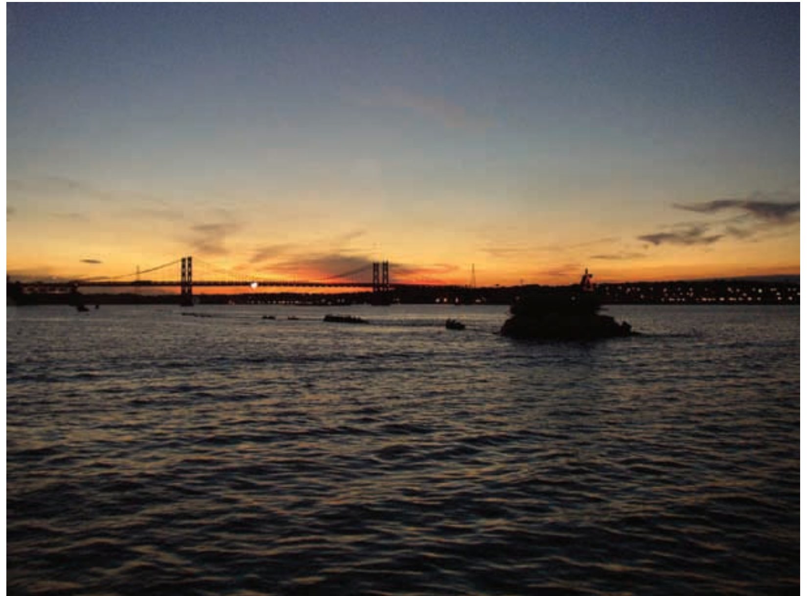
Figure 0.4 - Existing Memorial Bridge
