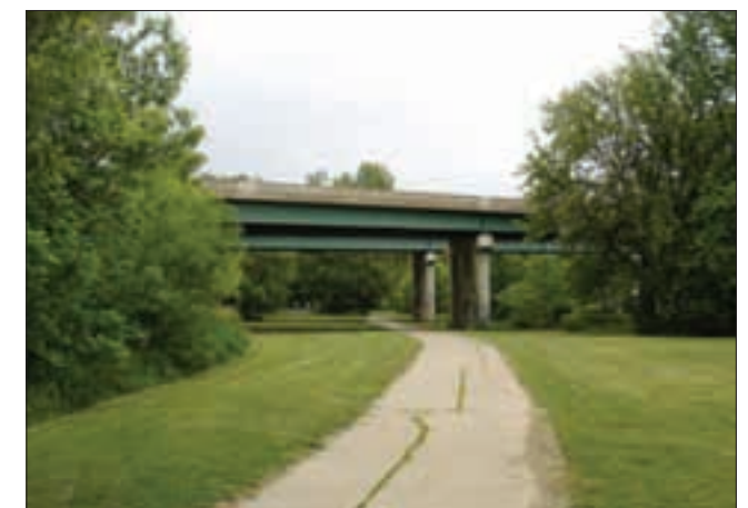
Figure 3.5 – Underpass Bridge to be Rebuilt, Duck Creek, Davenport
