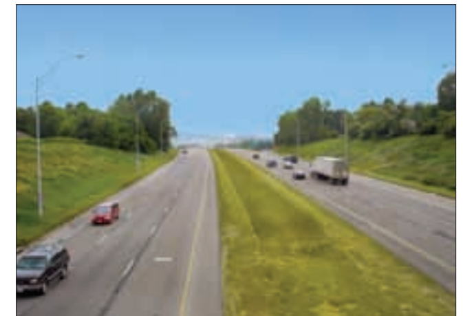
Figure 0.2 – Existing I-74 Corridor, South Bound Bettendorf
