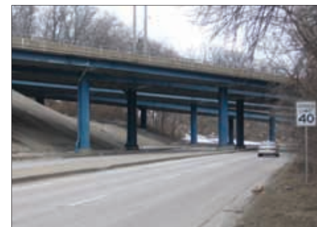
Figure 1.12 - Underpass Bridge at 19th St. & I-74, Moline
