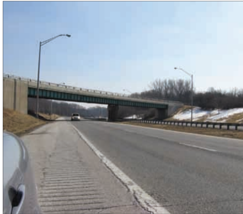
Figure 3.1 – Example of Existing Bridge to Remain, 27th St., Moline
