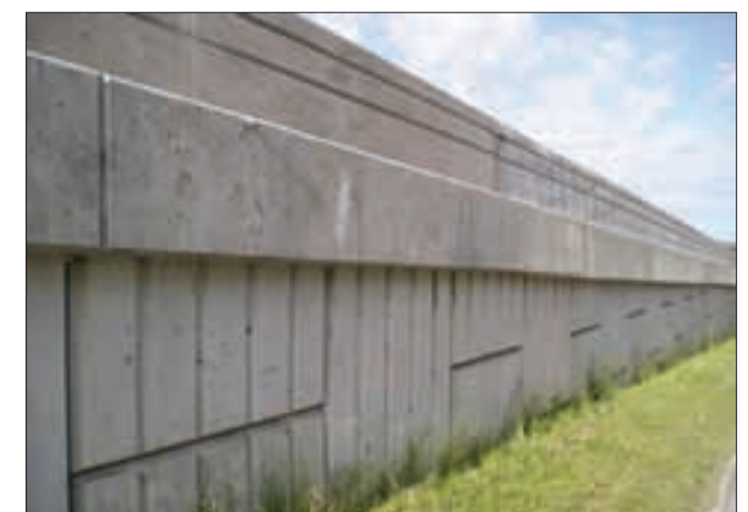
Figure 1.18 - Example of Retaining Walls
