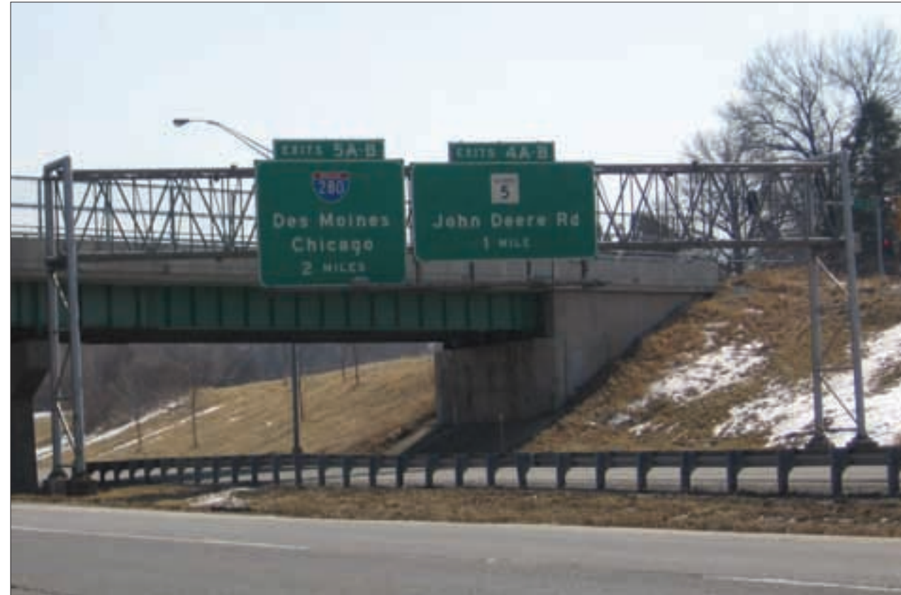
Figure 1.15 - Example of Sign Truss
