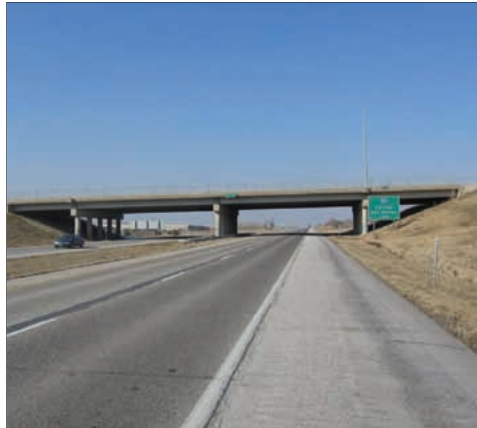
Figure 3.2 – Existing Bridge to be Widened or Rebuilt, E. 53rd St., Davenport
