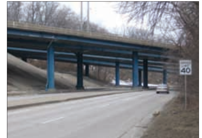
Figure 3.3– Example of Mainline/Underpass Bridge to be Rebuilt 19th St. & I-74, Moline
