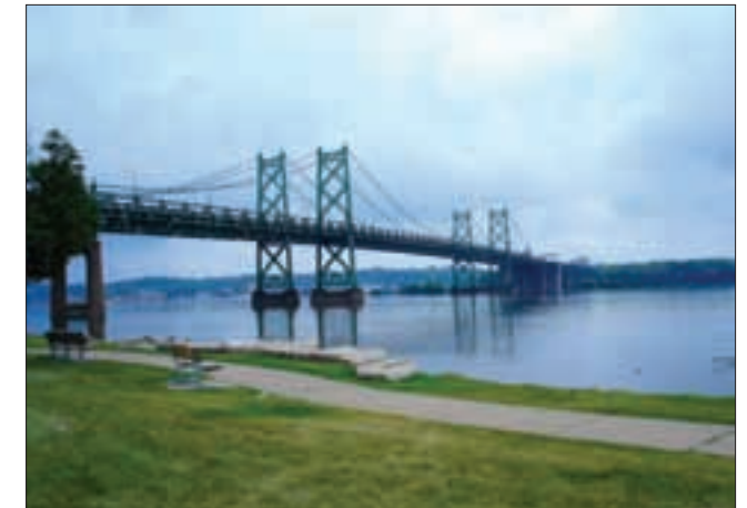
Figure 0.1 – Existing Memorial Bridge
