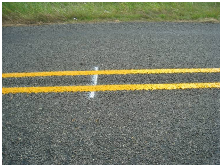
Figure 10. FM 1680 Road Surface with Marking.
