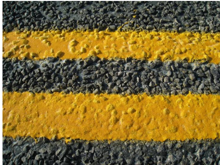
Figure 11. SH 85 Road Surface with Marking.
