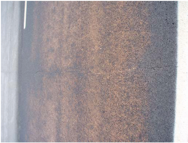
Figure 3.5 Close-up of a Cured Rejuvenating Seal on US-40 (Courtesy of Jusang Lee, INDOT)
