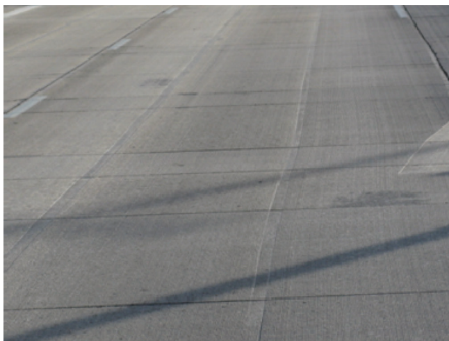
Figure 7.1 Continuous Grinding on US-50
