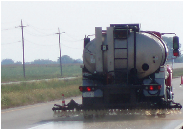
Figure 3.2 Application of Rejuvenating Seal on US-40 (Courtesy of Jusang Lee, INDOT)
