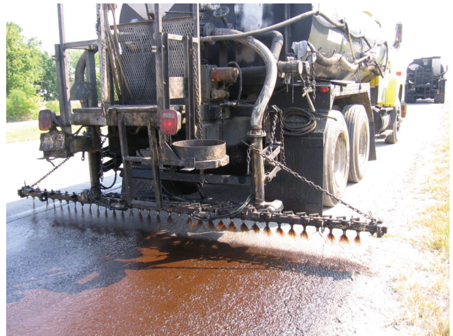
Figure 3.1 Application of Fog Seal on US-36
