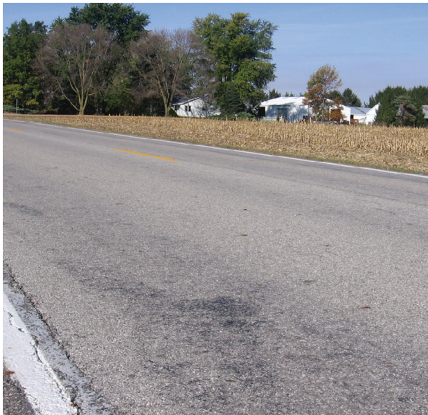
Figure 2.1 Photo of a Typical Single Chip Seal Pavement after 36 Months of Service
