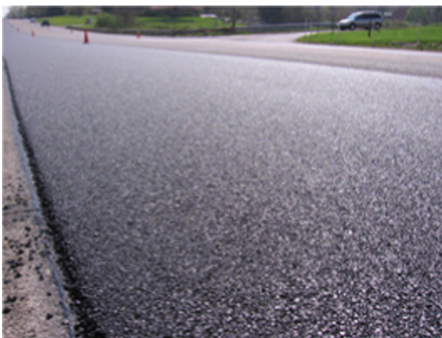
Figure 5.1 Photo of a Freshly Placed UBWC
