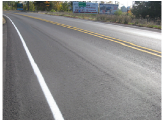
Figure 4.2 Photo of a Fresh Microsurfacing Pavement
