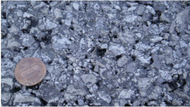
Figure 5.4 Close-up of Polished UBWC Surface on SR-114
