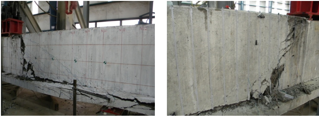
Figure 6.8: Specimen IT.7.22.6.FT/FTG at failure
