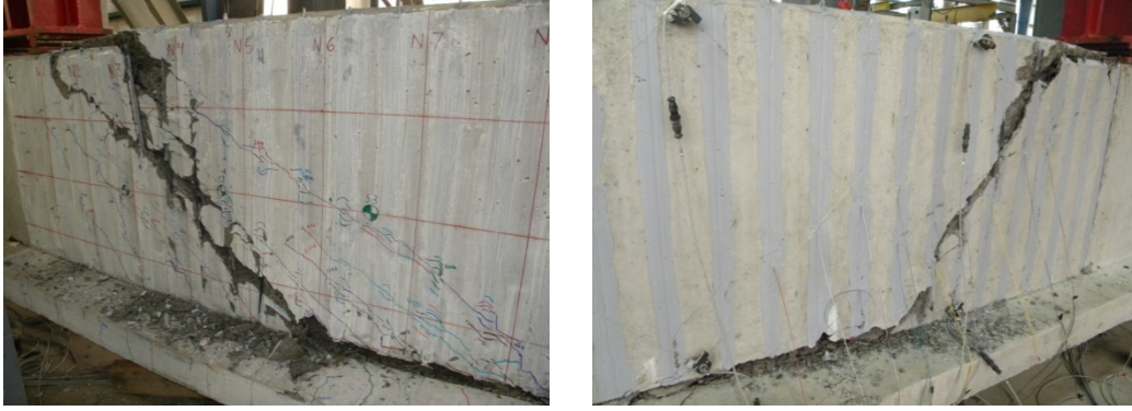
Figure 6.7: Specimen IT.7.22.6.FTG at failure
