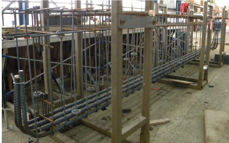
Figure 5.13: Example of reinforcing cage (T specimen shown)
