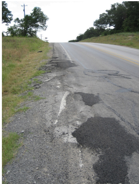
Figure 43. Shoulder Patches near County Road Intersection (FM 2257, Fort Worth District).
