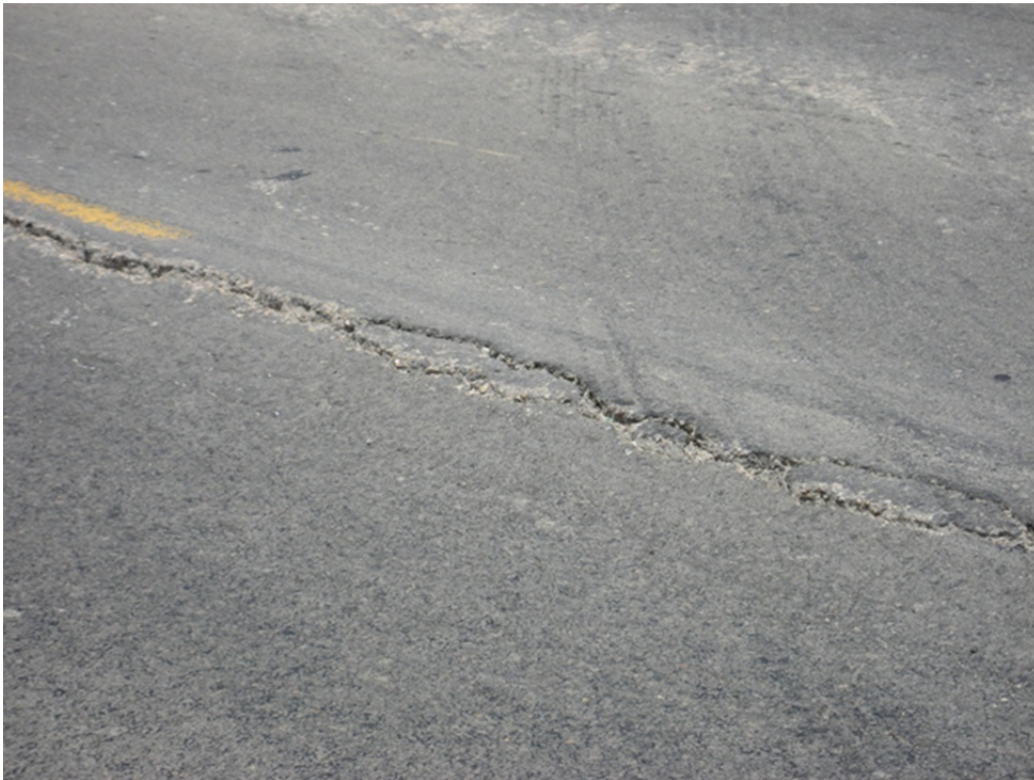
Figure 47. Shoulder Patch (IH 35W – Frontage, Fort Worth District).
