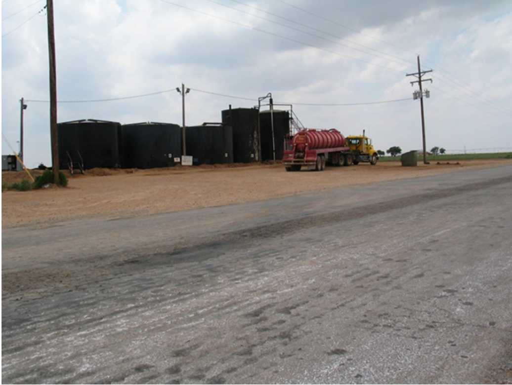
Figure 20. Well Fluid Station (FM 1585, Lubbock District).
