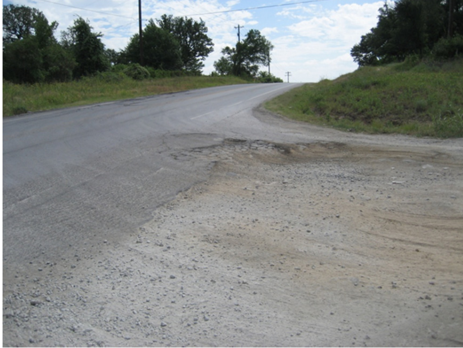
Figure 42. County Road next to Saltwater Disposal Facility (FM 2257, Fort Worth District).
