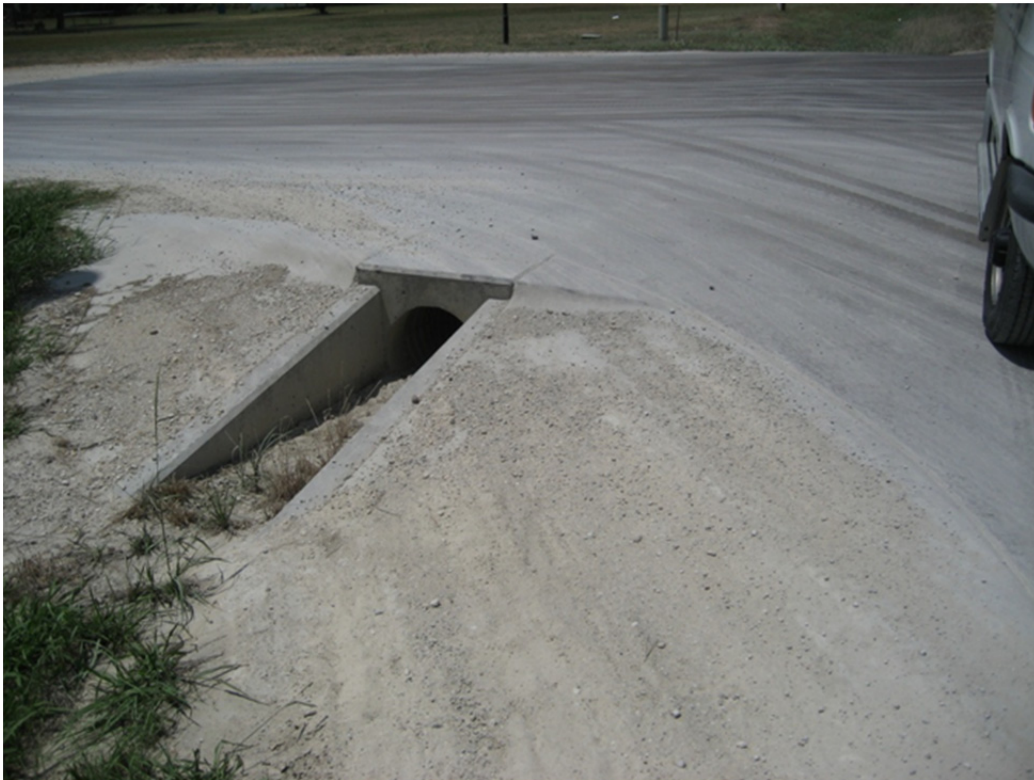
Figure 51. Tire Tracks, Safety End Treatment (IH 35W – Frontage, Fort Worth District).
