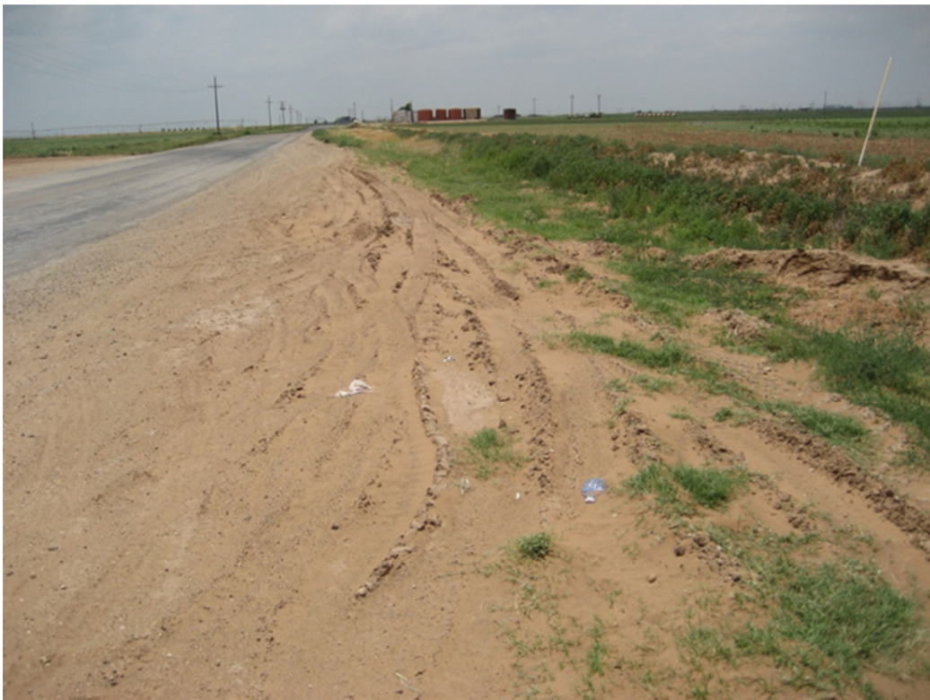
Figure 23. Tire Tracks on Unpaved Shoulder (FM 1585, Lubbock District).
