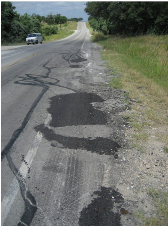
Figure 43. Shoulder Patches near County Road Intersection (FM 2257, Fort Worth District).
