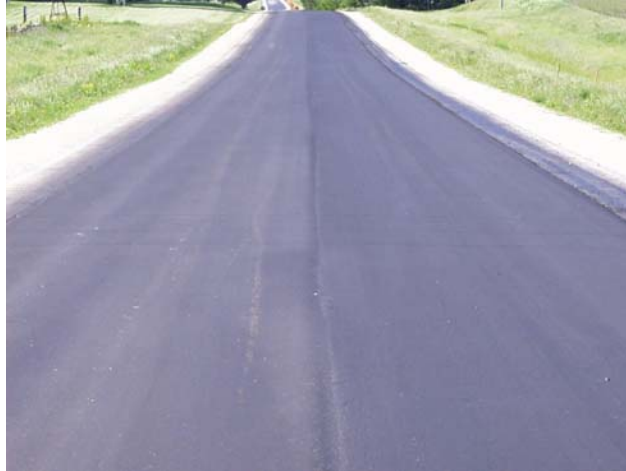
Figure 7. HMA stress relief layer
