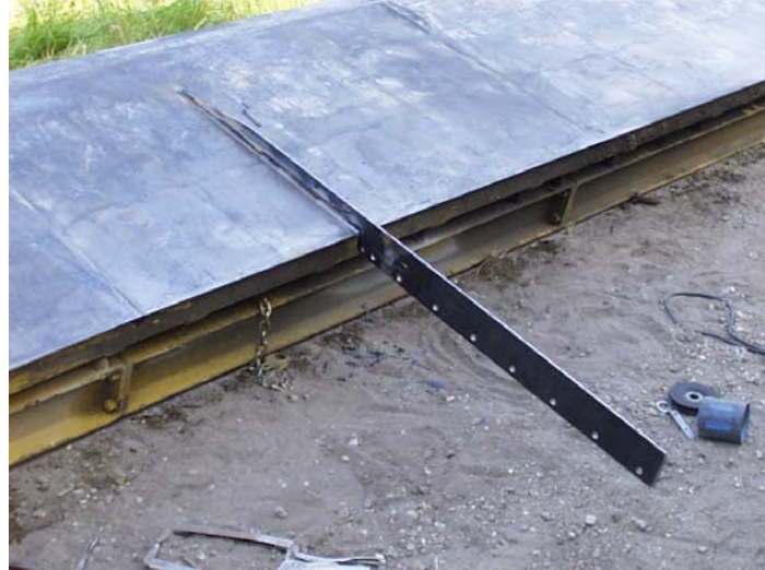
Figure 11. Longitudinal joint-forming knife
