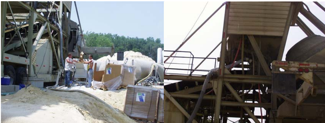
Figure 13. Fibers being blown into the concrete mixing drum
