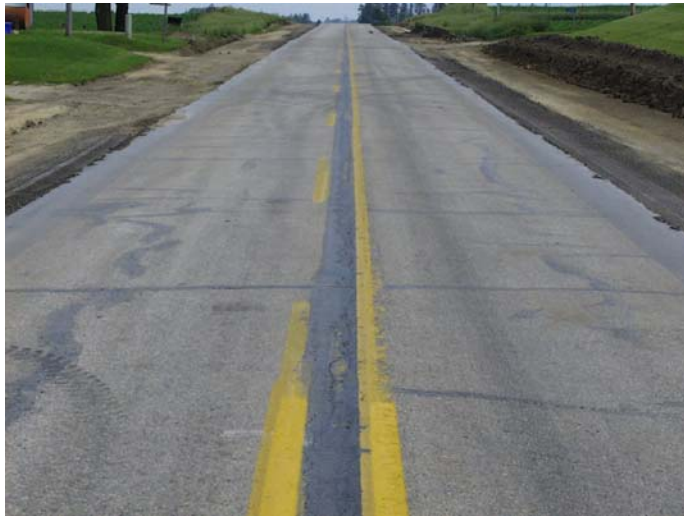
Figure 6. Completed widening unit milling operation
