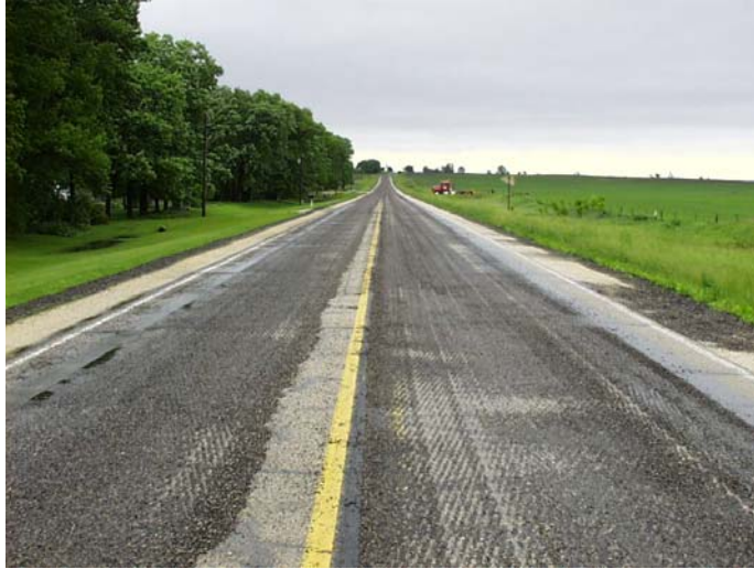
Figure 5. Scarified pavement surface
