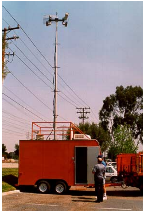
Figure 3-3. Trailer operational at Cerritos Avenue and Sunkist Street
