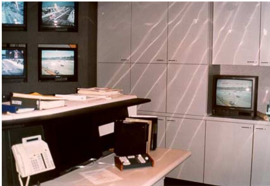
Figure 3-5. Anaheim TMC work area
