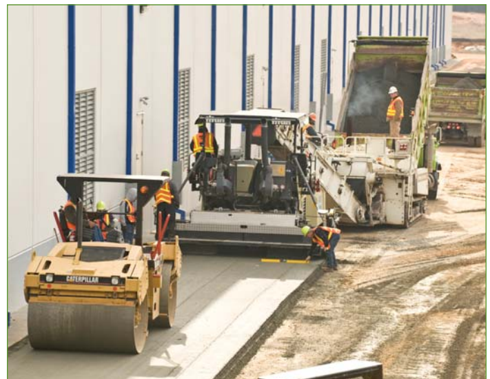
RCC paving train
