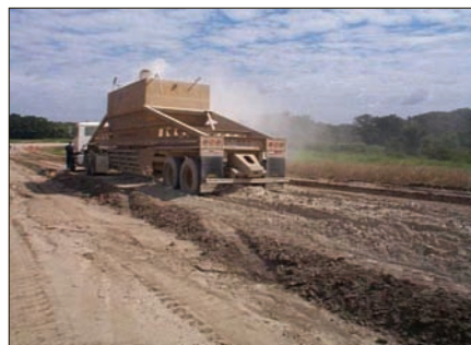
Fly ash can be used as a soil-stabilizing additive.
