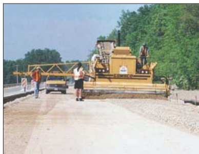
Trimming a granular subbase
