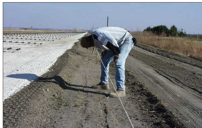
Eyeball the stringline for alignment.
