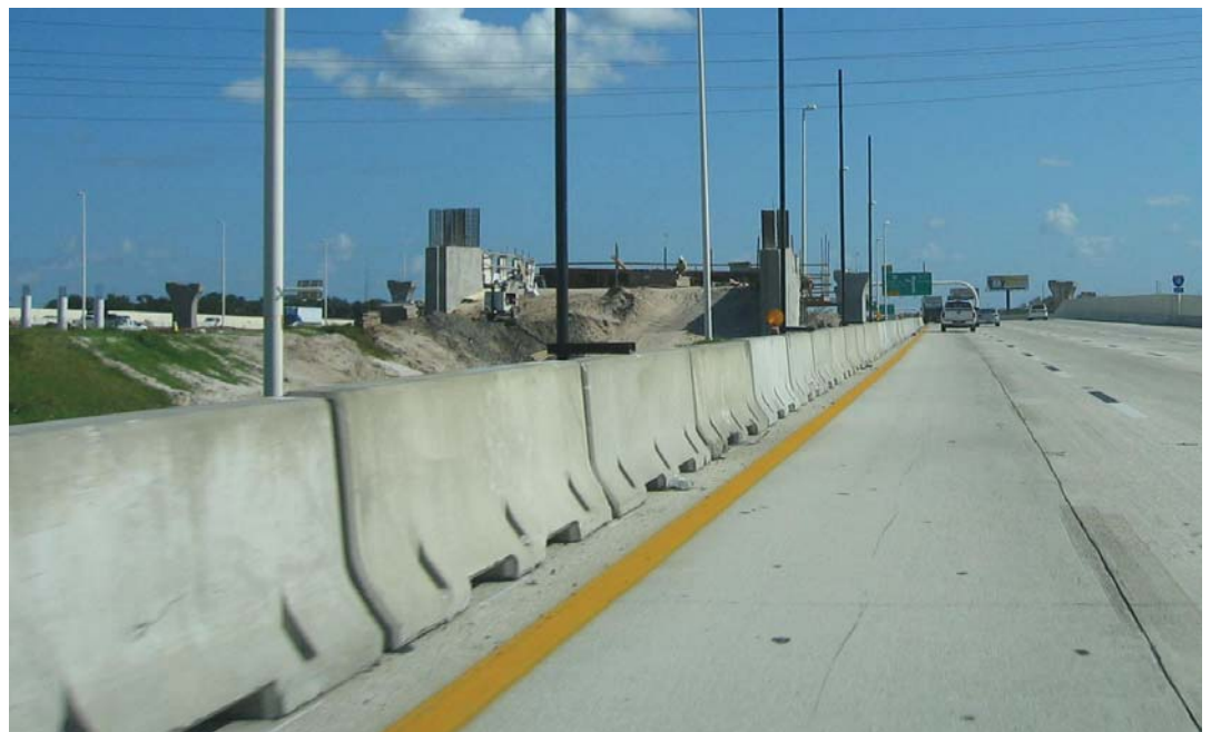
Eastbound I-4 at the CSX Railroad overpass. The contractor for the I-4 to Selman Expressway expansion project used K-barriers along the length of the five-mile project. Bolting the barriers to concrete reduces the distance barriers deflect if struck by an errant vehicle and reduces the size of the deflection zone required in work zones.
