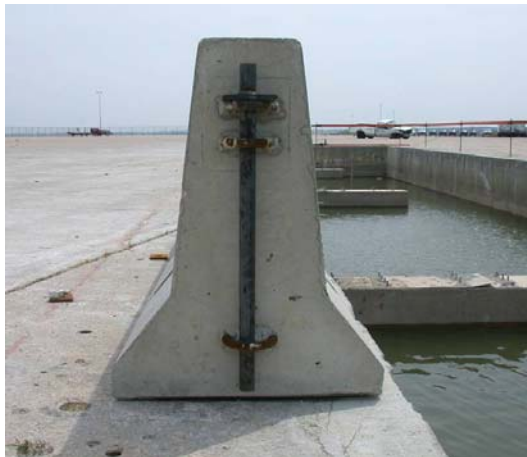
Below: End view of a K-barrier depicting a pin and loop end connection. Typically, safety barriers are attached end-to-end by a load-bearing connection that keeps the barriers joined and helps to stop a vehicle upon impact.
