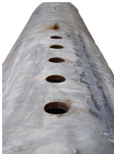
Figure 6-5. Longitudinal seam weld placed to the right of through-bolt holes. Photo courtesy of S. Dalton.
