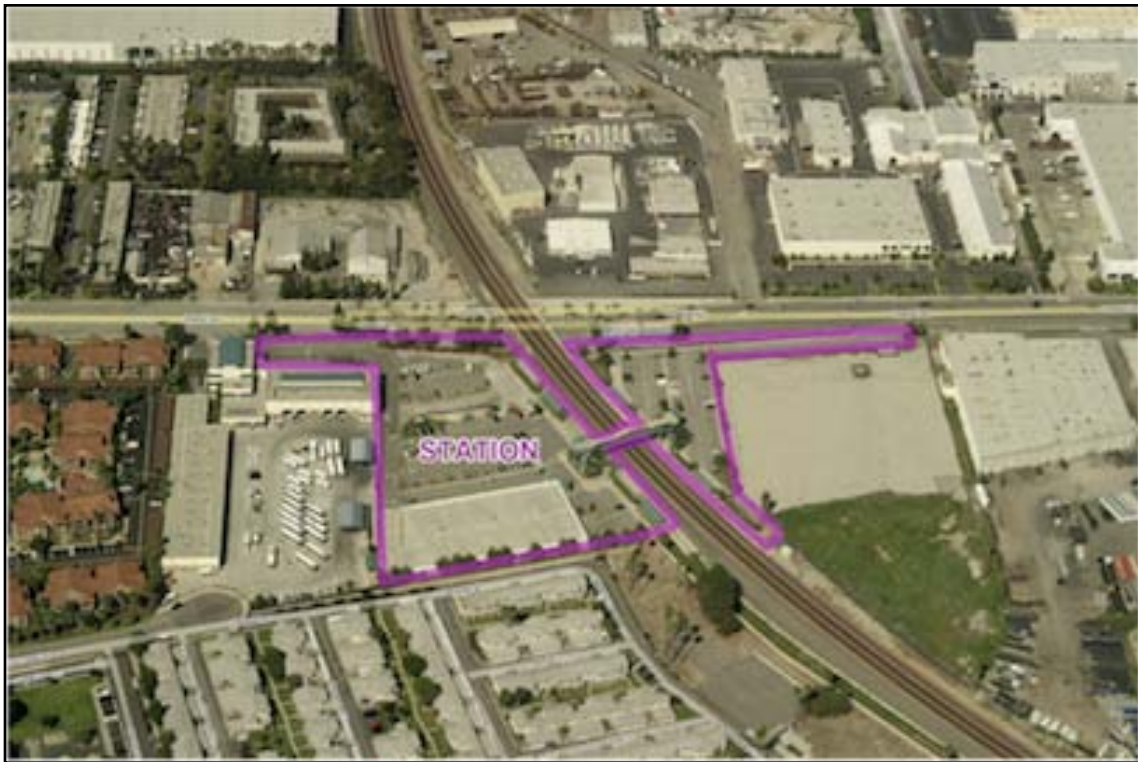
Figure 36. Industrial Land Uses near the Norwalk Tracks
