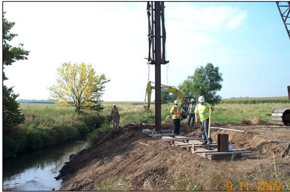
c. Pile driving in west abutment
