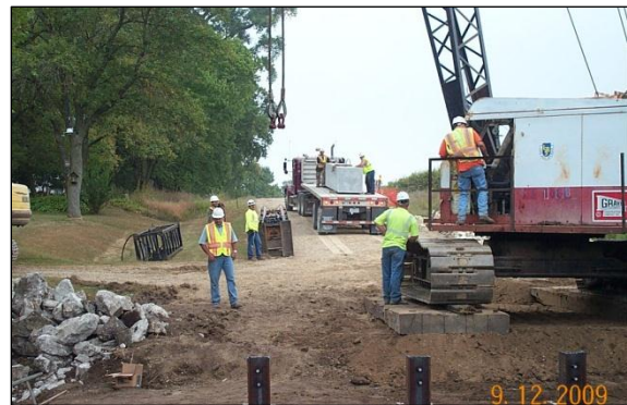
f. East abutment cap arriving at site
