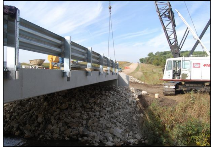
f. Completing north guardrail
