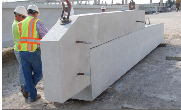
Figure 2.15. Precast backwall and abutment
