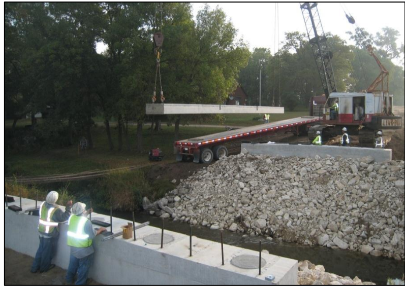
b. Unloading of Beam #4
