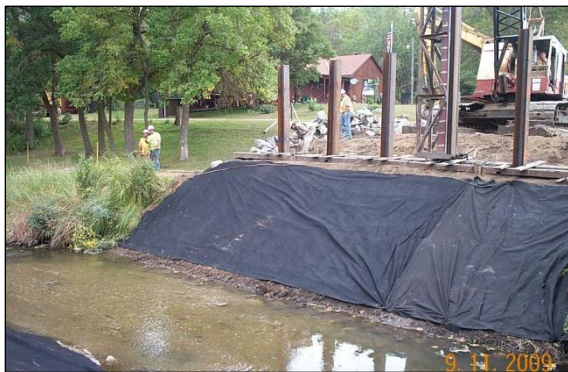
e. Driving piling in east abutment
