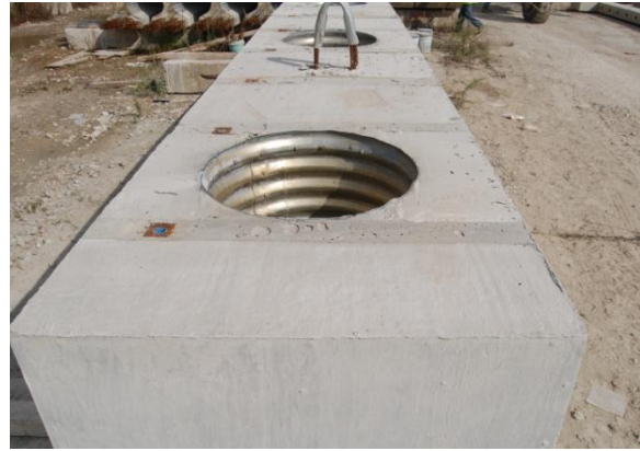
b.) Precast abutment pile connection openings
