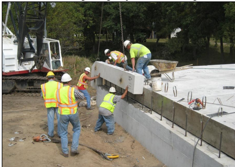
c. Placement of a backwall segment
