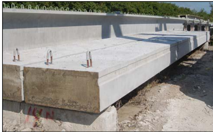
Figure 2.14. Voided precast beams
