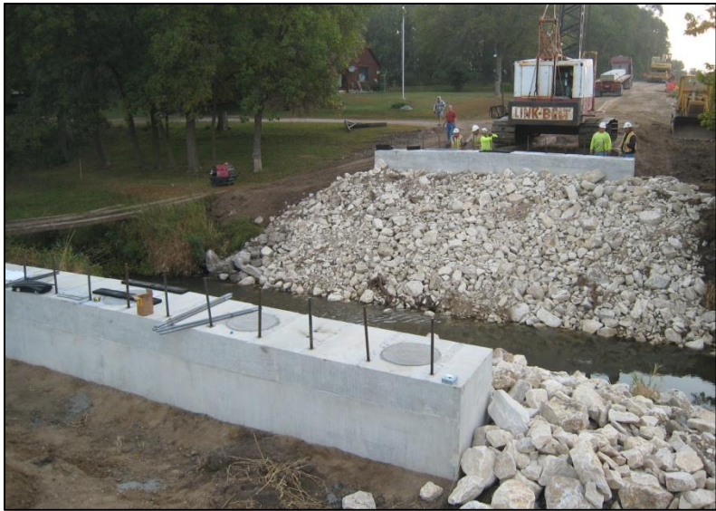
a. Both abutments in place
