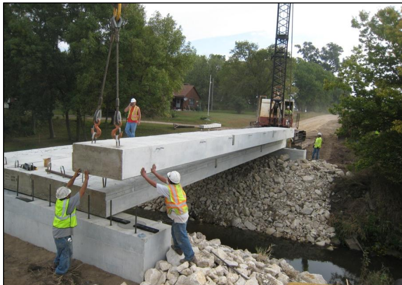
g. Positioning of exterior Beam #7
