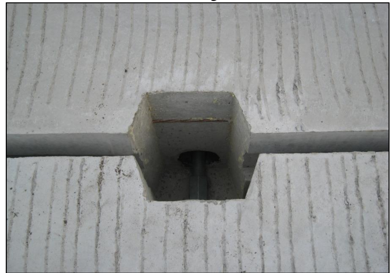
h. Tie rod block out
