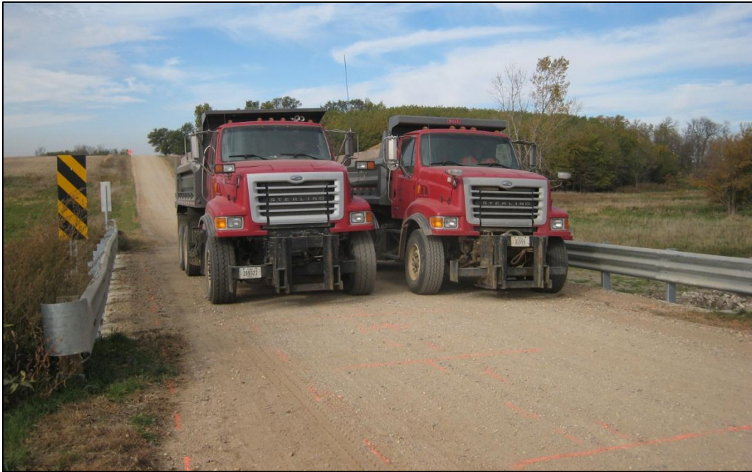
Figure 3.5. Trucks on bridge during 2010 LC7 test
