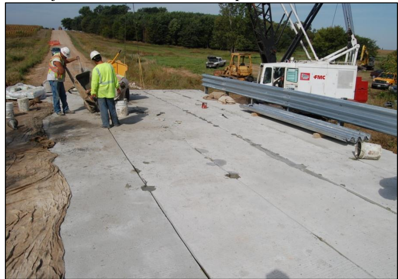
l. Placement of non-shrink grout
