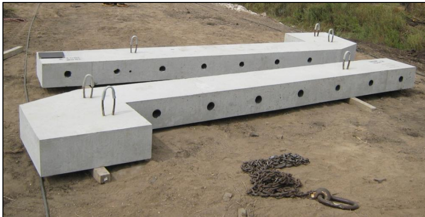
c. Wing wall segments
