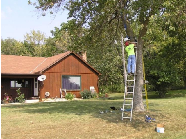
a. Camera installation
