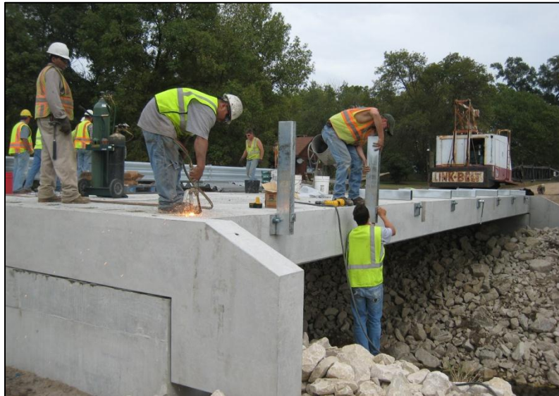
g. Installation of guardrail post on south side of bridge
