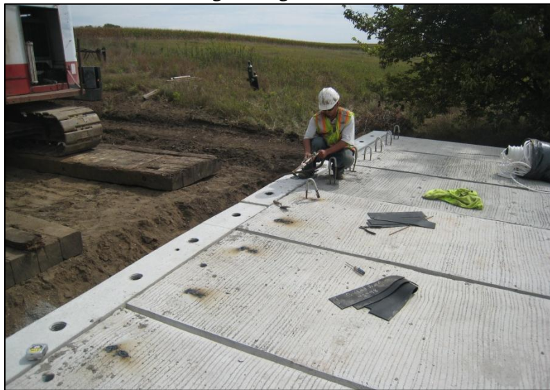
k. Cutting off beam lift cables
