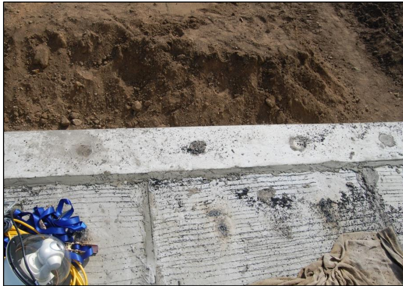
e. Grouting of various voids and joints
