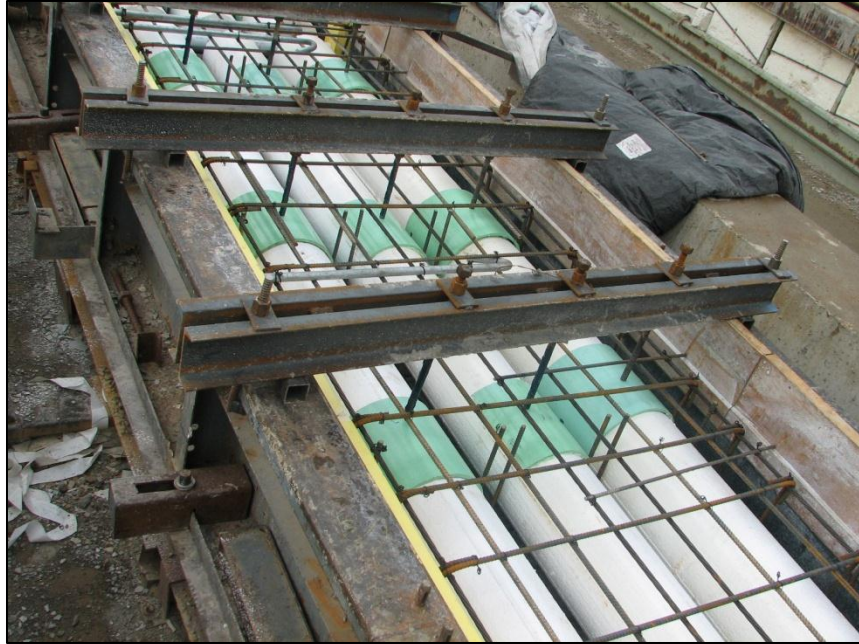
a. Overall view
