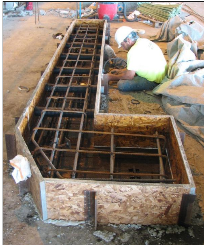
Figure 2.11. Backwall formwork
