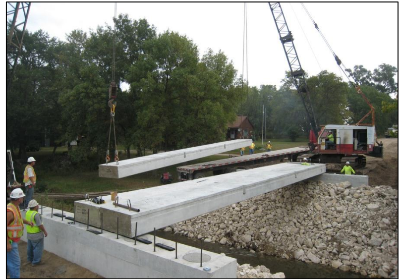
f. Positioning of Beam #3
