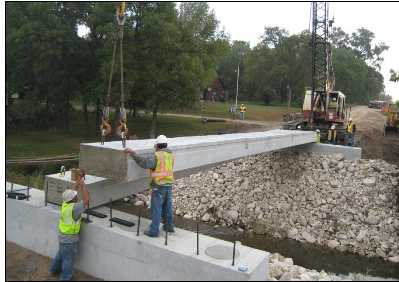
d. Setting of Beam #5
