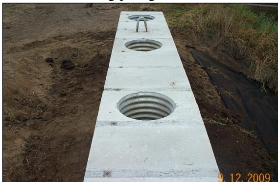
g. East abutment cap in place
