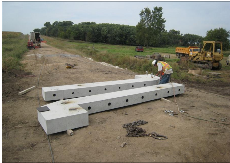
a. Removing lifting loops on backwall segments
