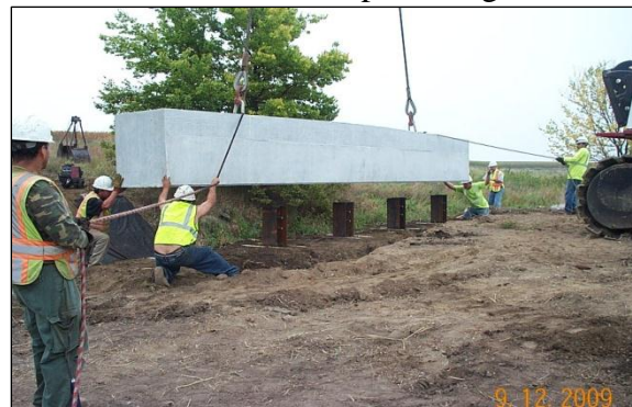
h. Installing west abutment cap
