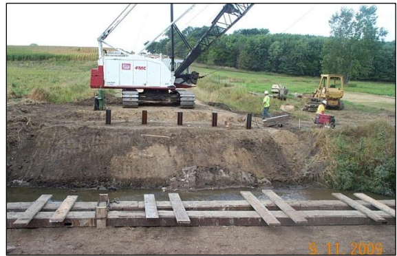
d. Piling completed in west abutment
