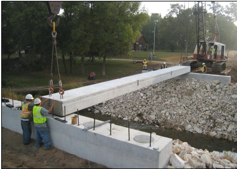
c. Positioning of Beam #4
