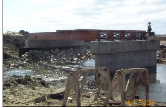
b. Erection of south span girders
