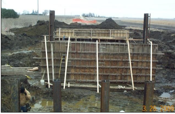
a. Construction of abutments and pier
