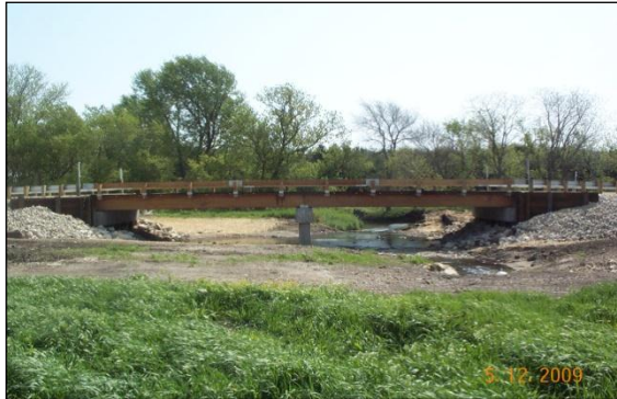
h. Completed demonstration bridge
