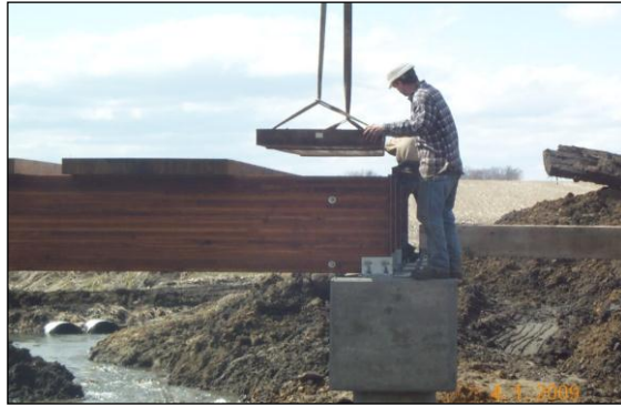
c. Deck panel placement
