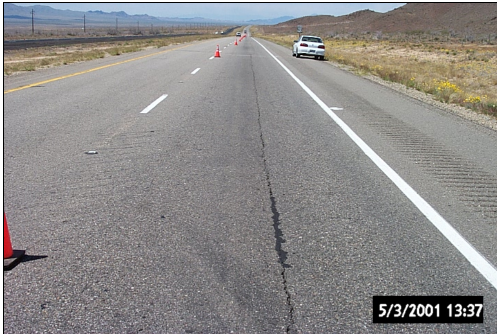
Figure 10. Photograph of paving seam.
