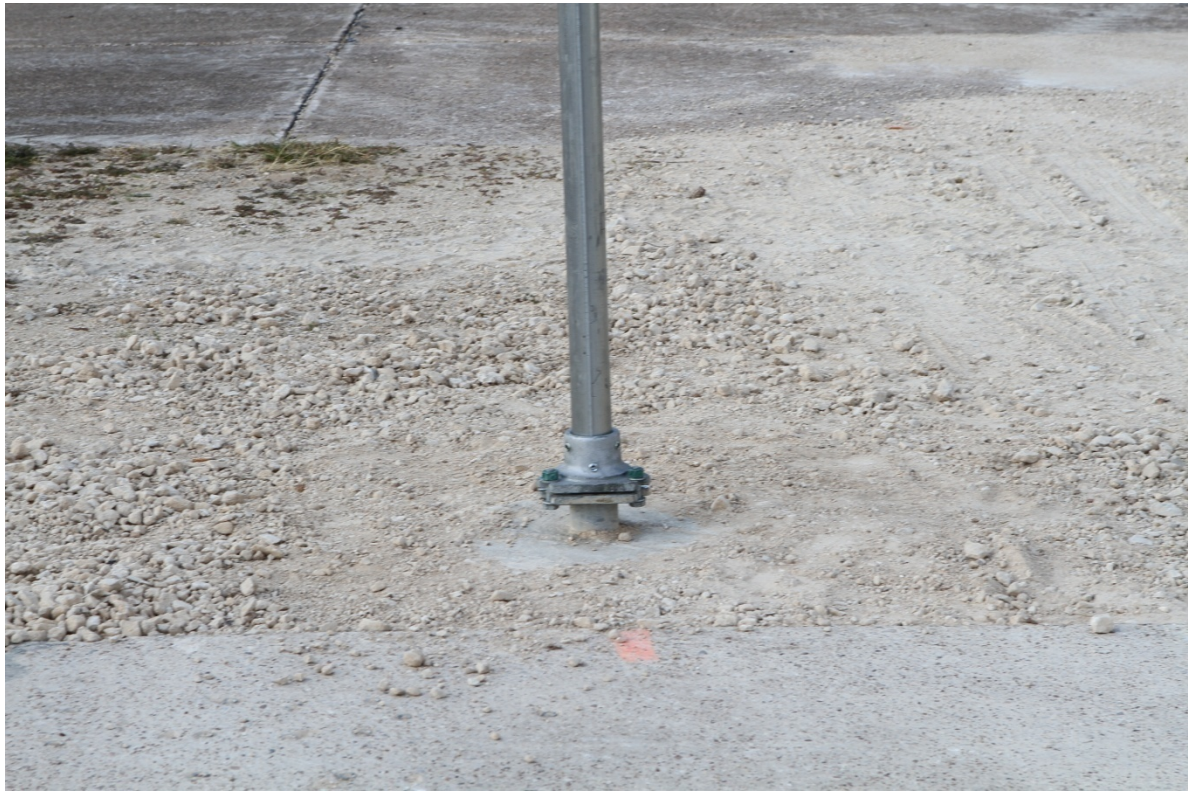
Figure 9.30. Sign Support System prior to Test Nos. 463631-1 and 2.
