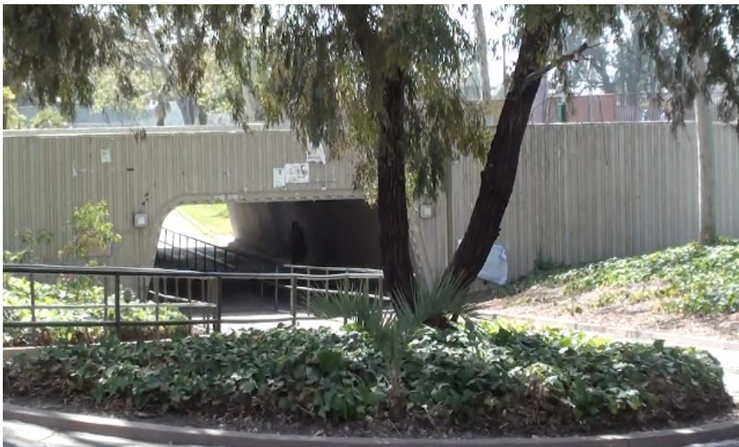
Figure 46. Underpass for Bicycle Path #1 – Santa Barbara, California
