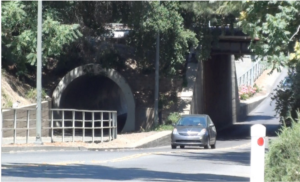
Figure 45. Bicycle Underpass – Davis, California
