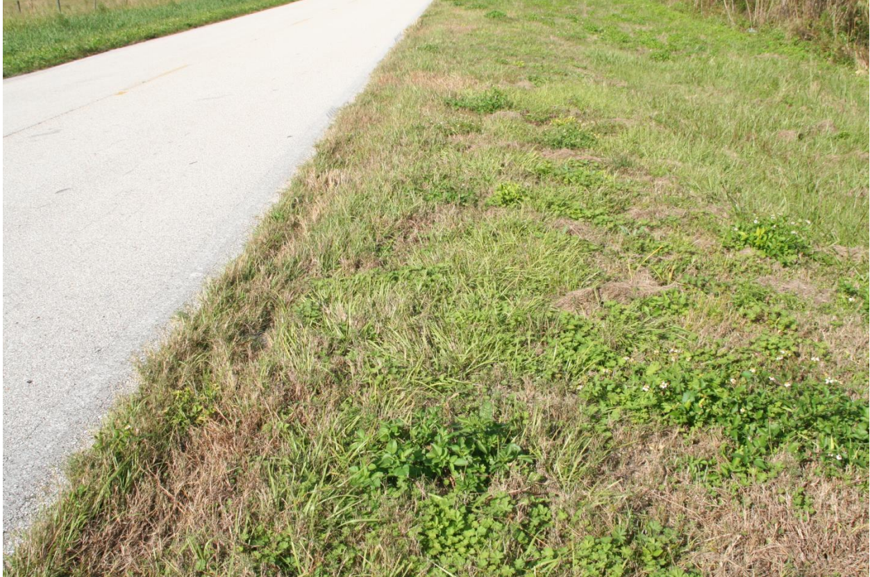
Image 3. Roadside at conclusion of project. Hardee County.
