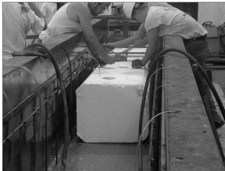
Figure 5-7 Expanded polystyrene void forms are placed in the casting bed during casting of box beams.
