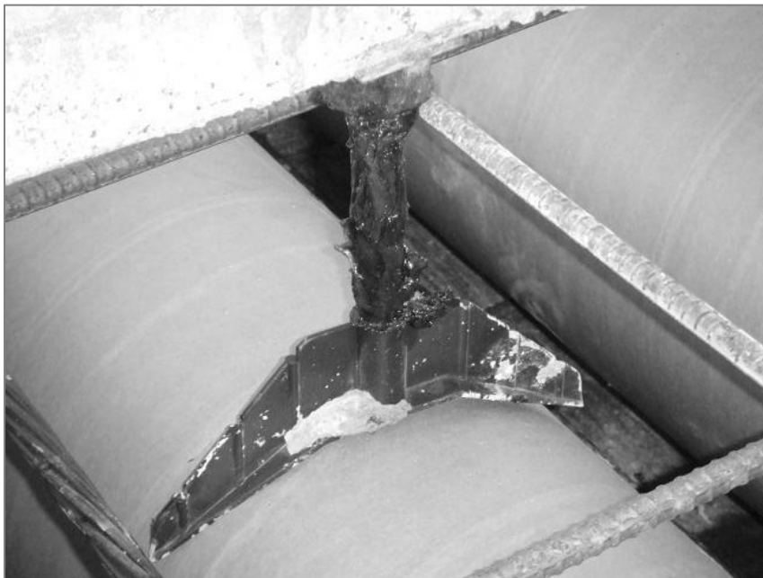
Figure 5-11 A molded plastic device is used to contact the void tube in the external hold-down system.
