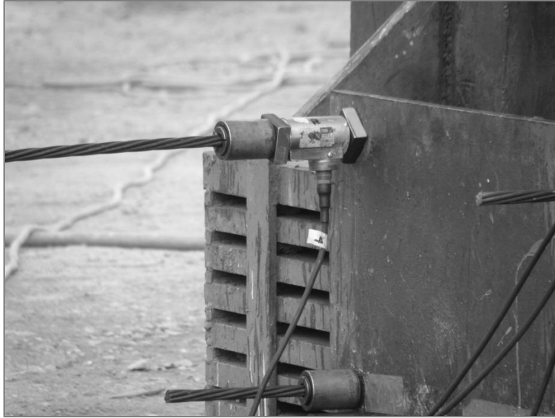
Figure 4-3 Load cells placed on selected strands to measure the prestressing force.
