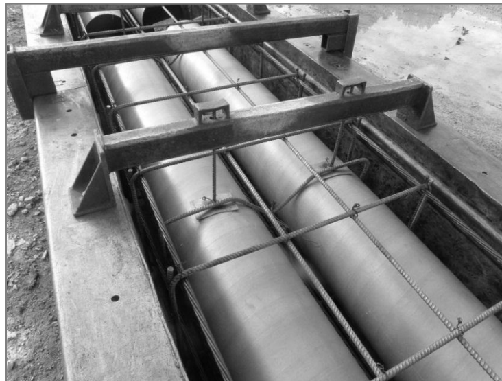
Figure 5-9 Paper tubes have been placed in the casting bed to form the internal voids of cored slabs. The tubes are held in place with an external hold-down system.
