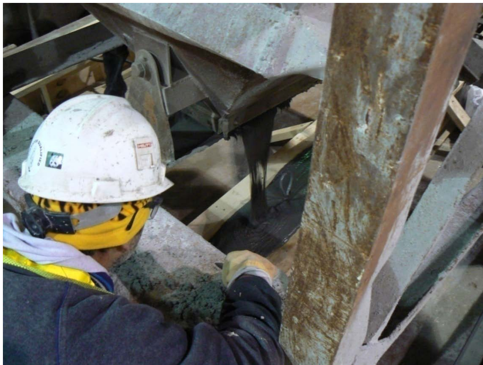
Figure 4.18. Beginning of first pour of UHPC units
