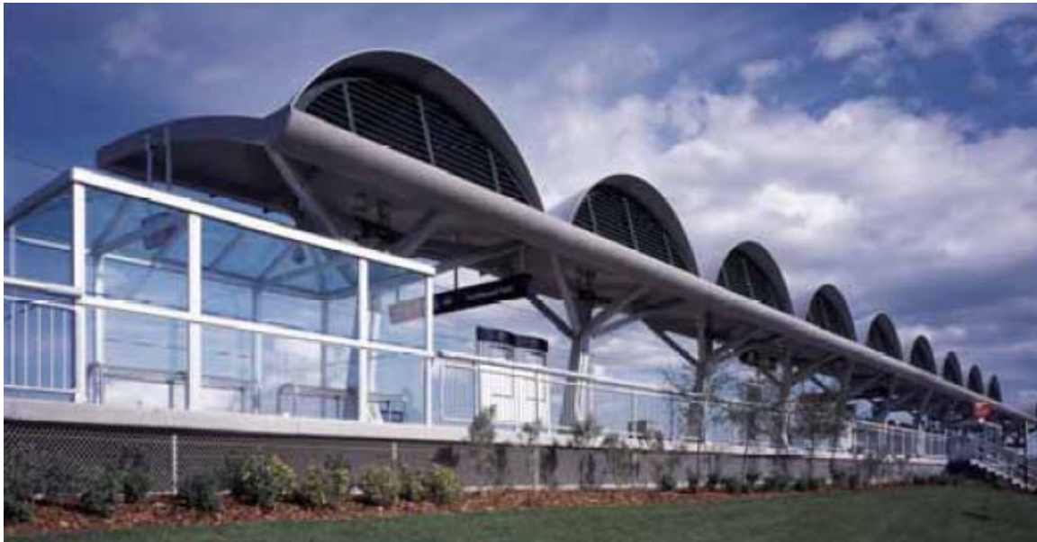
Figure 2.34. Shawnessy LRT station with UHPC canopies (Perry 2006)
