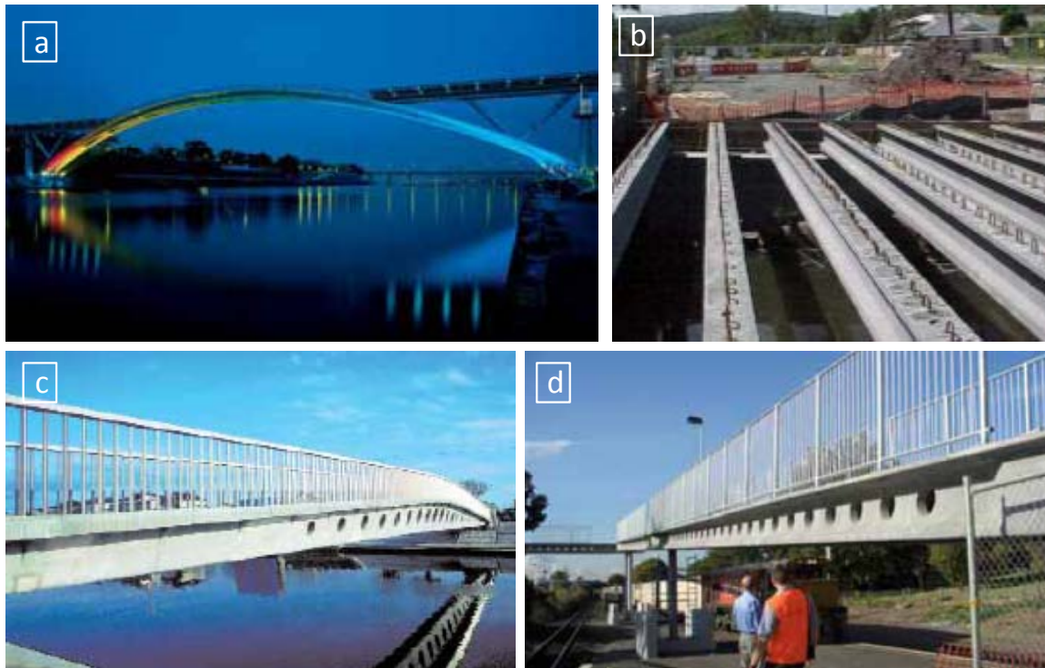
Figure 2.33. Examples of UHPC bridges and footbridges: a) Footbridge of Peace in South Korea, b) Shepherd Creek Road Bridge in Australia, c) Sakata Mirai footbridge in Japan, and d) Papatoetoe footbridge in New Zealand (Perry 2006, Lafarge 2007, Billon 2006)
