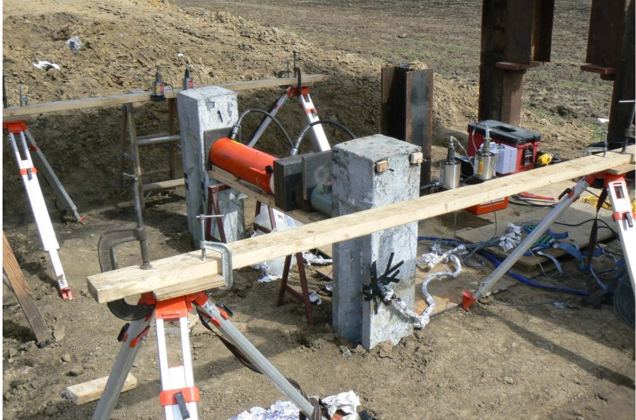
Figure 5.33. Overall layout at beginning of lateral load test on UHPC piles
