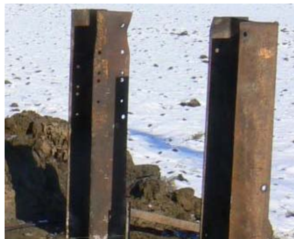
Figure 5.8. Local buckling and bending damage to two steel anchor piles due to driving
