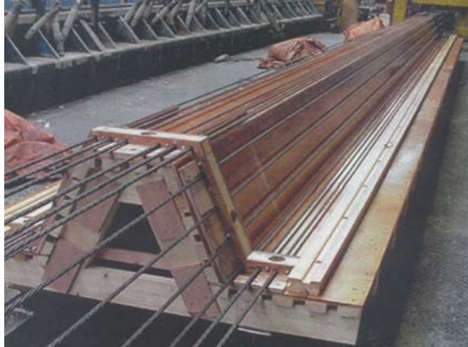
Figure 2.42. Prestressing strands and formwork used for production of SCFRC sheet piles (Walraven 2007)
