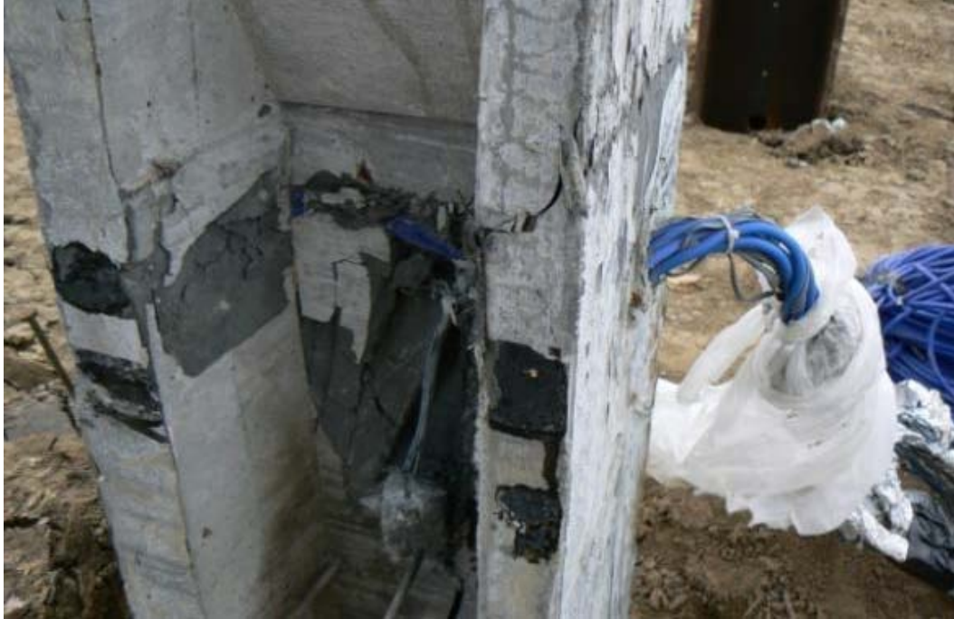
Figure 5.48. Bundle of instrumentation wires passing through the web and out of the flange of UHPC pile P1
