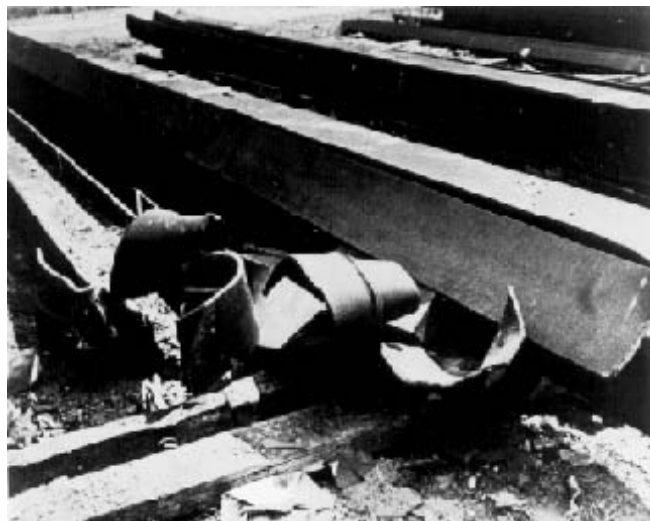
Figure 1.5. Steel piles heavily damaged due to hard driving (DiMillio 1998)
