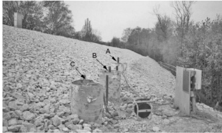
Figure 5-1. Instrumented section of embankment at Hildenborough after berm had been regraded to create a two-stage slope (Smethurst and Powerie 2007)
