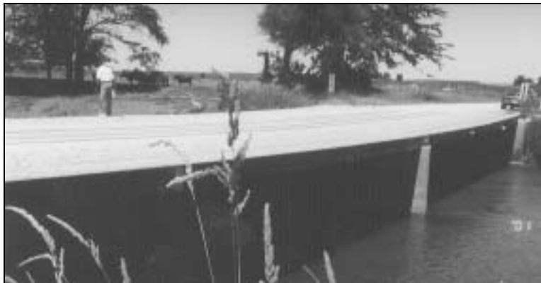
Low Water Bridge
