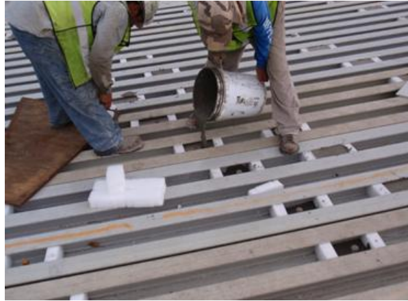
Figure 14 – Grout pockets being poured at each stud
