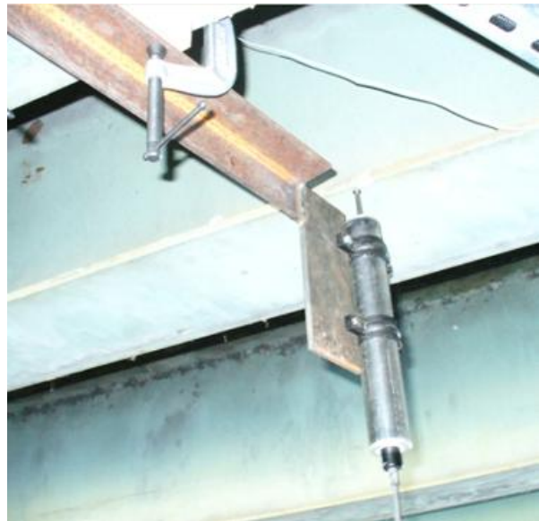
Figure 29 – Deflection gage on steel girder
