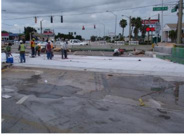
Figure 17 – Placement of polymer concrete wearing surface
