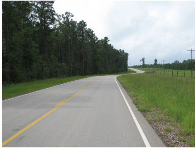
Figure 66. Two-Lane Roadway with Narrow Shoulder.
