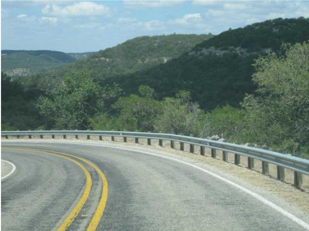
Figure 17. RM 337 -- Typical Road Studied in San Angelo District.
