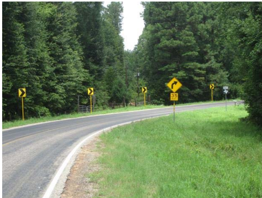
Figure 54. Example of Chevrons on a Two-Lane Road.
