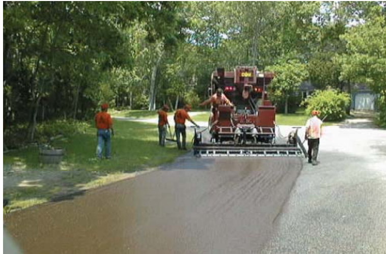
Figure 64. Application of Skid-Resistant Pavement Surface in Curve (FHWA, 2006).
