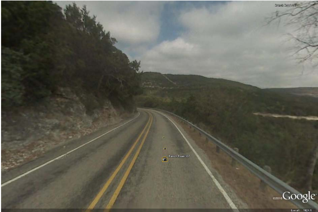
Figure 12. Example of Sideslope Rating 5. (Image Credit: Google Earth™ Mapping Service, Street View)
