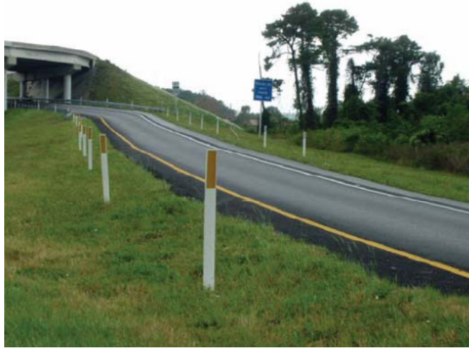
Figure 55. Post Delineators Installed on a Ramp (FHWA, 2006).
