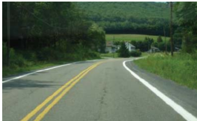
(b) Roadway with 8-inch edgeline.
