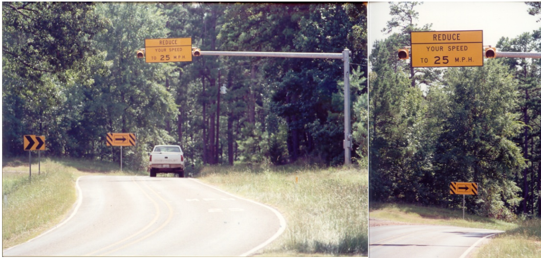
Figure 60. Dynamic Curve Speed Warning System in Camp County, Texas.
