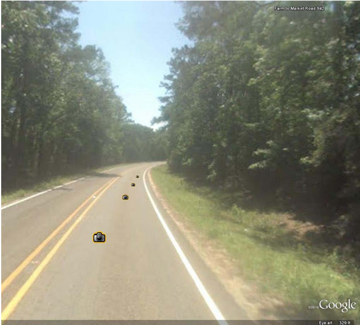
Figure 9. Example of Sideslope Rating 2. (Image Credit: Google Earth™ Mapping Service, Street View)
