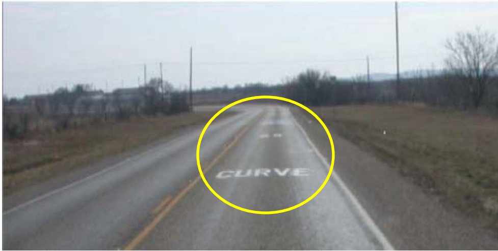
Figure 61. Speed Limit Advisory Pavement Marking (FHWA, 2006).
