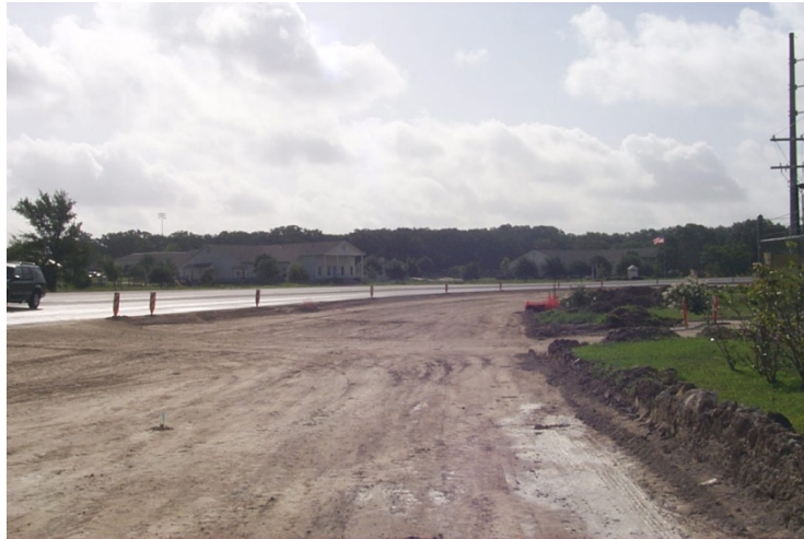
Figure 65. Lane Width Being Modified.
