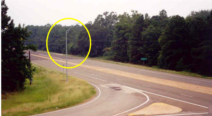
Figure 63. Safety Improvement by Adding Lighting.
