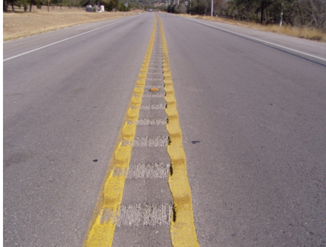
Figure 69. Illustration of Rumble Strip for Centerline.
