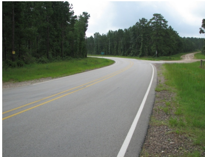
Figure 72. Driveway Intersecting a Rural Road in the Lufkin District.
