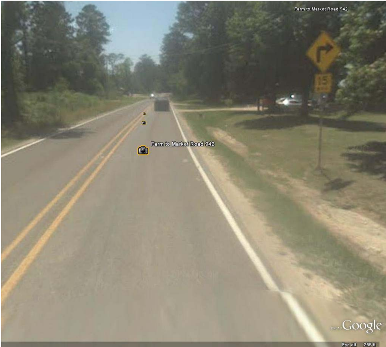
Figure 10. Example of Sideslope Rating 3. (Image Credit: Google Earth™ Mapping Service, Street View)
