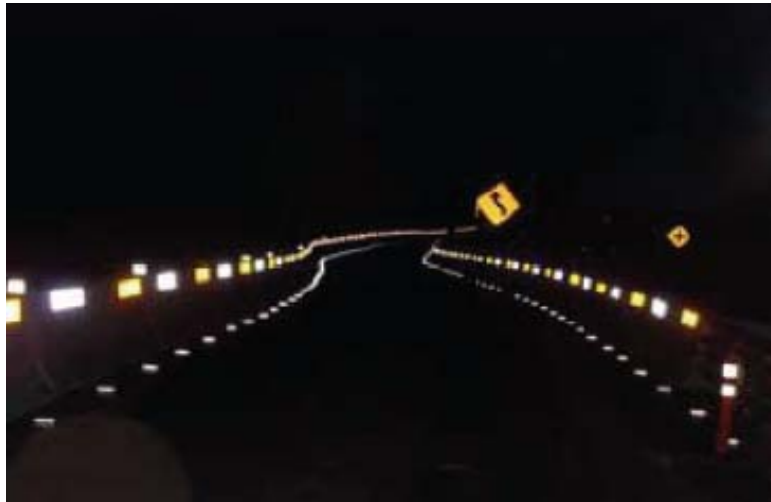
Figure 57. Example of Reflective Barrier Delineation (FHWA, 2006).
