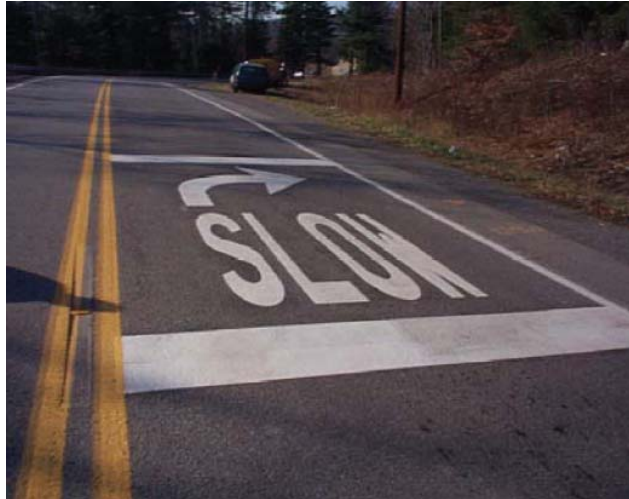
Figure 74. PennDOT Curve Advance Marking (FHWA, 2006).
