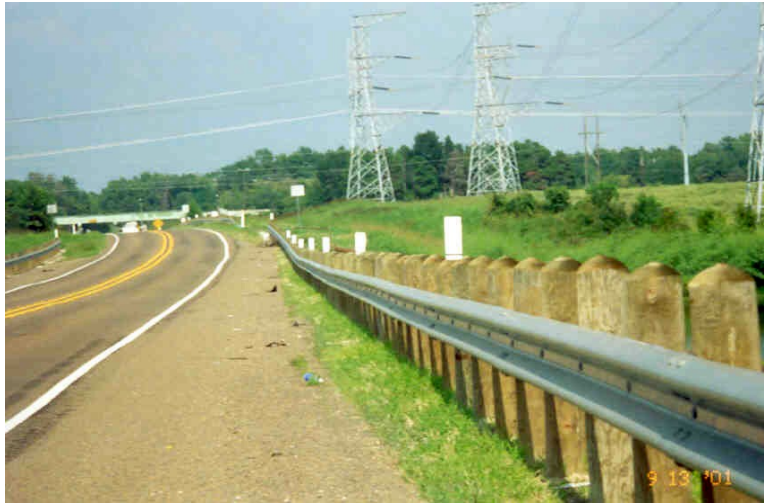
Figure 71. Guardrail Used as a Barrier and Shield.
