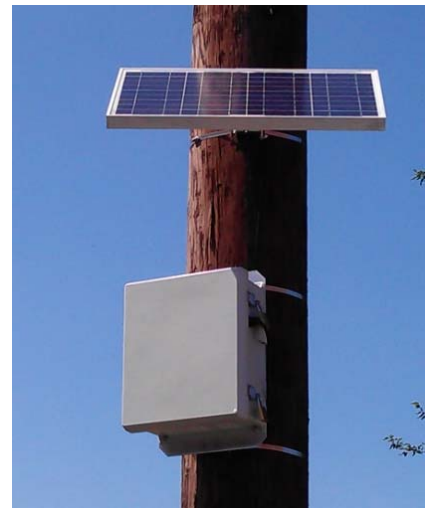
Figure 4 Sample Permanent Installation
