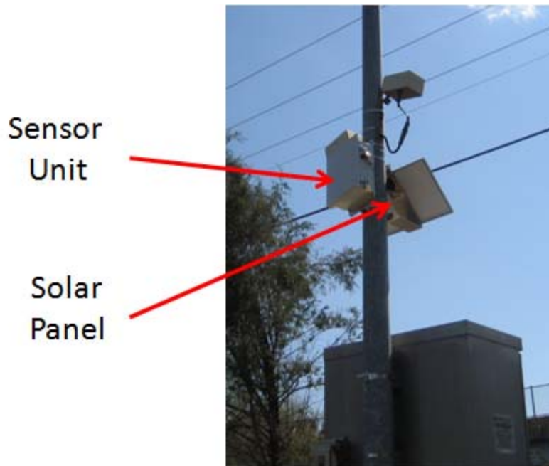
Figure 5 Actual Installation of BTM Unit
