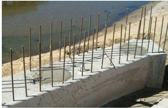
Figure 120. Finished specialty concrete in the east abutment, October 5
