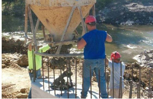
Figure 119. Concrete being placed in the east abutment, October 5
