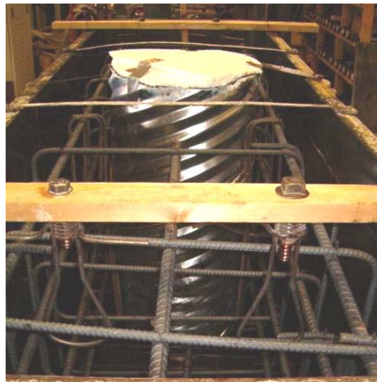
Figure 18. Lifting hooks and Styrofoam cover before placing concrete
