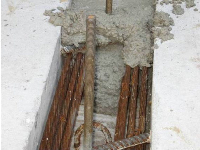
a) Concrete flowing in channel
