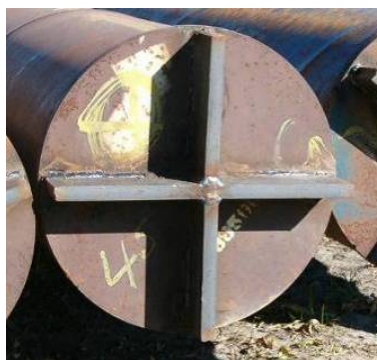
Figure 111. Steel pipe pile driving point, September 28
