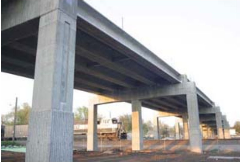
Figure 8. Bridge pier cap located Lincoln, Nebraska
