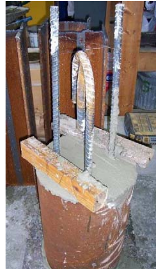
b) Pipe pile after placing concrete
