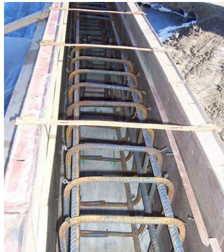
Figure 144. Barrier rail reinforcement, December 8
