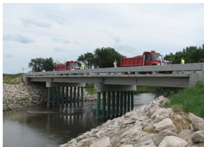
Figure 2.12 Static test (Load Case 2)
