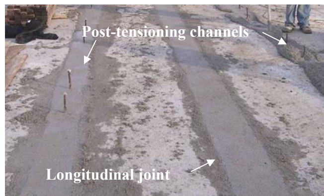
Figure 140. Longitudinal joint and one channel finished, November 28
