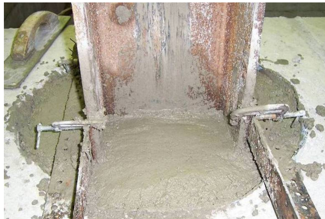
Figure 23. H-pile after being grouted in place
