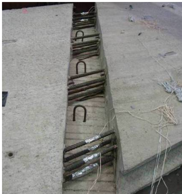
Figure 2.10. Reinforcing bars instrumented with steel strain gages
