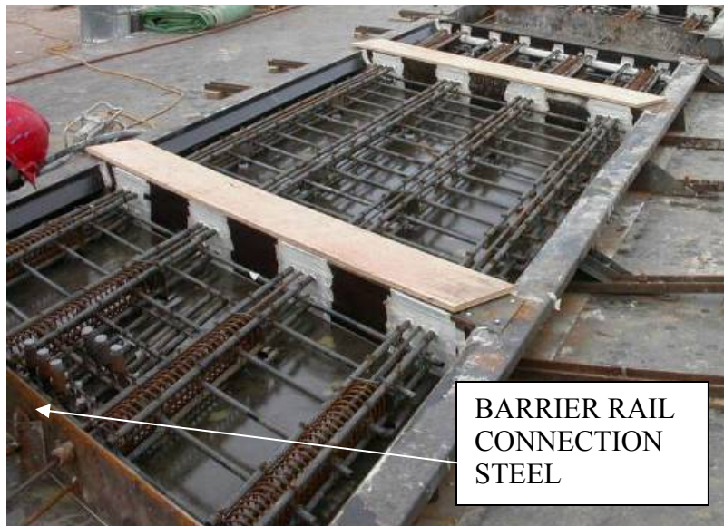
a) Deck panel reinforcing steel
