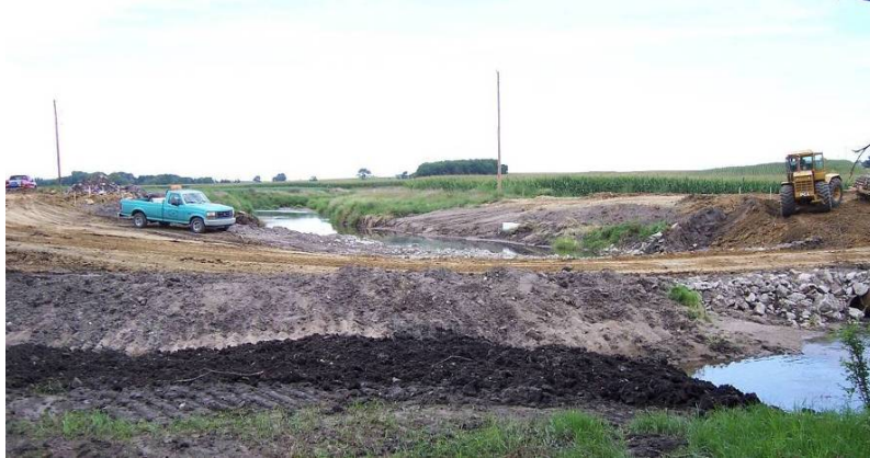
Figure 103. Cleared bridge site, August 7
