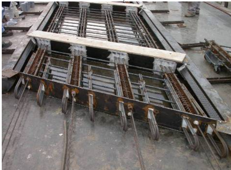
b) Double hooks and prestressing strands
