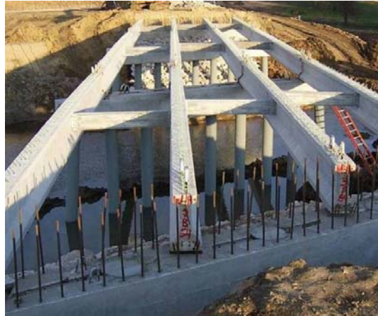
Figure 126. Erected bridge girders, October 24
