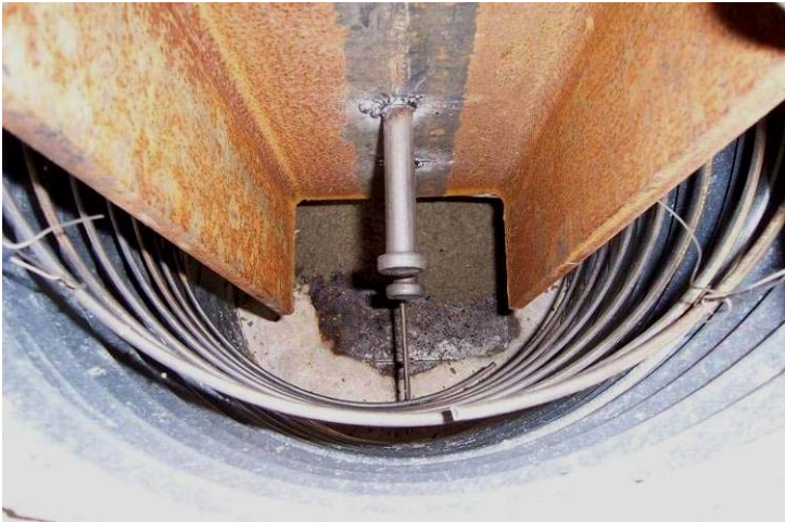
Figure 15. H-pile connection in test specimen before concrete was placed
