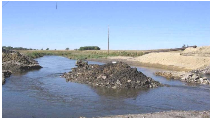
Figure 108. Bridge site on September 20
