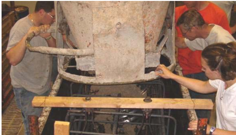
Figure 19. Concrete being placed in the first series of abutment specimen
