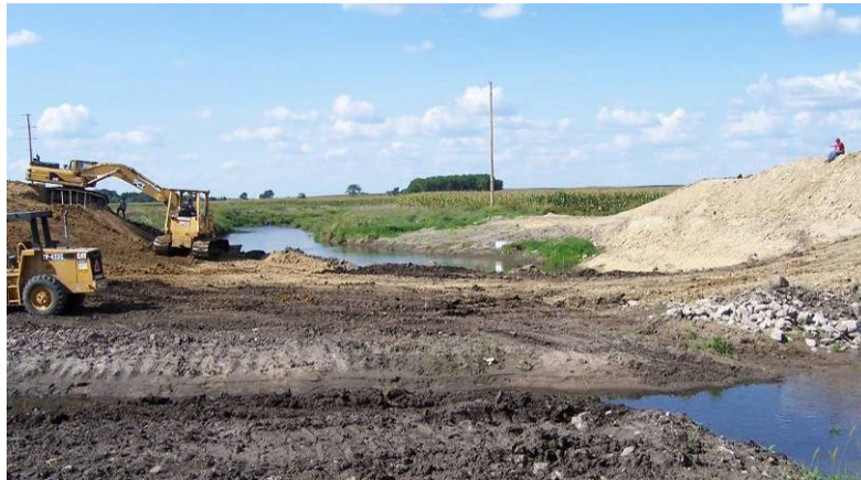
Figure 105. West bridge abutment site prepped for pile driving, September 5
