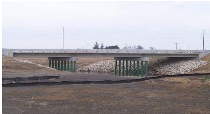
Figure 2. Completed replacement bridge on 120 th Street
