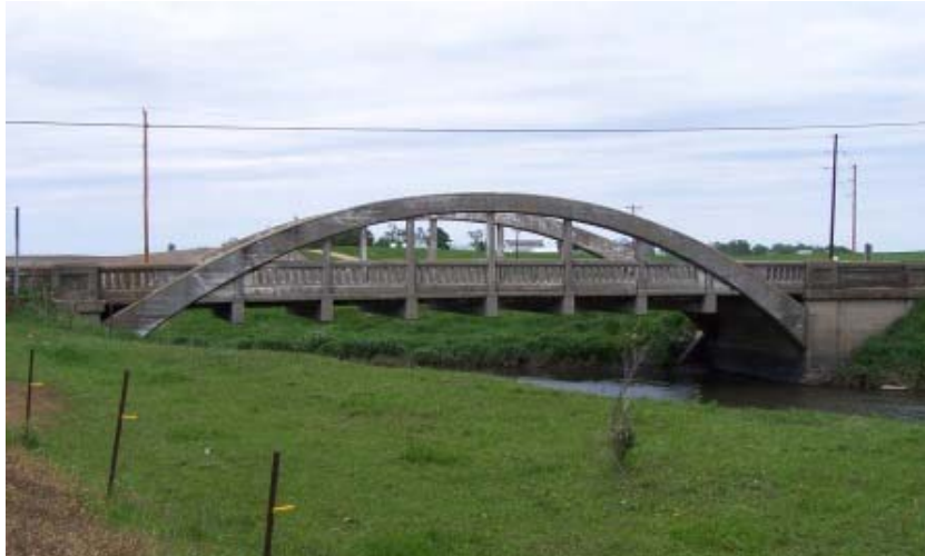
Figure 1.1 Marsh Arch Bridge originally on 120th St
