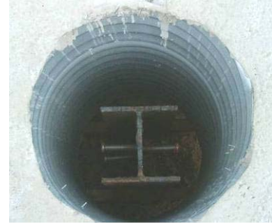
b) H-pile in the abutment
