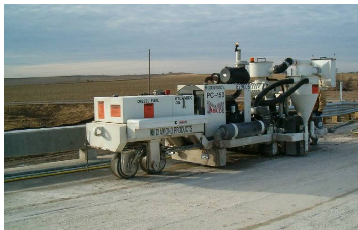
Figure 146. Bridge deck grinding equipment on site, December 27
