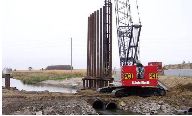
Figure 121. East pier pipe piles being driven, October 10
