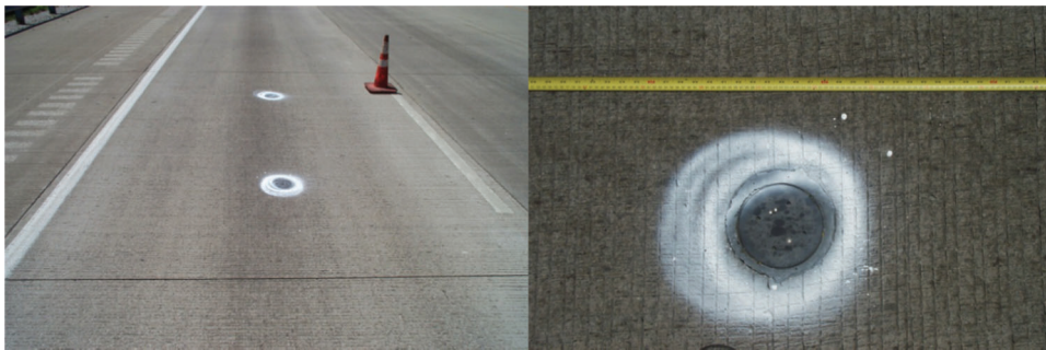
Figure 3.4 "Ground Hog" traffic count and classification sensors
