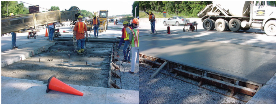
Figure 2.7 Concrete placement of the 15 inch-thick and 15-foot joint spacing slabs (south)
